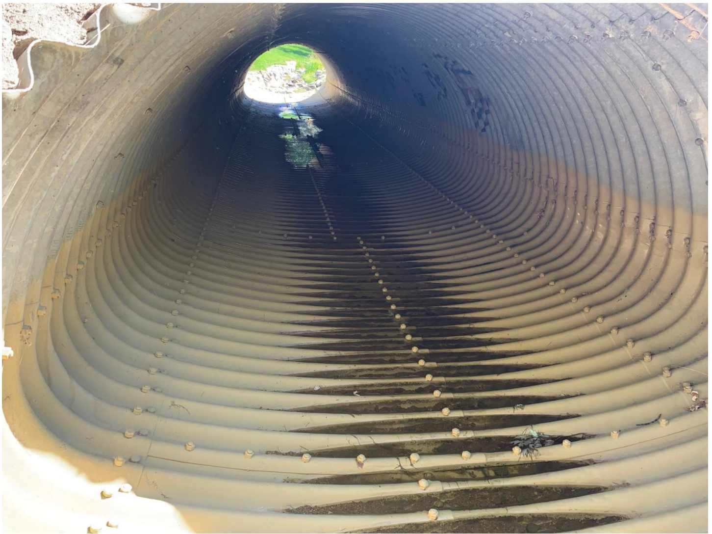
During Inspection and Cleaning Prior to lining
