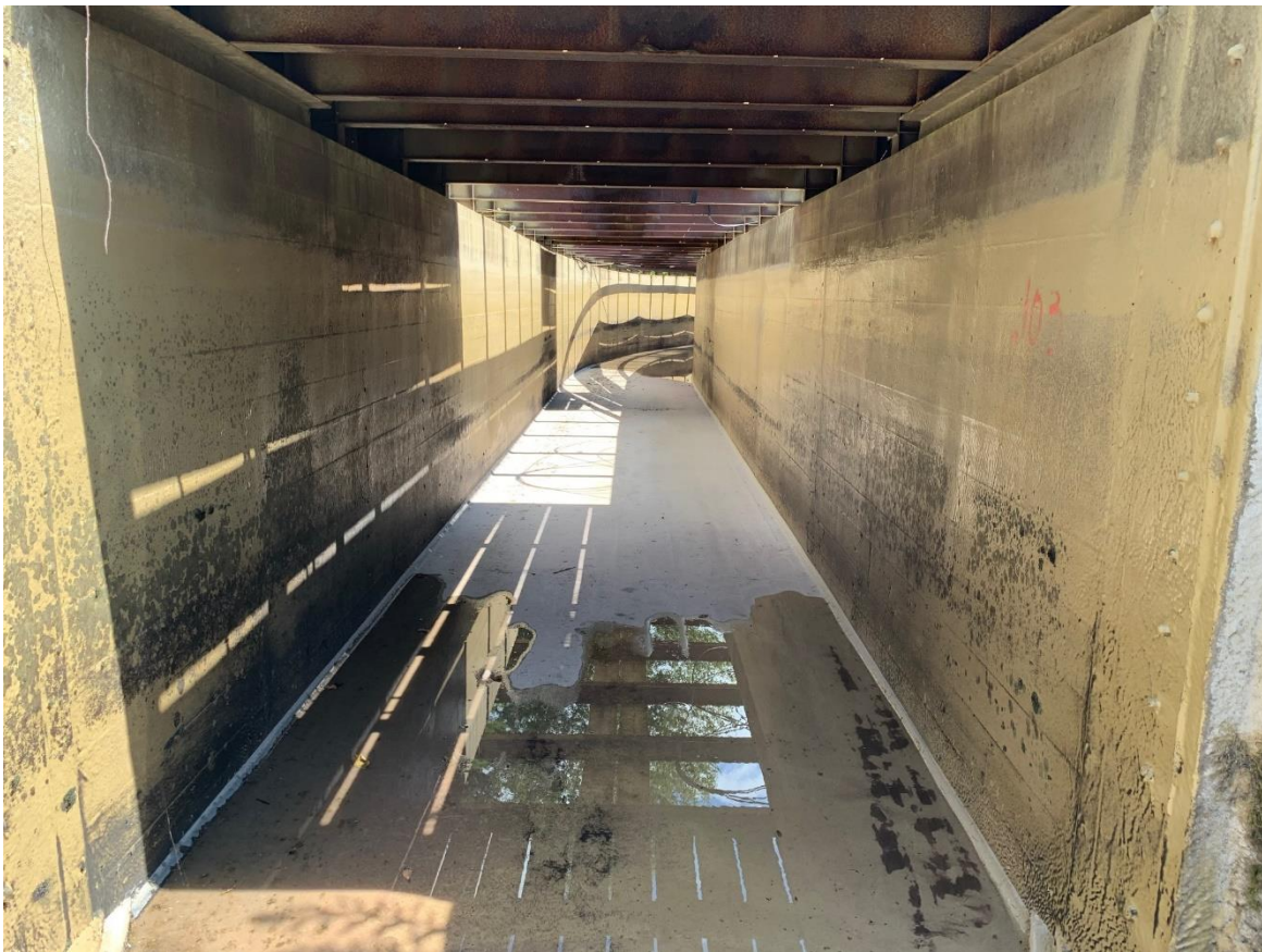
This is the Flume 12 years post liner install, not clean but in perfect condition after 24/7 operation that entire time. Note high water mark. Rock, Silt, Sand and wood travel this flume.
