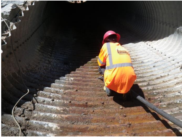
During Inspection and Cleaning Prior to lining
