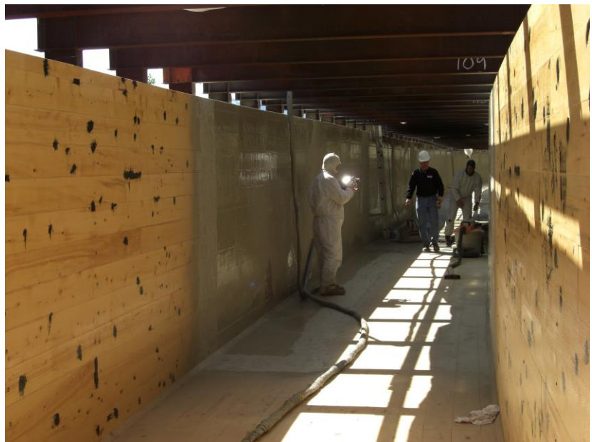
Unlined Cedar. Note that large voids were filled with a rapid dry filler and the wood was primed with a roll on primer to ensure proper bond of the 250 Mil spray applied Liner. Also note in the photo at the end of the lining material that there is an abraded surface, to ensure bond of the next layer of material. This photo was taken at the beginning of a new day of lining and is important due to some observed issues with the liner 12 years post install.
