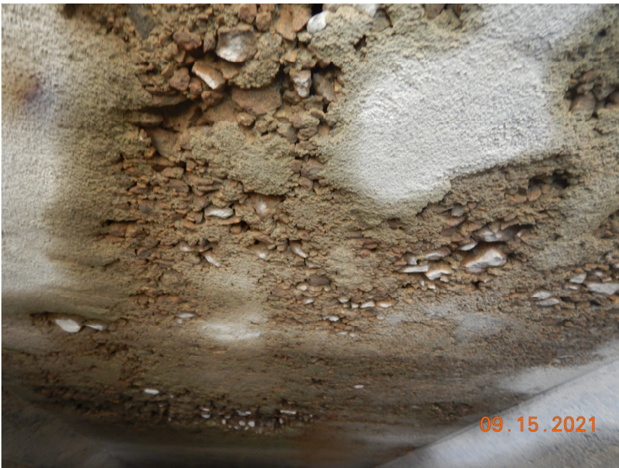
Abraded concrete with exposed aggregate on ceiling immediately downstream of the steel lining.
