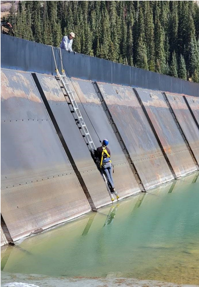
Photograph 7: View looking east from the auxiliary spillway. RJH obtains thickness measurements.
