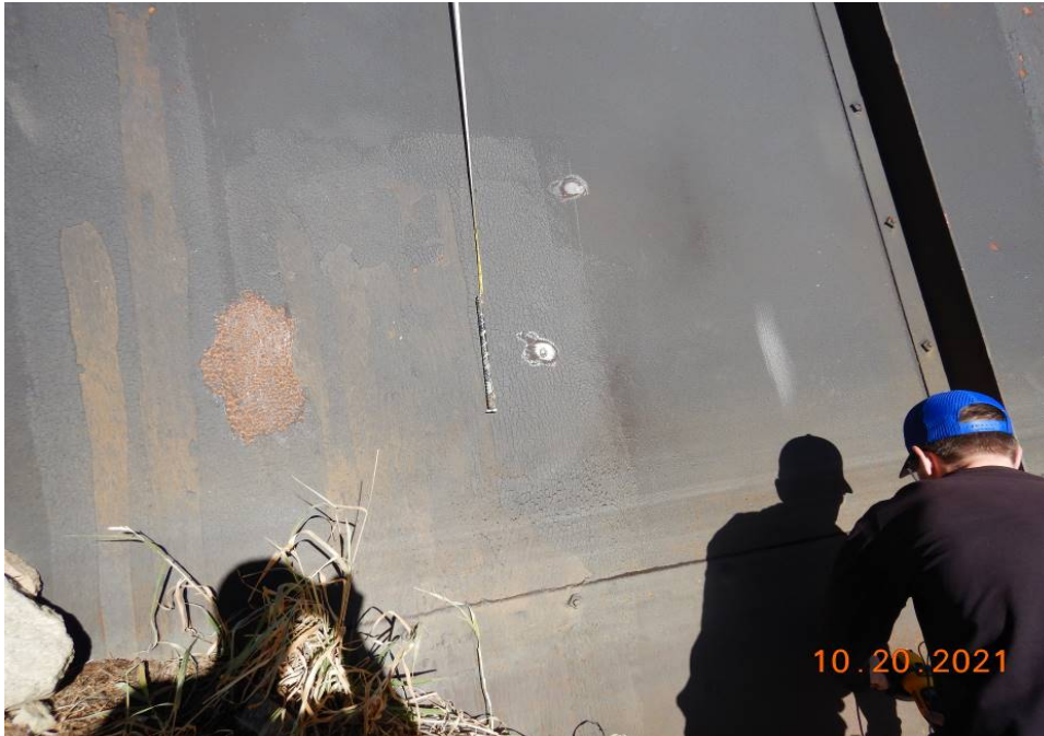
Photograph 1: View looking north at panel P01. RJH removed coating from the steel facing prior to obtaining measurements.
