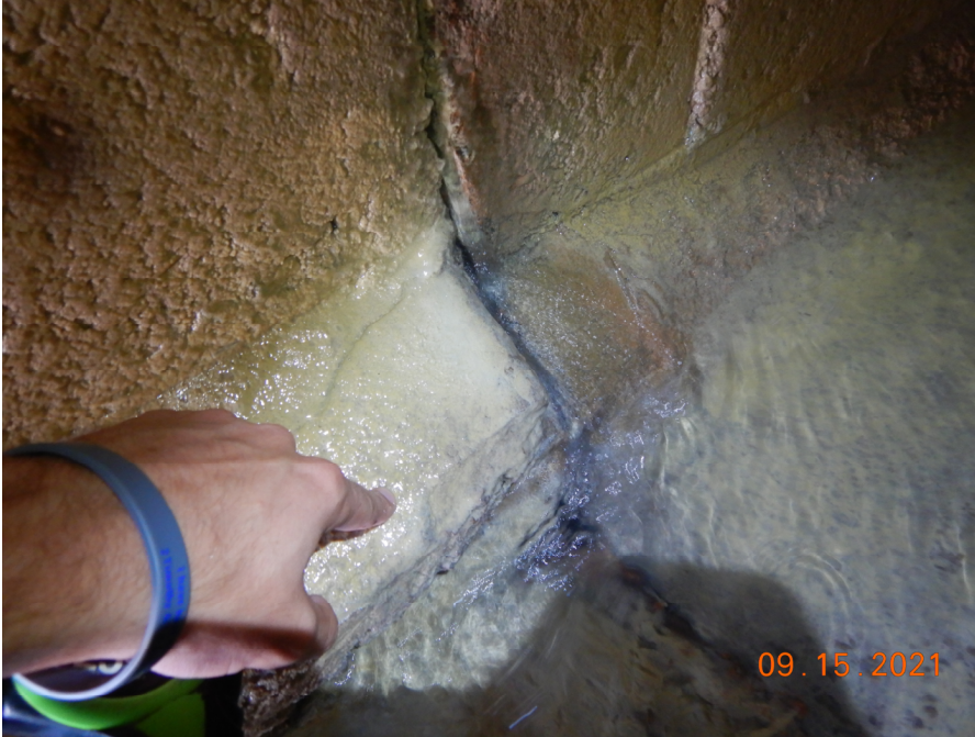
Typical joint crack with clear flow.
