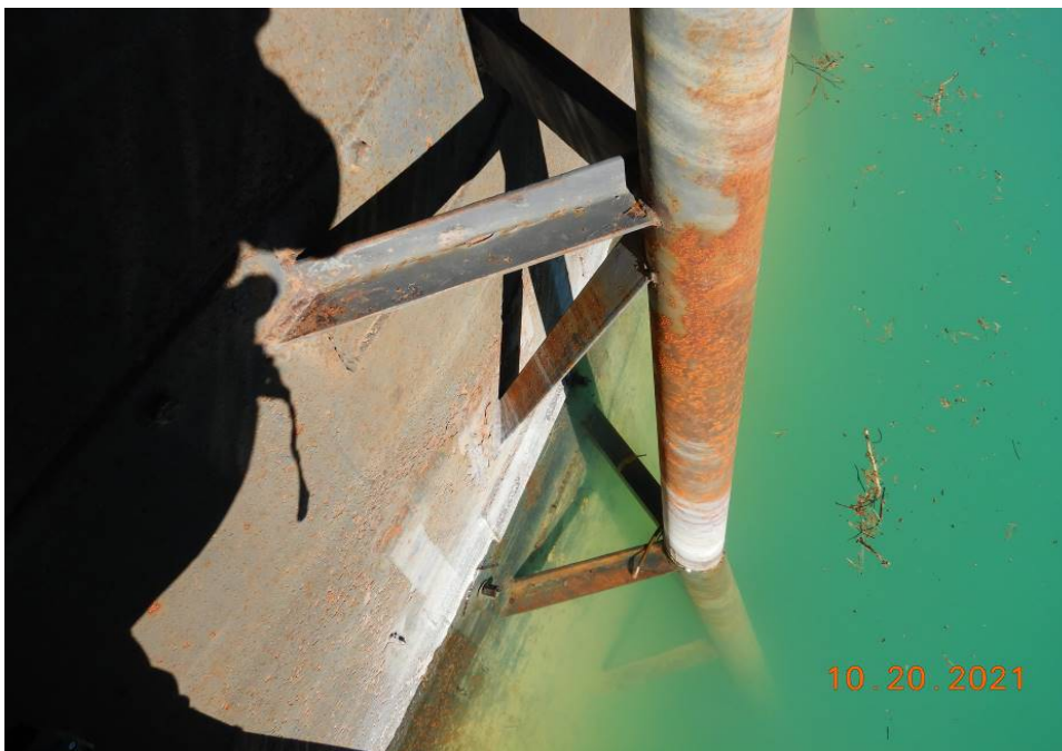
Photograph 6: Gate operator supports.
