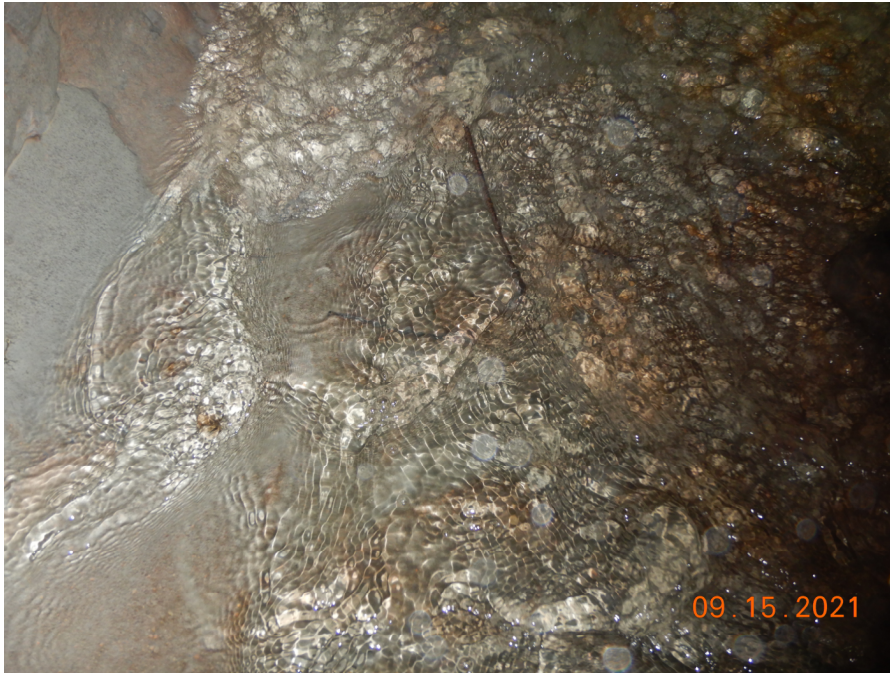
Concrete erosion of the floor immediately downstream of the steel plate lining.
