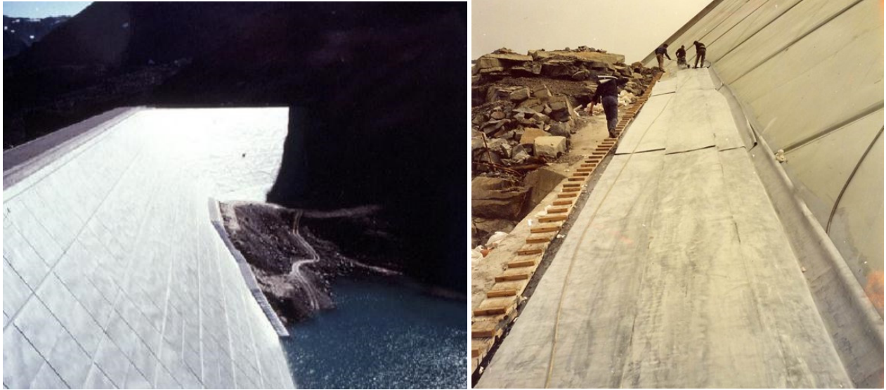
Lago Verde dam (Italy 1970) - Carpi's first installation on a dam with 38,000 ft 2 of geomembrane to connect steel facing elements to concrete plinth. On right, the installation is still in place today, more than 50 years later. This installation mirrors Grizzly Dam regarding the tricky detail of connecting a steel face to a concrete plinth.
