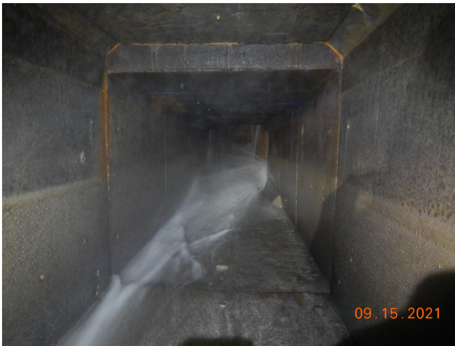
Seepage spraying from the upstream slide gate.
