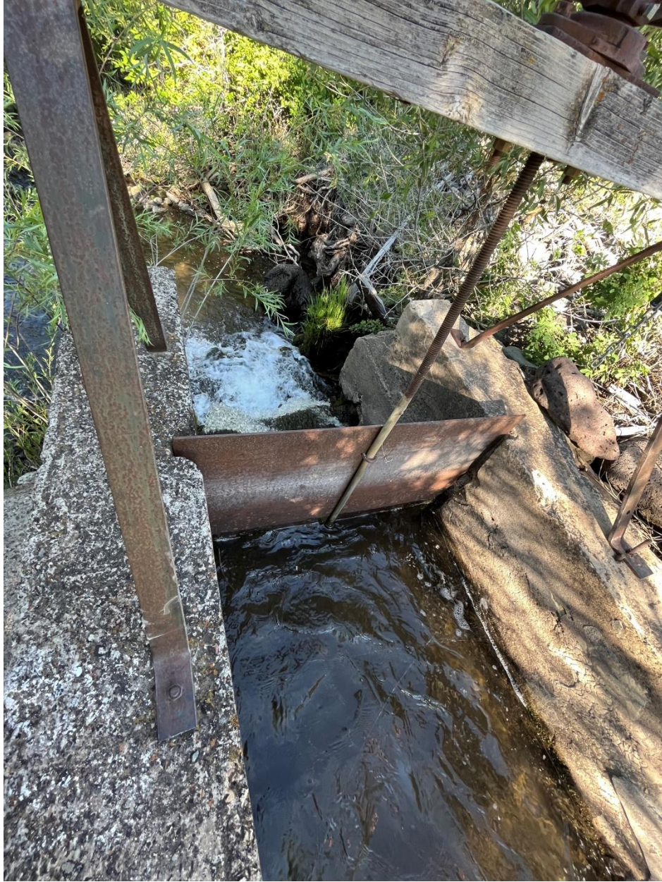
Waste Control Gate d/s of Diversion Point
