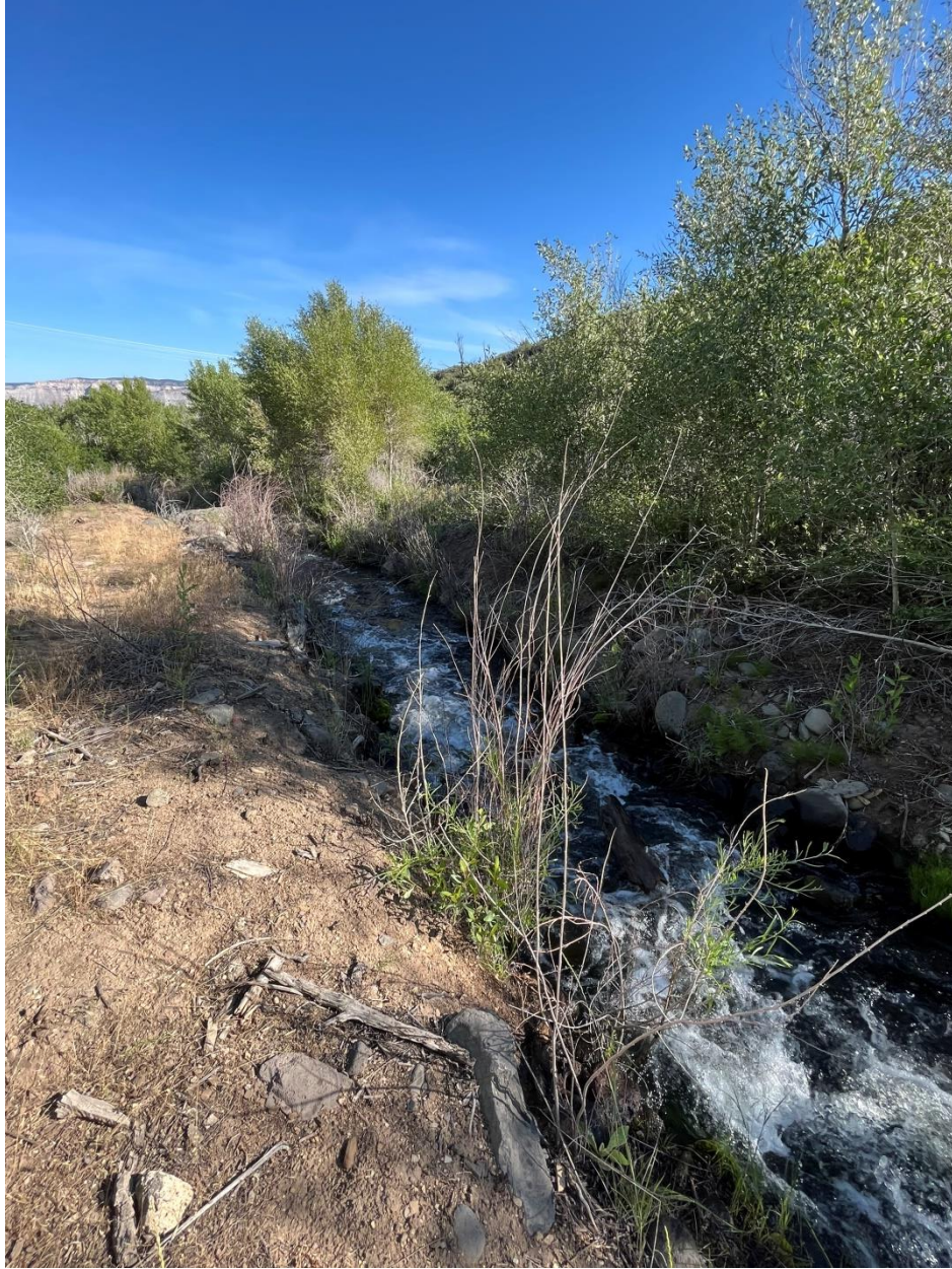
Approximate Location of Start of Buried Pipe 30' d/s of Flume
