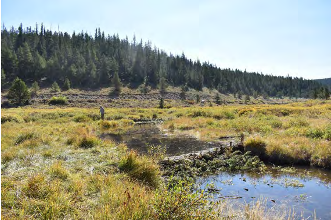
Two recently constructed BDAs along Trail Creek
