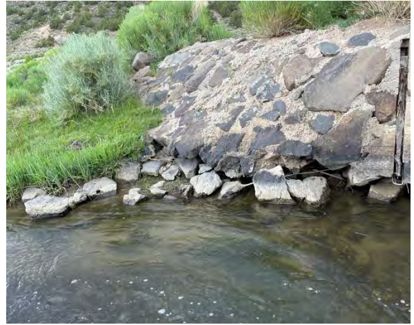
Figure 6-196 Exposed rebar on left edge of water Culebra Creek at San Luis streamflow gage.
