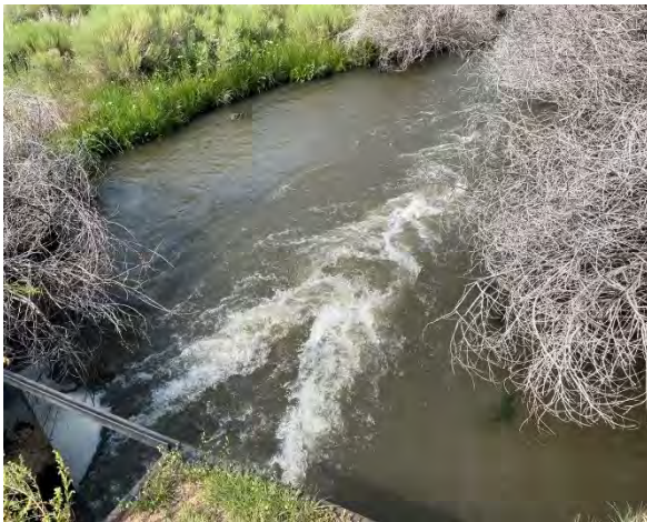
Figure 6-79 Large scour pool between splitter structure for North and South San Acacio Ditches.
