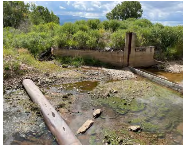
Figure 6-57 Pipe conveying San Francisco Creek through Sanchez Canal.
