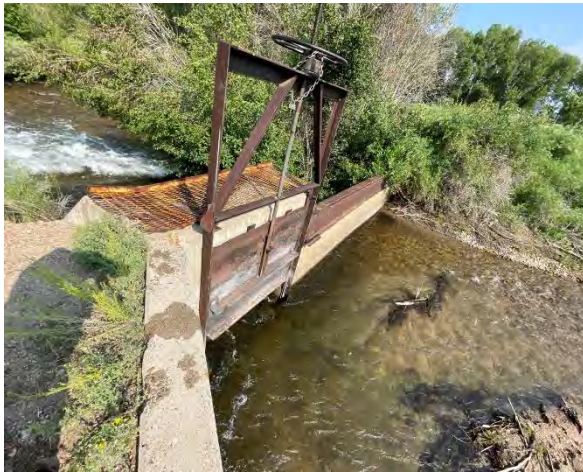
Figure 16-10 Slide gate regulating flows in Culebra Creek at Sanchez Canal Diversion Dam.
