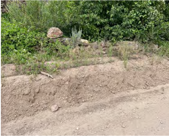
Figure 6-156 Road grading around crossing on Rito Seco creek shows the creation of berms that prevent water from running off the road as sheet flow (37.2531, -105.3336).
