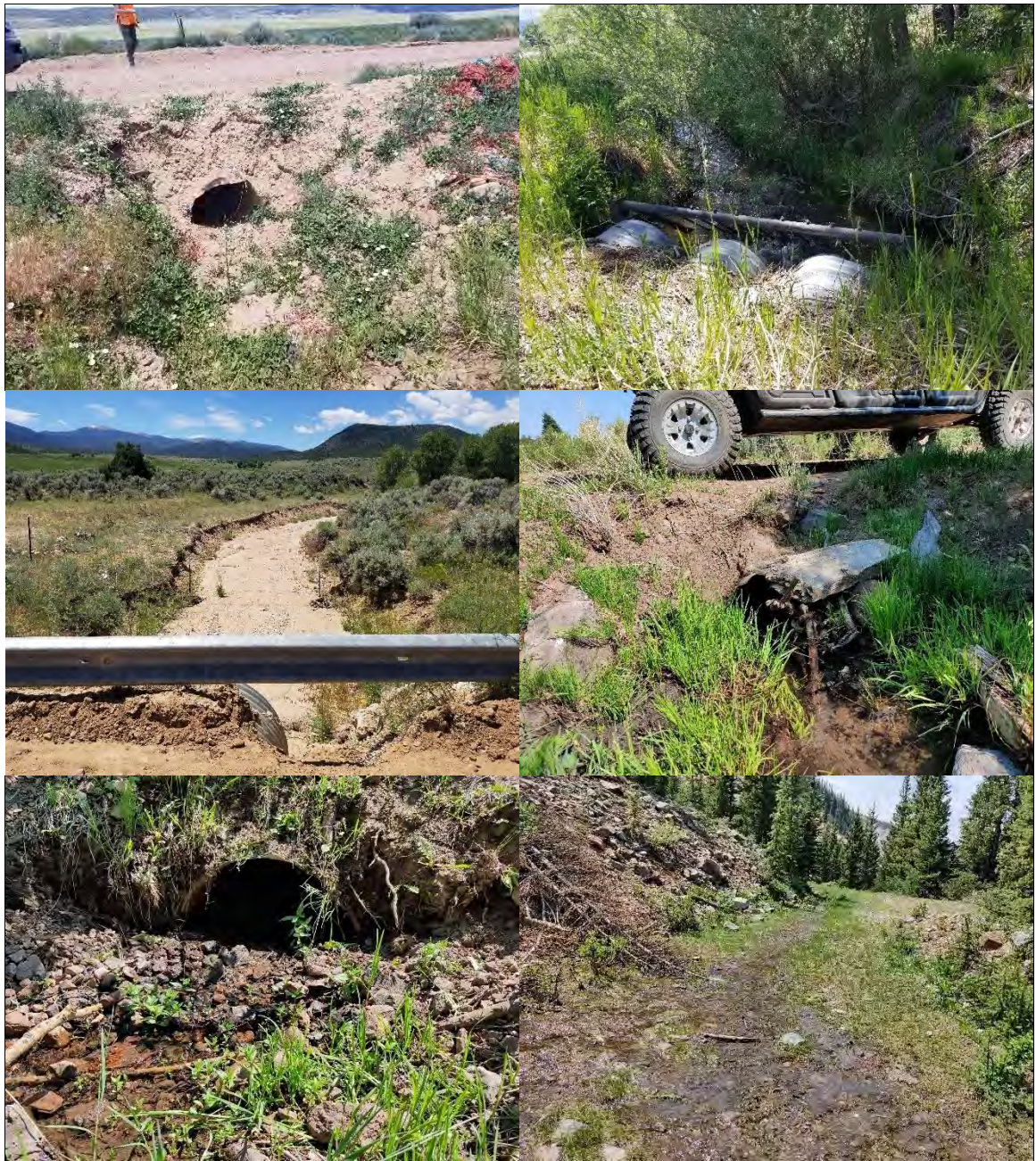
Figure 4-12 Top left: culvert filling with sediment below the road. Top right: three culverts convey water at the road crossing. Middle left: culvert at a road crossing, notice channel incision and cutbanks. Middle right: culvert at road crossing filling with sediment. Bottom left: culvert filling with sediment. Bottom right: water running off down the road.
