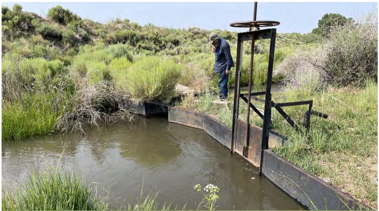
Lateral headgate San Acacio Ditch
