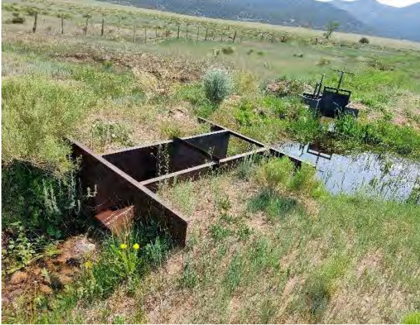
Figure 6-139 Maestas Ditch splitter boxes at County
