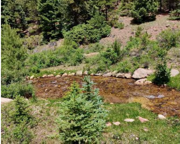
Figure 6-180 Stream channel stabilization below area of extensive hillslope erosion.
