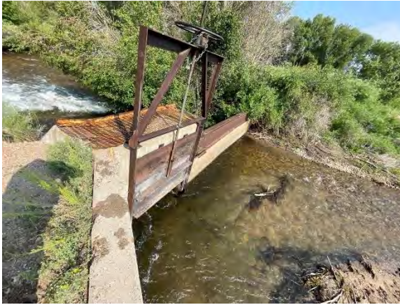
Figure 4-71 Headgate across Culebra Creek for the Sanchez Canal.
