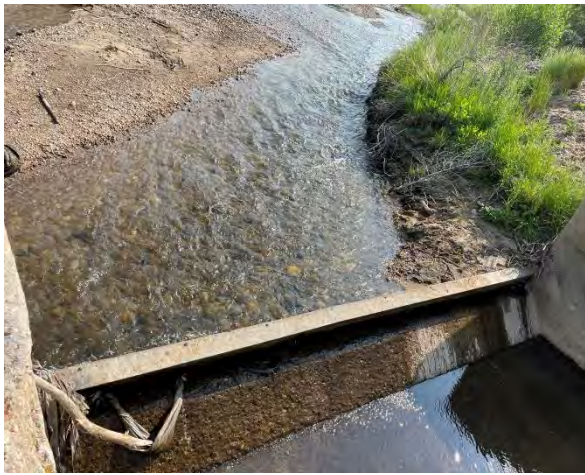
Figure 6-44 Sanchez Canal headgate, headgate seeping into canal. Culebra Creek regulated to flow through four-foot slide gate.
