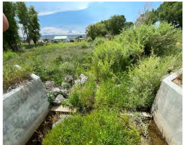
Figure 6-97 Vallejos Ditch south Parshall flume some light debris.
