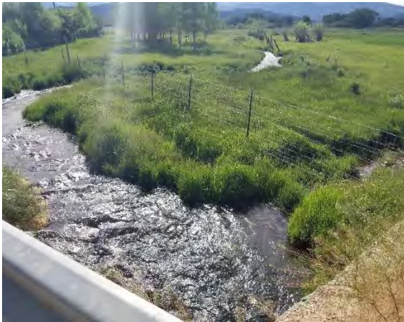
Figure 6-169 Bridge not aligned with creek.
