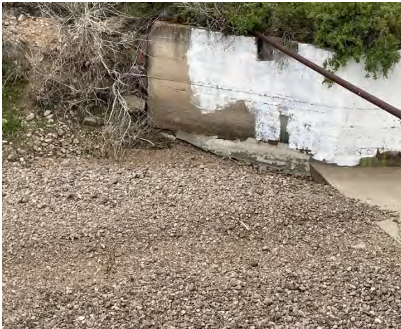
Figure 6-205 Some scour noted on upstream left edge of flume.
