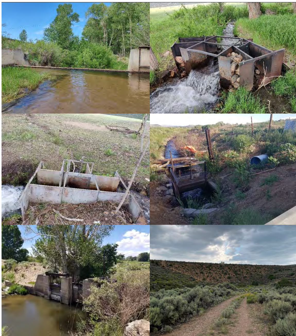
Figure 4-13 Top left: sediment filling in behind check structure at San Francisco Ditch headgate, notice elevation difference between top of the structure and downstream of it. Top right: splitter box to split flows. Middle left: splitter box. Middle right: culvert and headgate. Bottom left: headgate for Culebra Cerritos, Island Ditch, and Francisco Sanchez. Bottom right: the Sanchez Dam.
