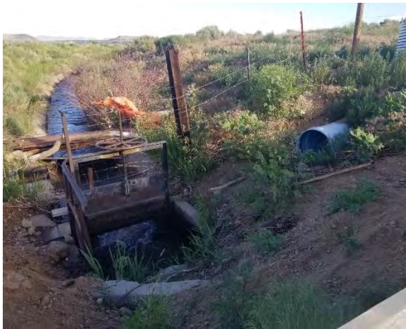
Figure 6-63 Cerro Ditch farm headgate.
