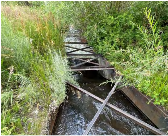
Figure 6-96 North Parshall flume was found with good drop and was clean in good condition.
