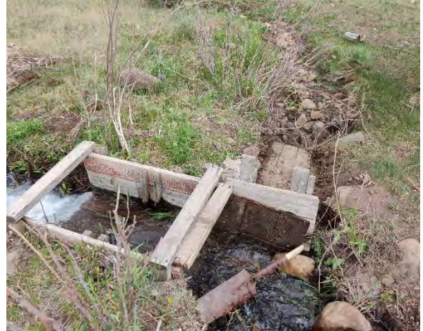
Figure 6-137 Wood splitter box on Cuates Creek.
