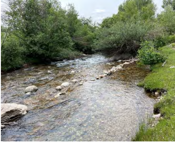
Figure 6-8 Hand built cobble diversion dam. No risk of flooding, ditch may trap fish.
