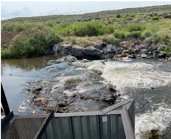
Figure 6-77 San Acacio diversion dam, with trash.
