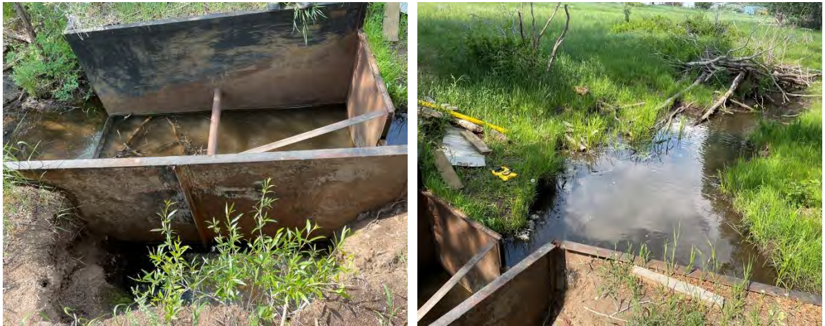
Figure 6-134 Jaroso Ranch ditch splitter structure with erosion on left edge.
