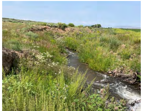
Figure 6-80 Erosion along San Acacio ditch.
