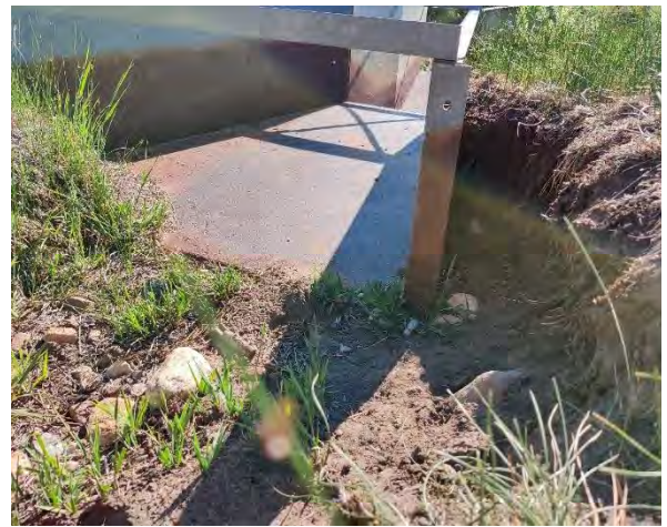
Figure 6-25 Measurement flume with debris in inlet and scour downstream. Scour noted on left edge of flume.
