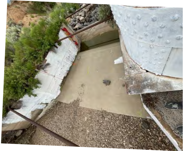
Figure 6-204 Flume clean and relatively free of debris. Staff plate has been vandalized.
