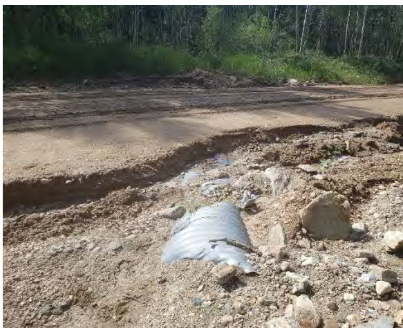
Figure 6-163 Two plugged culverts and roadway erosion on Forbes Road.
