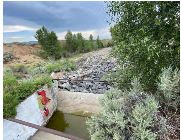
Figure 6-206 Downstream riprap placed to prevent erosion.
