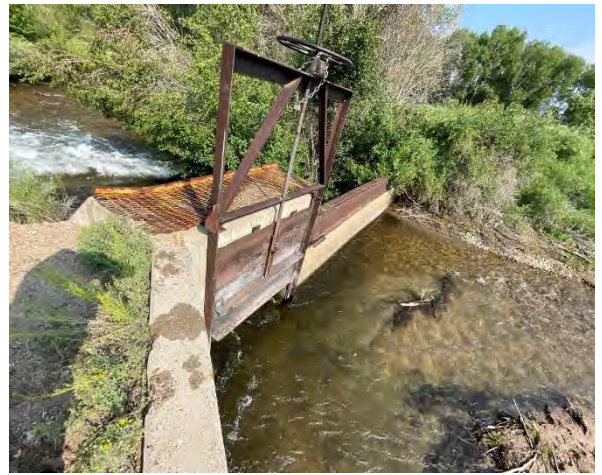
Figure 6-44 Sanchez Canal headgate, headgate seeping into canal. Culebra Creek regulated to flow through four-foot slide gate.
