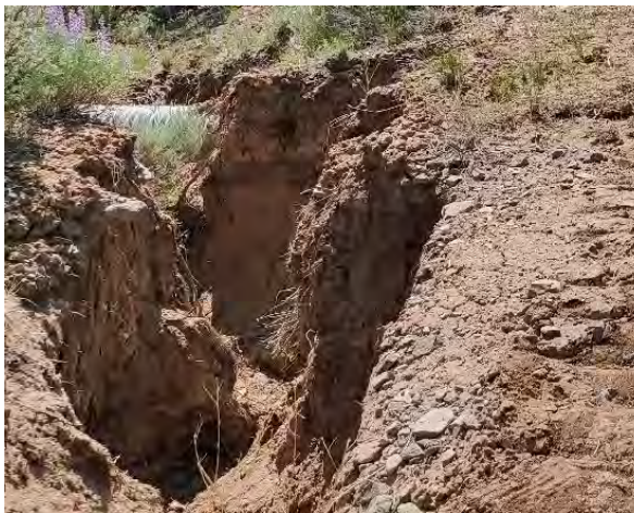
Figure 6-185 Headcut up road ditch near culvert.
