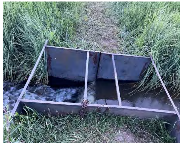
Figure 6-6 Montez Ditch headgate, metal splitter box with no observed measurement structure.
