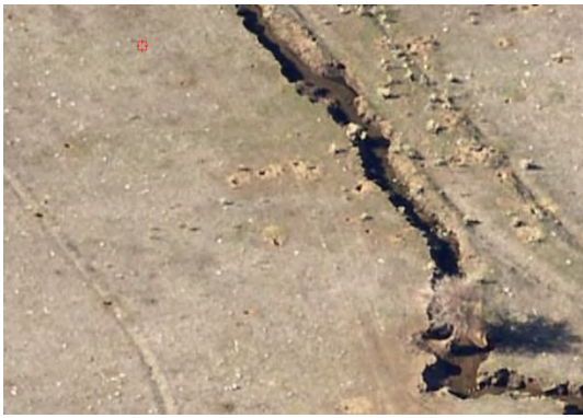
Figure 6-28 Jose M Sanchez Ditch showing significant erosion throughout portions of the ditch.
