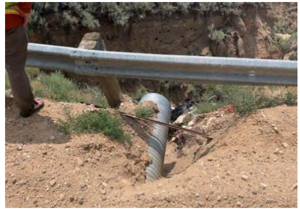
Figure 16-7 Roadway safety hazard due to embankment failure and insufficient culvert cover along County Road K.5.
