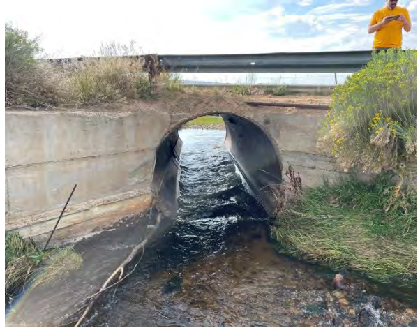
Figure 6-168 Culebra Creek County Road L.5 bridge. This bridge is not aligned with the creek. Some seepage noted on left edge.
