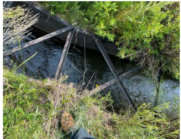
Figure 6-75 Francisco Sanchez measurement flume, submerged - inoperable.
