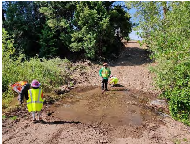
Figure 6-182 Low water crossing that is not stabilized by streambed.
