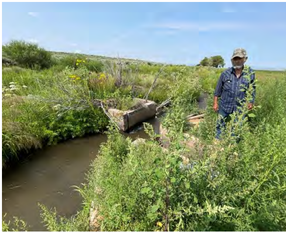
Figure 6-81 Farm headgate from San Acacio Ditch. Estimates indicate that many of these structures may date back to the 1920s.
