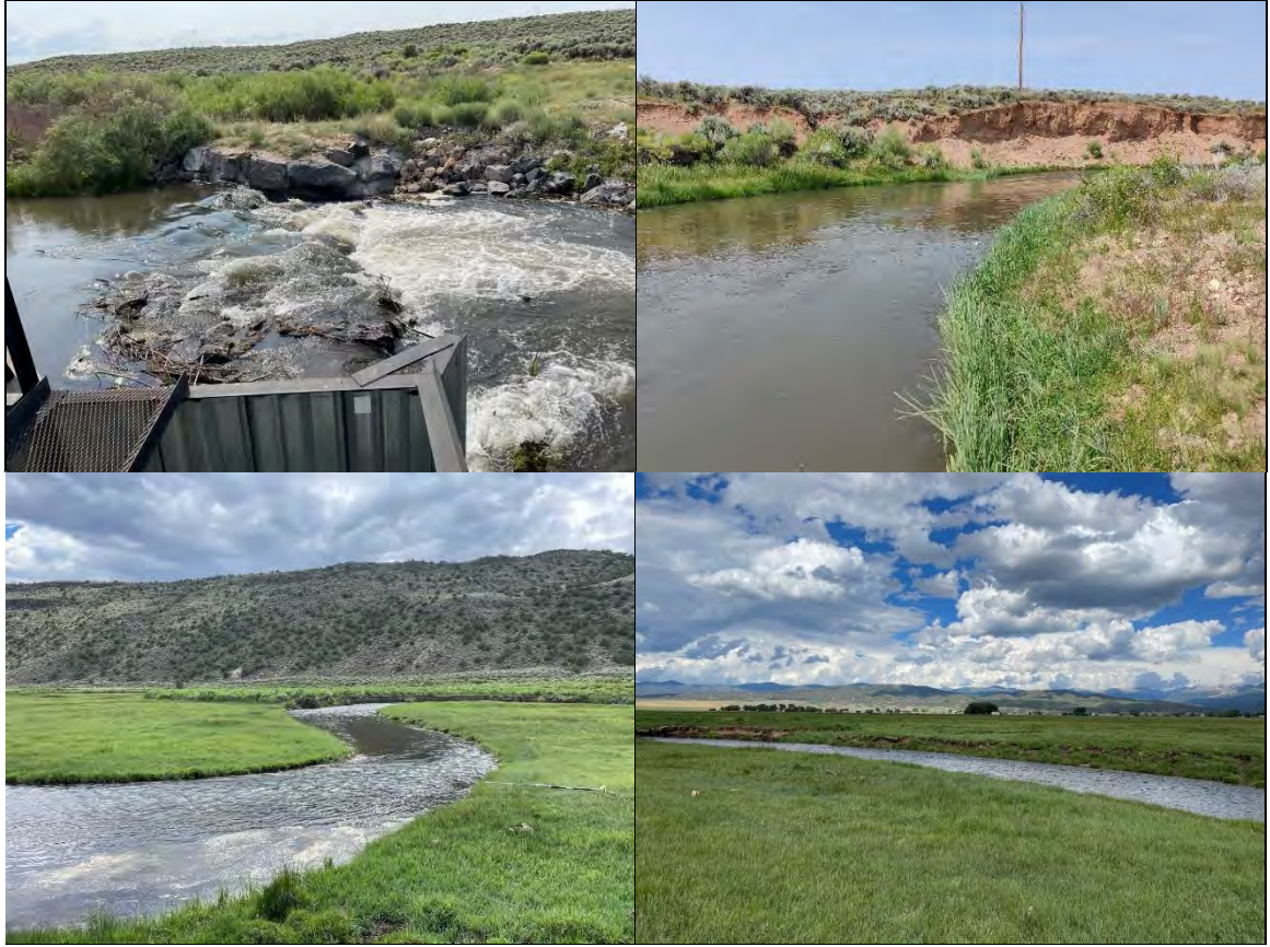
Figure 4-16 Top Left Culebra Creek (30) notice use of riprap for bank stabilization. Top Right Culebra Creek (29) notice bank erosion in background. Bottom Left Culebra Creek (27) notice vertical bank in the background. Bottom Right Culebra Creek (27) notice channel is slightly entrenched with bank erosion.
