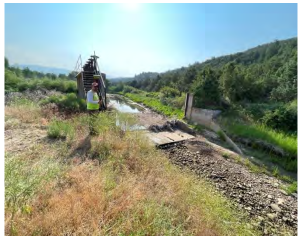
Figure 6-47 Flood gates on Sanchez Canal near Culebra Creek headgate. Concrete apron once had places to insert boards to stop flow down ditch.
