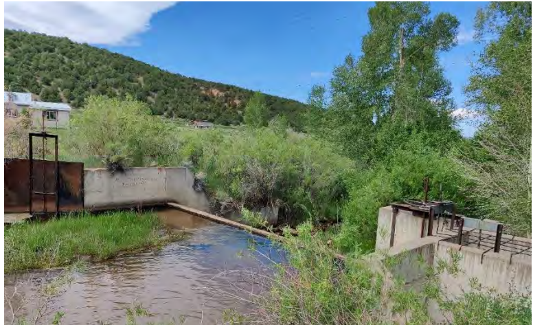
Figure 16-23 San Francisco Ditch diversion dam. Single screw gate on left edge of water provides sediment passage when ditch is not in priority.
