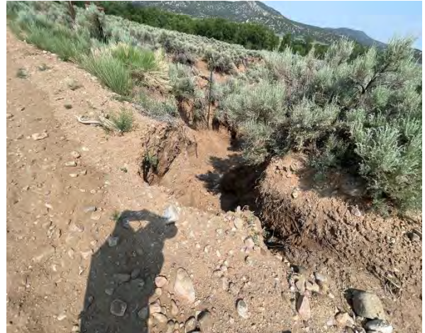
Figure 6-157 County Road M.5, water concentrated from road is the probable cause of gully erosion.
