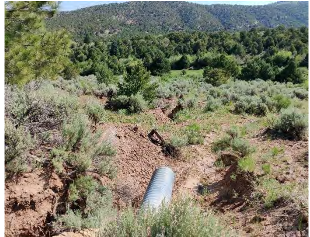
Figure 6-171 Culvert outlet causing downstream erosion due to large drop below outlet.
