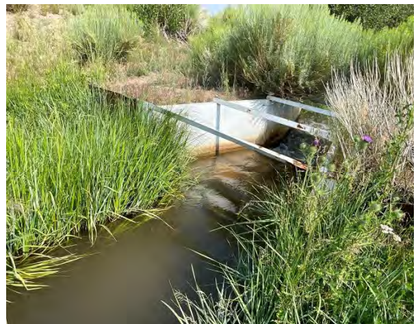
Figure 6-76 Culebra Cerritos Canal and Island Ditch 6-ft measurement flume.
