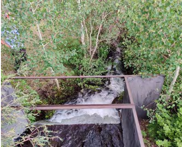
Figure 6-136 Large drop below splitter box on Cuates Creek diversions, preventing fish passage and increasing risk of structure failure.
