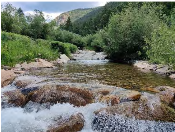
Figure 4-87 El Poso Creek upstream of ElPoso202107091115, notice drop structures and boulder bank protection.
