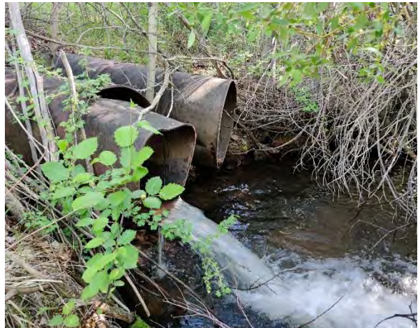
Figure 6-170 Culverts causing degradation in the stream and reducing fish passage on Torcido Creek.
