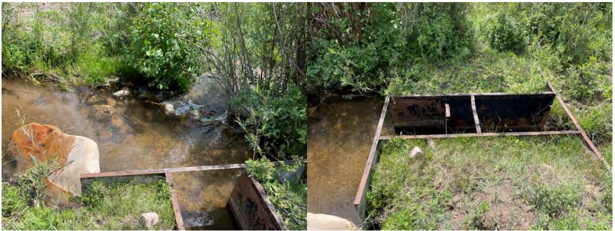
Figure 6-86 Bennie & Kiko headgate. Appears to be functioning with some gate leakage.
