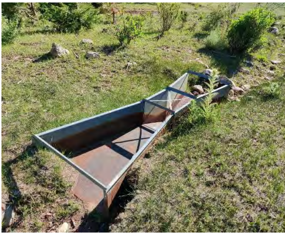
Figure 6-24 Measurement flume Canon Ditch No. 1.
