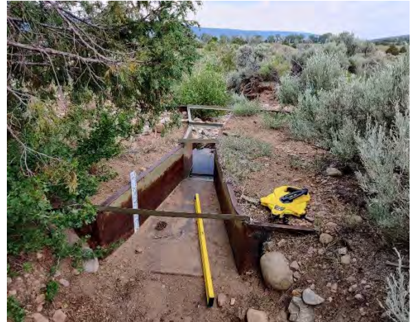
Figure 6-143 W.F. Meyer measurement flume. Downcutting noted in channel below structure.
