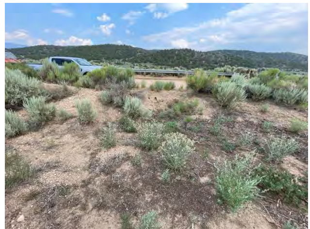
Figure 16-3 No culvert found in drainage, guardrail along roadway downstream due to gully formation (headcut).
