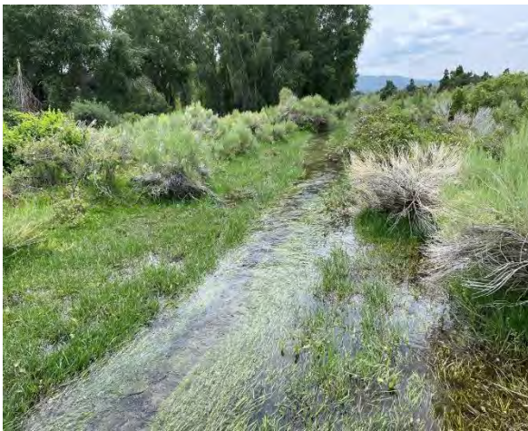
Figure 6-10 Water diverted into ditch was greater than ditch capacity resulting in overland flow back to creek.
