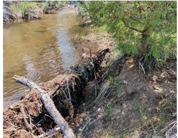
Figure 6-210 Flow along left edge of water of Willow Creek fish barrier.
