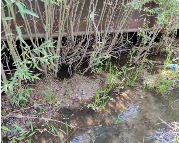
Figure 6-167 Jaroso Creek at County Road 21 bridge partially blocked by sediments and willows.
