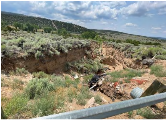
Figure 16-6 Vallejos tributary gully erosion and trash dumping along County Road K.5. Note culvert in lower left of photo extending well above the channel invert.
