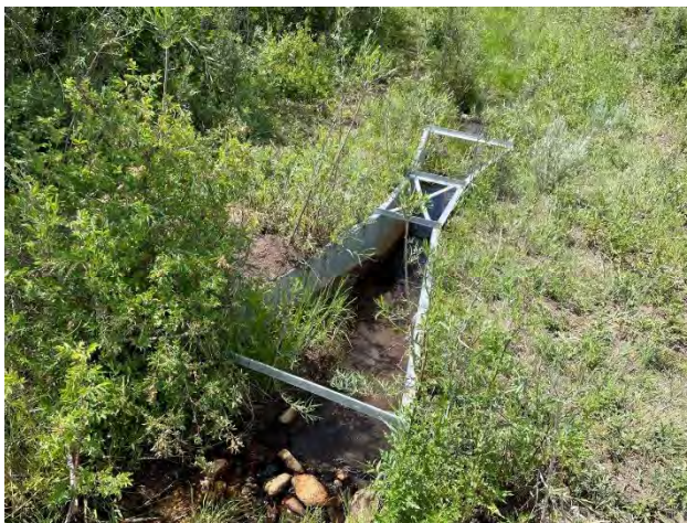
Figure 6-87 Bennie & Kiko 1 ft Parshall Flume with significant debris in structure including grass and rocks.
