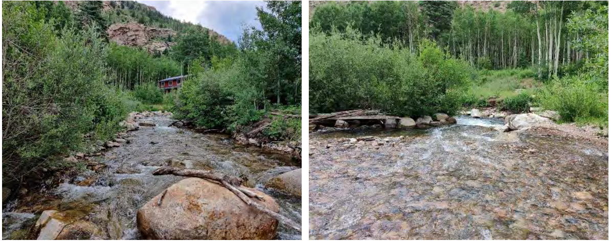
Figure 6-193 Boulder toe stabilizing channel around houses along El Poso Creek (left) and channel stabilization work resulting in a large drop in a channel that is causing excessive erosion downstream and high probability of head cut upstream after toe failure in a channel (right).
