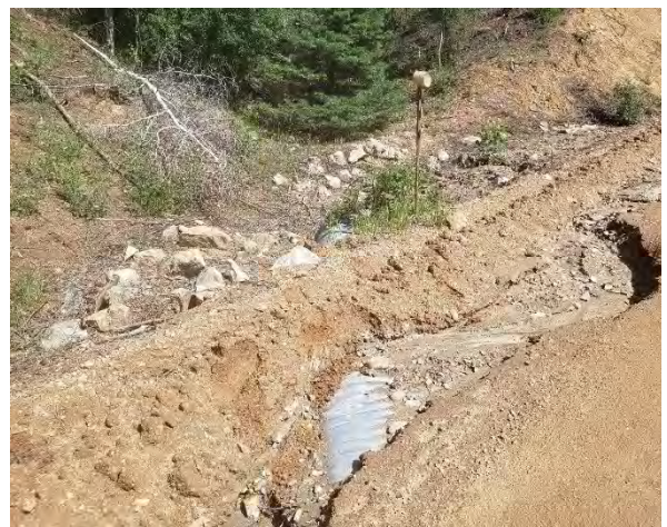
Figure 6-163 Two plugged culverts and roadway erosion on Forbes Road.
