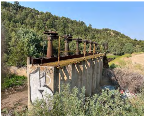
Figure 6-47 Flood gates on Sanchez Canal near Culebra Creek headgate. Concrete apron once had places to insert boards to stop flow down ditch.
