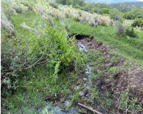
Figure 6-12 Erosion from ditch seepage.
