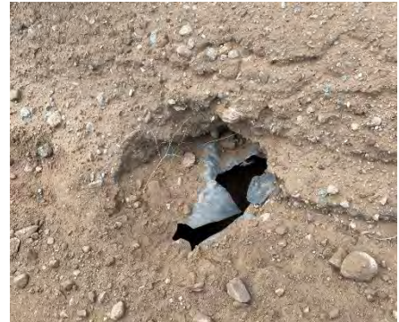
Figure 16-2 Damaged culvert in Rito Seco Road.
