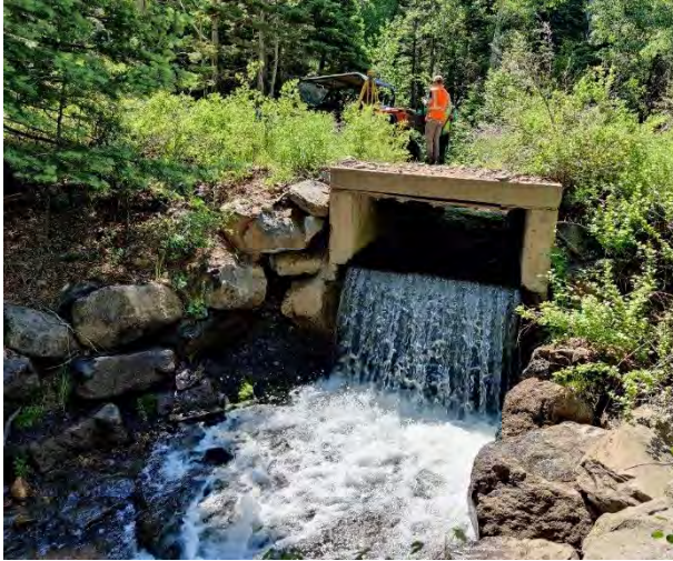
Figure 6-207 Jaroso Creek fish barrier.
