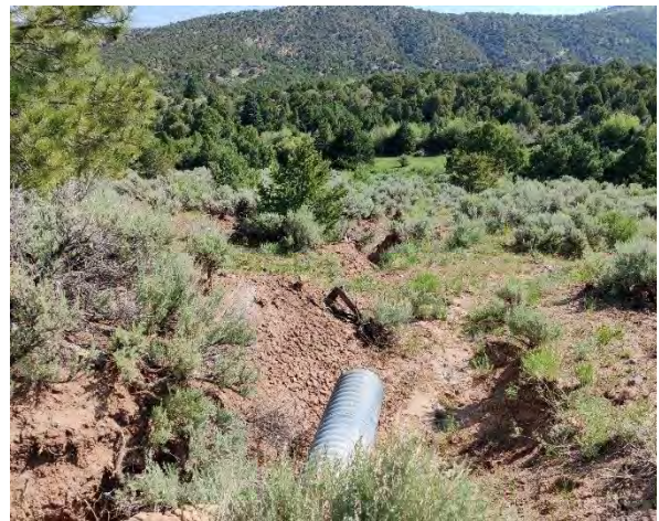
Figure 6-186 Downstream end of culvert that is buried upstream in Jaroso Creek drainage, headcut along road embankment shown in Figure 6-185..
