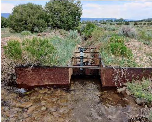
Figure 6-142 W.F. Meyer diversion structure from Willow Creek.
