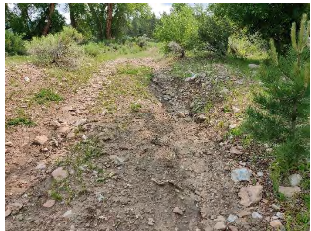
Figure 16-29 Ruts in road from water running down road instead of in channel.
