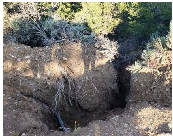
Figure 6-158 Skidmore Road head cut, Note concentrated flow down road (lower left) culvert remnant (lower right).
