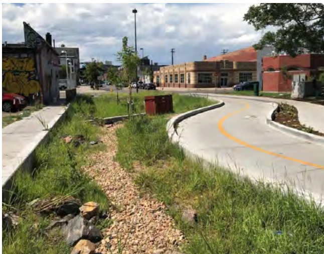
This bioretention water quality facility located at 21st and Broadway in downtown Denver removes pollutants from stormwater runoff before releasing the water to the storm sewer.
