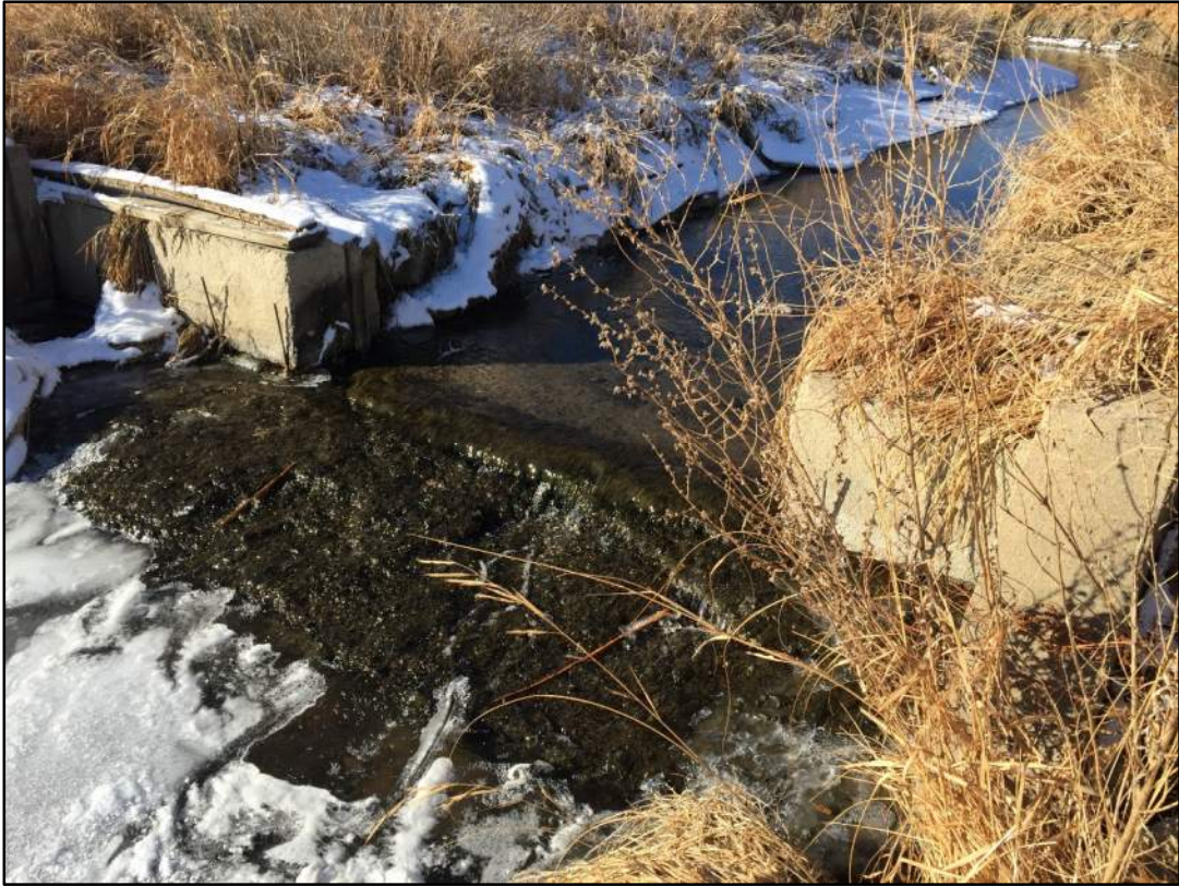
Photo 3: Smith and Emmons Ditch Check Structure
