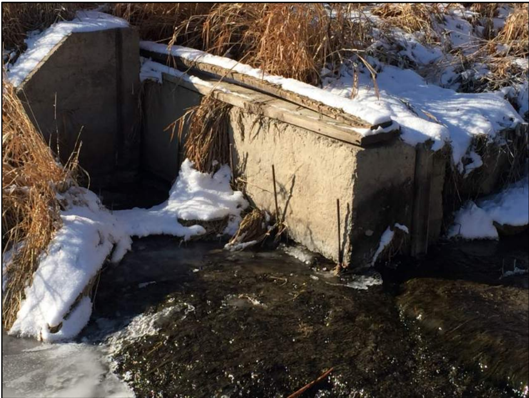
Photo 4: Smith and Emmons Ditch Check Structure - Detail
