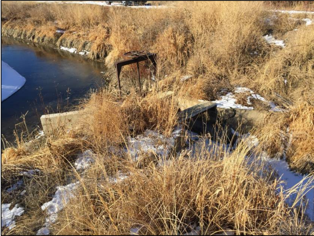
Photo 1: Smith and Emmons Ditch Headgate
