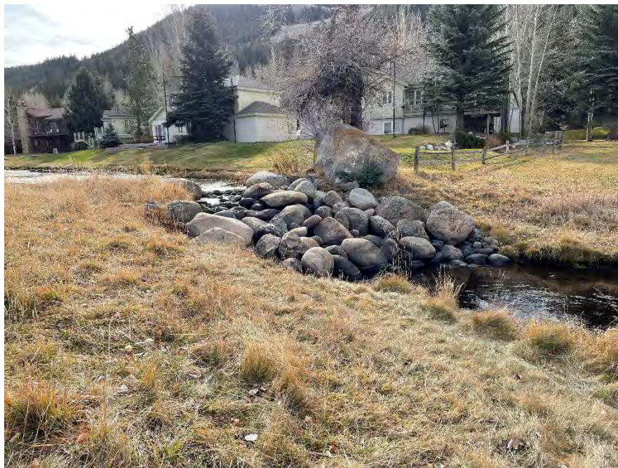
Nine Man-made boulder dams – causing sediment aggradation, bank erosion, poor water quality, and that are fish barriers.
