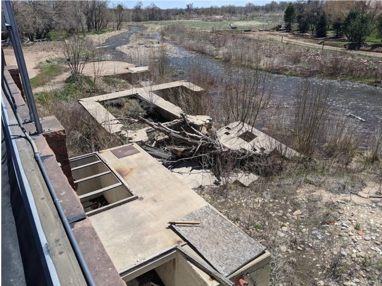
Figure 2 Downstream design area from the middle of the site
