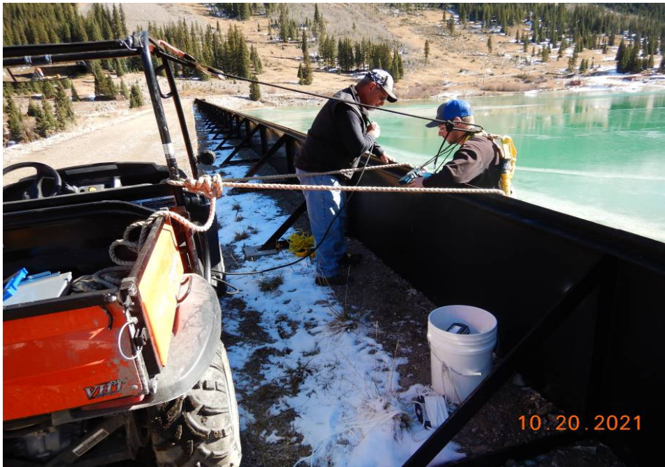
Photograph 2: View looking east near Station 0+15. RJH accessed the steel facing with a ladder and personal fall arrest system with a lifeline. The ladder and lifeline were anchored separately to the roll cage of a side-by-side.
