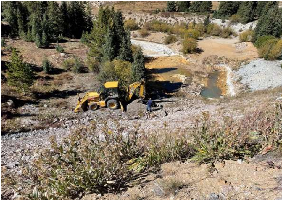
Photograph 3: View looking north from the dam crest. Excavation of TP-102.
