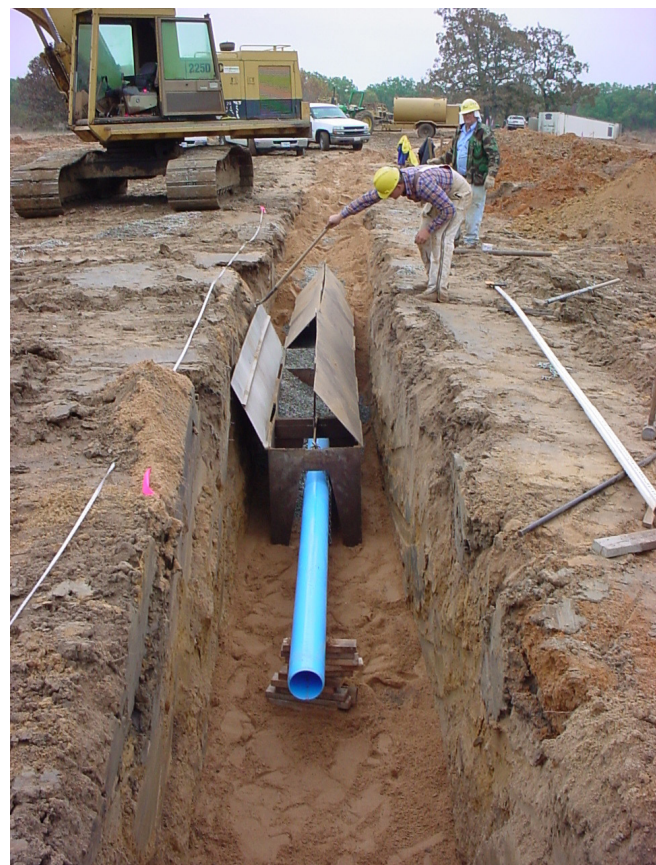
Figure 26A-3 Double filter surrounding collector pipe
