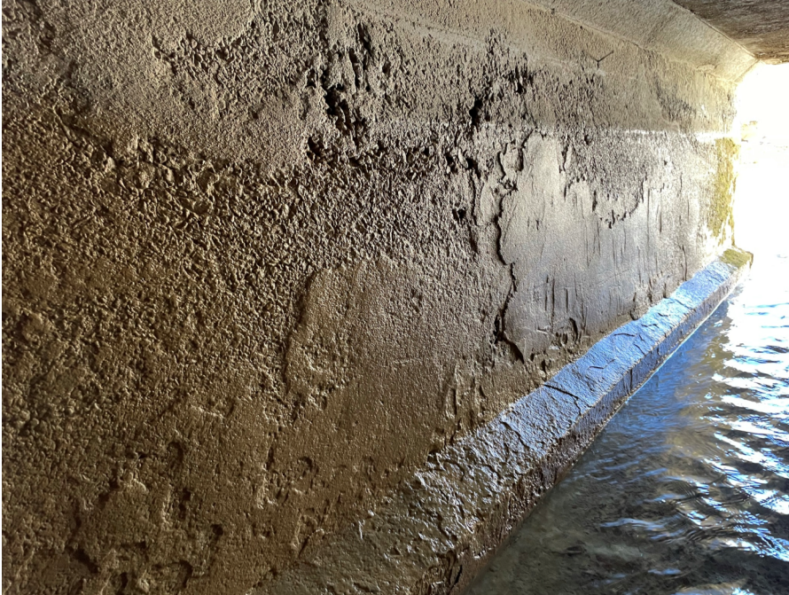
Previous concrete repairs to the first section immediately upstream of the discharge structure.
