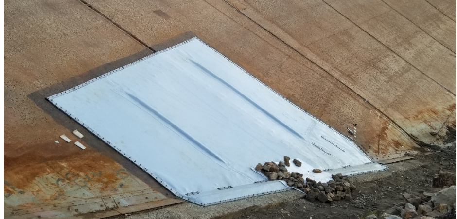
El Vado Dam (New Mexico 2018) – On the left is the test panel installation showing stainless steel tensioning profiles welded with tabs prior to the geomembrane installation. The right picture shows the completed installation. This is what the face of Grizzly will look like after we finish.
