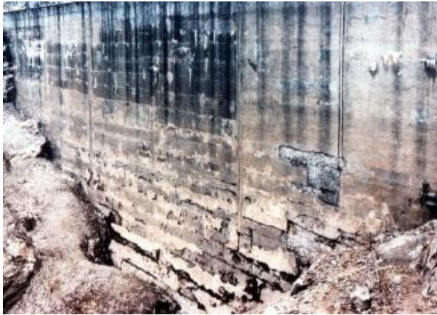
Lago Nero dam (Italy, 1980) - The pictures show the concrete gravity dam before and after rehabilitation with the CARPI system. The dam is located very high in the Alps with severe weather and has been operating for more than 40 years with the CARPI system.
