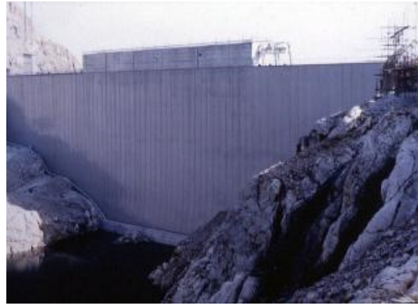
Lago Nero dam (Italy, 1980) - The pictures show the concrete gravity dam before and after rehabilitation with the CARPI system. The dam is located very high in the Alps with severe weather and has been operating for more than 40 years with the CARPI system.
