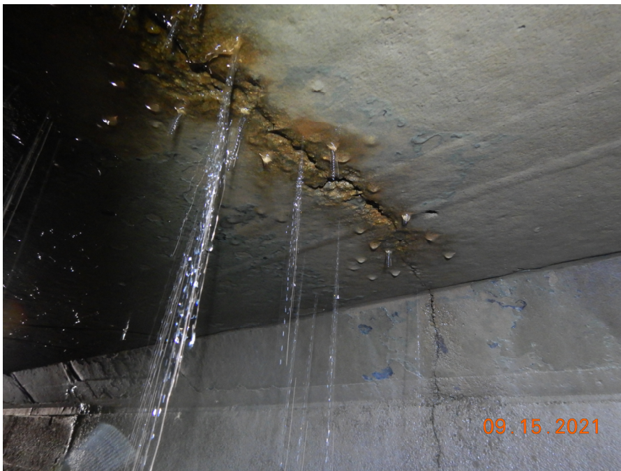
Flow from a joint crack on the outlet tunnel conduit ceiling.
