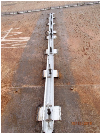
El Vado Dam (New Mexico 2018) – On the left is the test panel installation showing stainless steel tensioning profiles welded with tabs prior to the geomembrane installation. The right picture shows the completed installation. This is what the face of Grizzly will look like after we finish.
