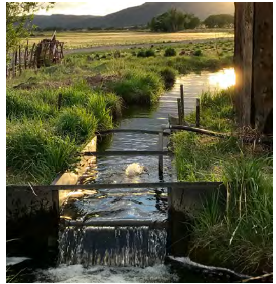
Irrigation ditch measurement structure (photo by Rio de la Vista)
