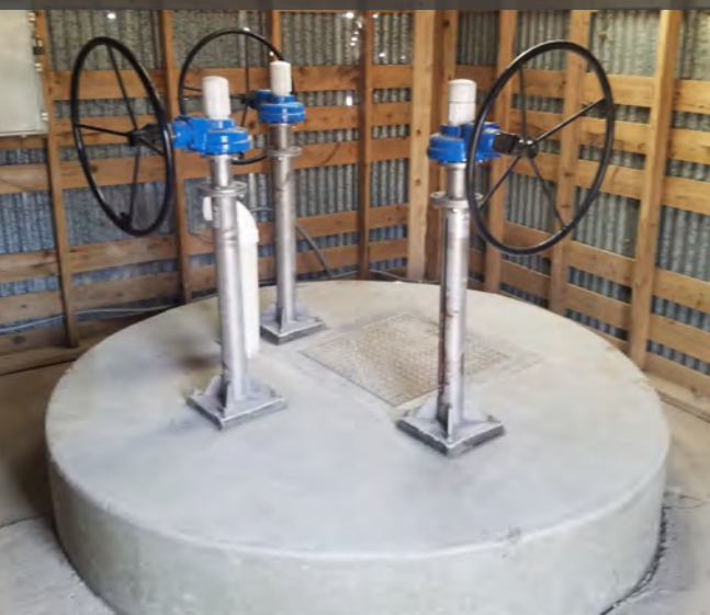
New reservoir outlet works for the Mountain Home Reservoir dam (photo by Wayne Schwab)
