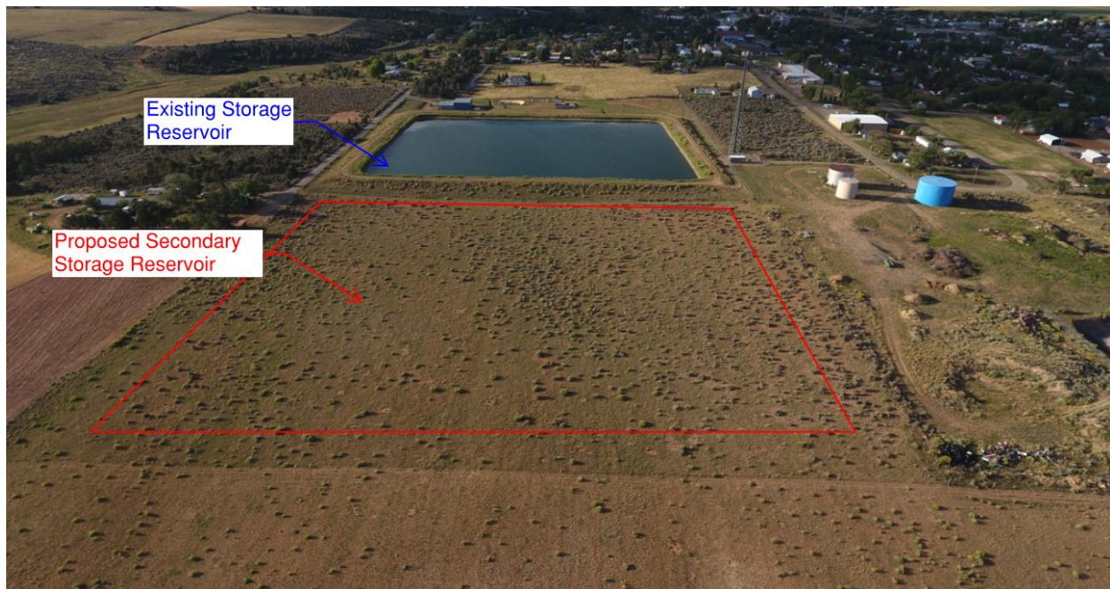
Figure 3. Drone Photo of Existing Reservoir Showing Proposed Area of Secondary Reservoir
