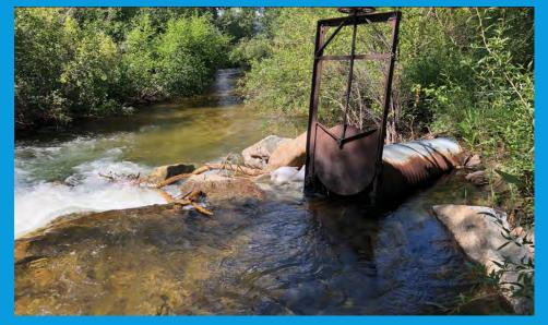
Wing wall failing causing a drop in water level at the headgate.
