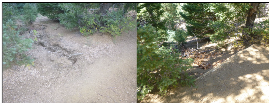
Figure 34. Before (left) and after (right) of timber retaining wall construction.
