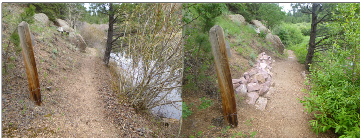
Figure 27. Before (left) and after (right) of retaining wall constructed to mitigate erosion adjacent to a pond.
