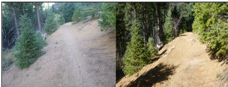
Figure 35. Before (left) and after (right) of trail improvement and timber retaining wall.
