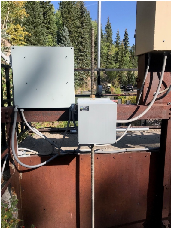
Figure 5 SCADA system at diversion
