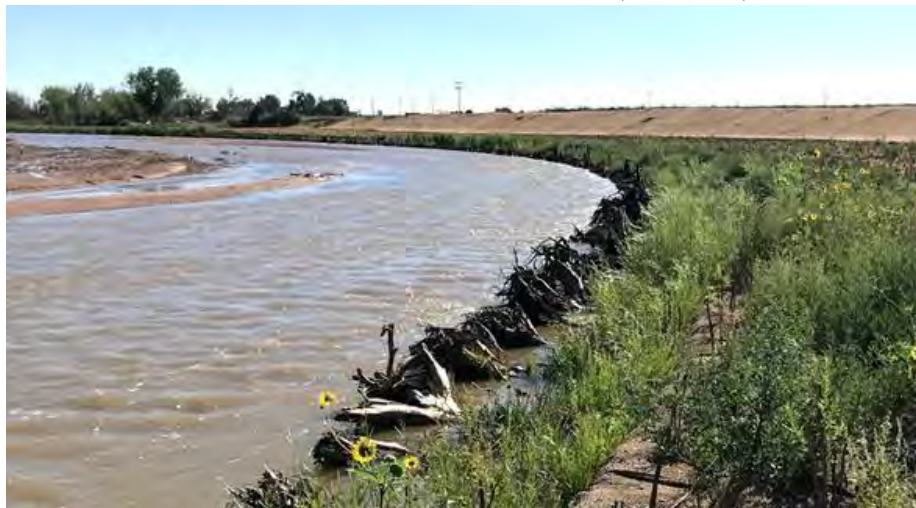
Figure 16: Toe Wood with Soil Lifts
