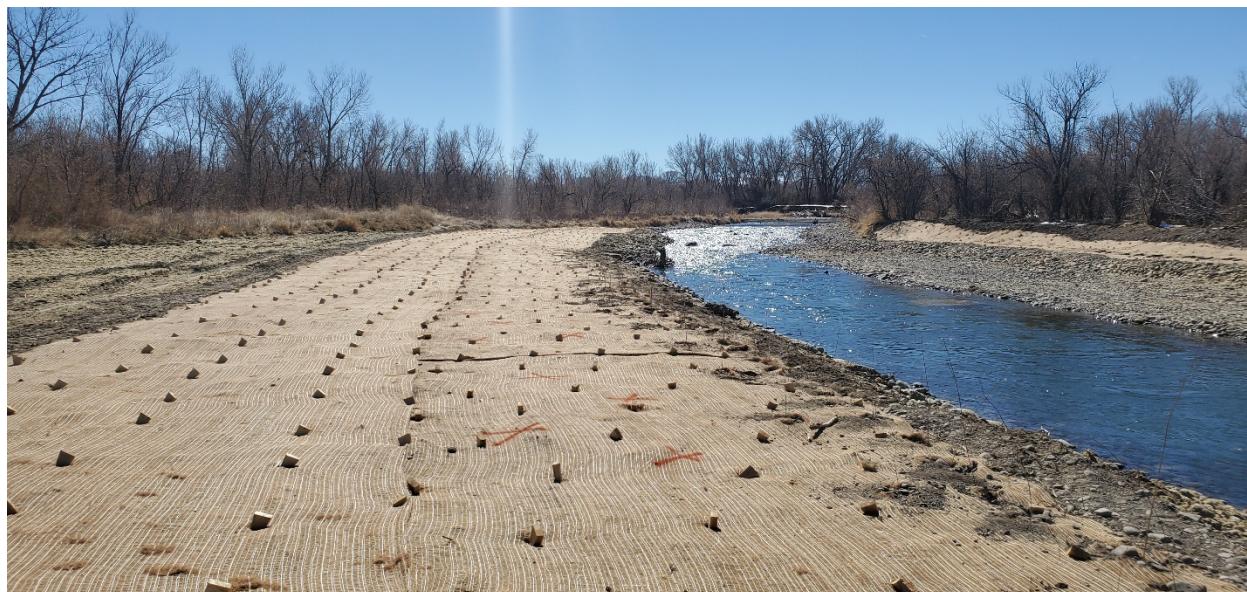
Fabric for Stabilization
