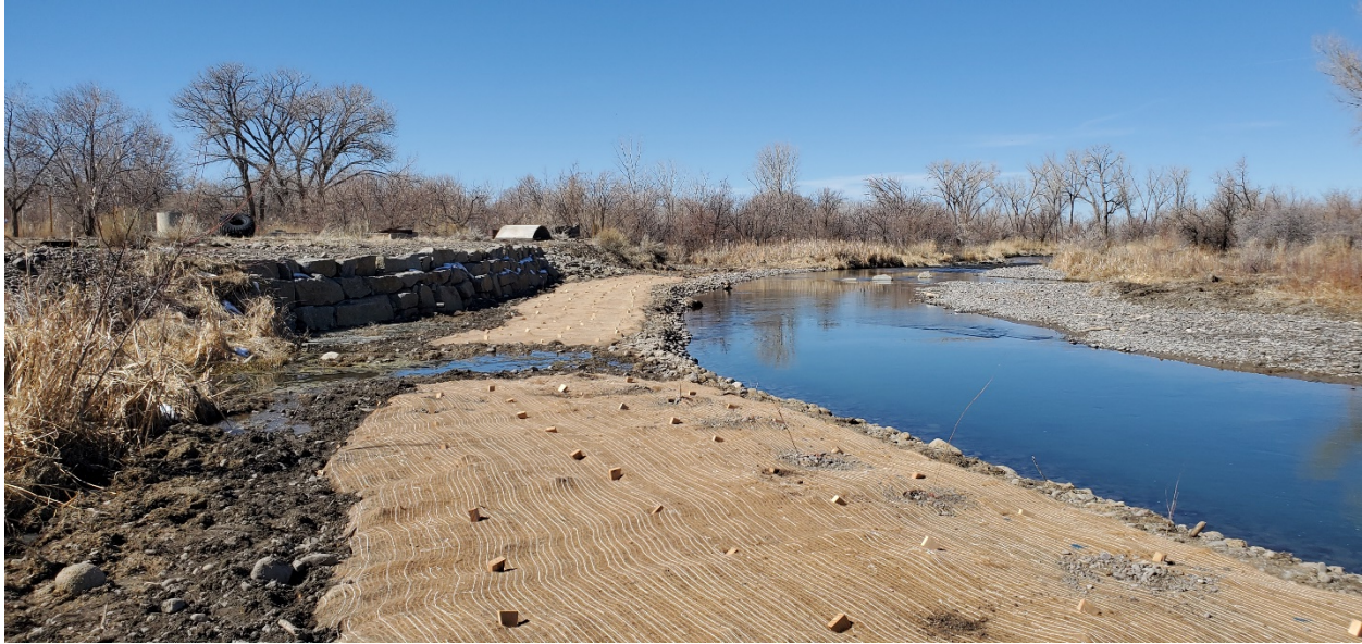
Native and Rock Wall Stabilization along Glide
