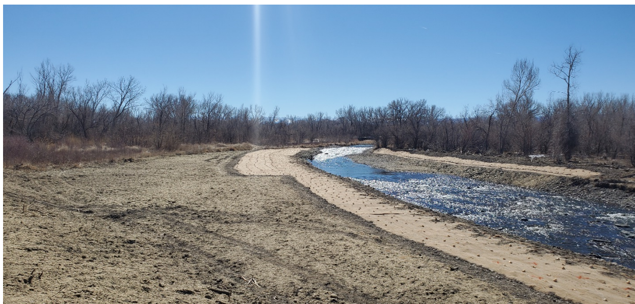
Terrace Grading with Seeding and Fabric
