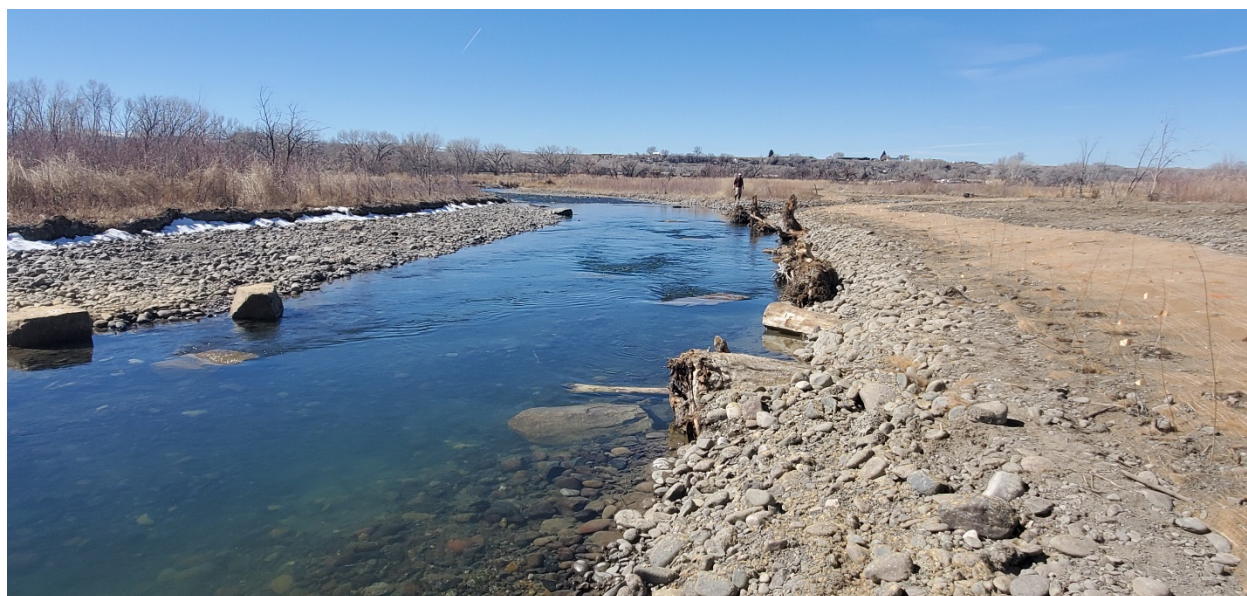
Rootwad Stabilization with Plantings
