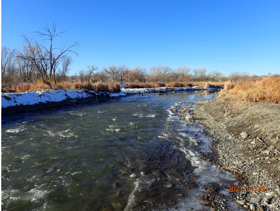
Constructed Riffle
