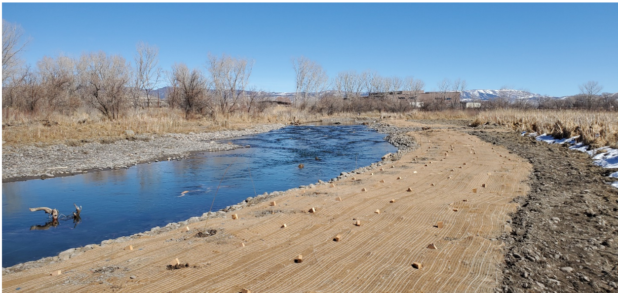
Overbank Grading and Stabilization with Habitat Features
