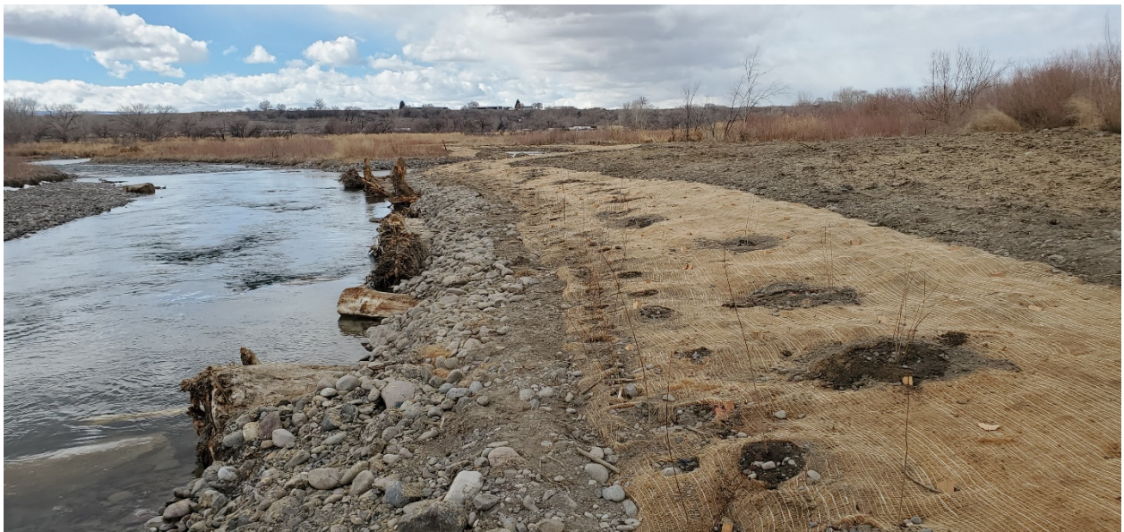
Bank Stabilization with Roots and Vegetation
