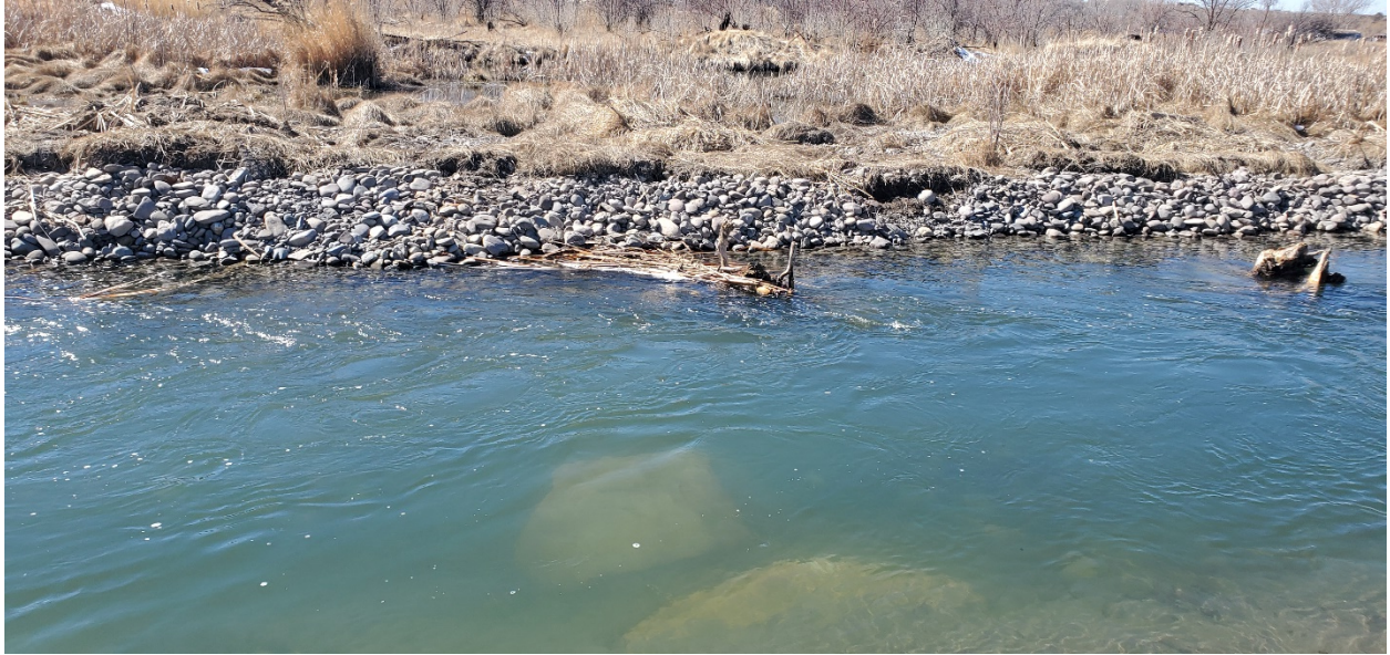
Bank Stabilization with Habitat Features
