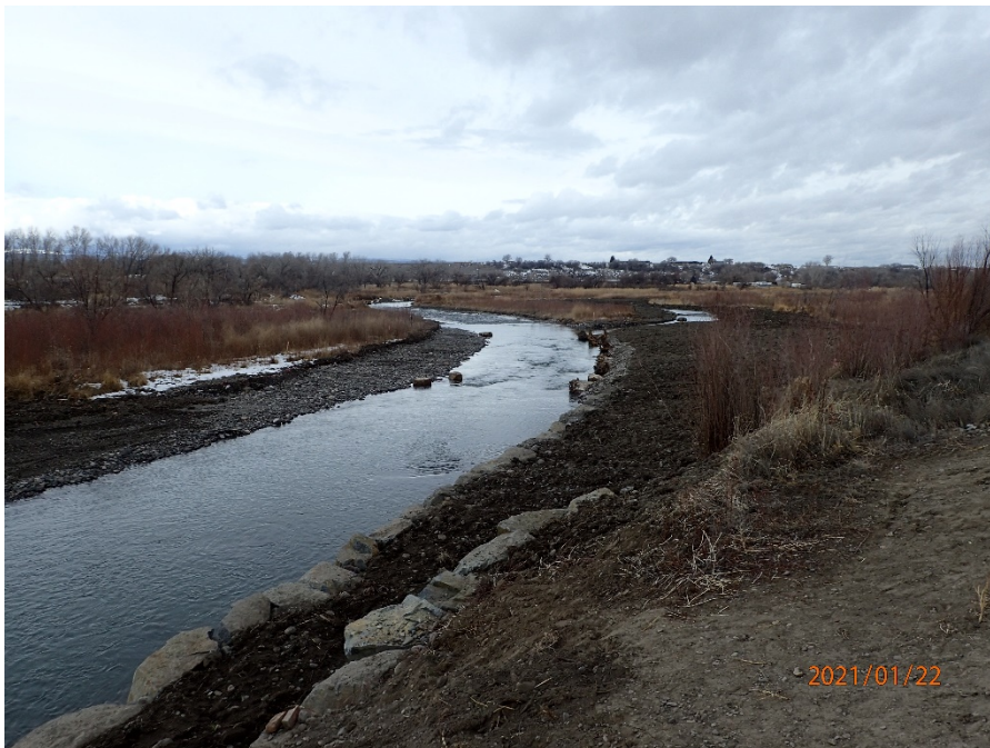
Rock Wall Stabilization (foreground) and Log Stabilization (background)
