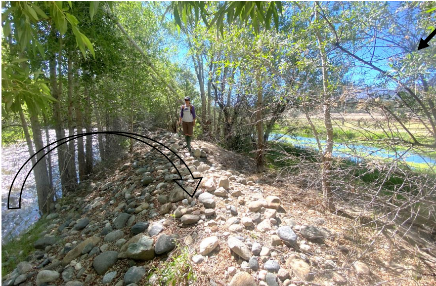
↑ Levees like these (above and below) were constructed during channelization projects in the 1940s or 50s by excavating the channel bed to build berms to create an incised channel with elevated banks—a double-whammy in terms of entrenchment. ↓
