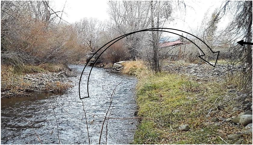
↑ Levees like these (above and below) were constructed during channelization projects in the 1940s or 50s by excavating the channel bed to build berms to create an incised channel with elevated banks—a double-whammy in terms of entrenchment. ↓
