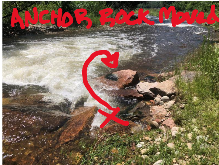
Figure 1- Cross channel structure stability, rock movement, looking downstream
