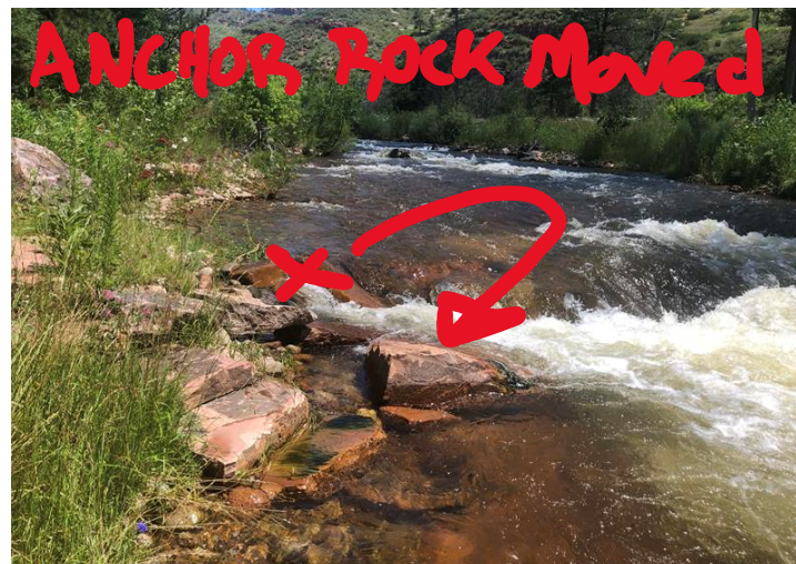
Figure 1- Cross channel structure stability, rock movement, looking downstream
