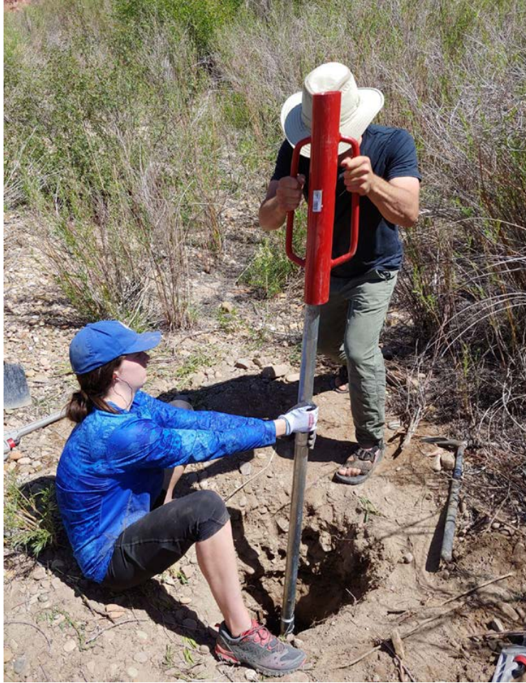
Figure 5: Fort Lewis College Students install groundwater wells at the Big Gypsum site. Phot: Dr. Melissa Clutter.
