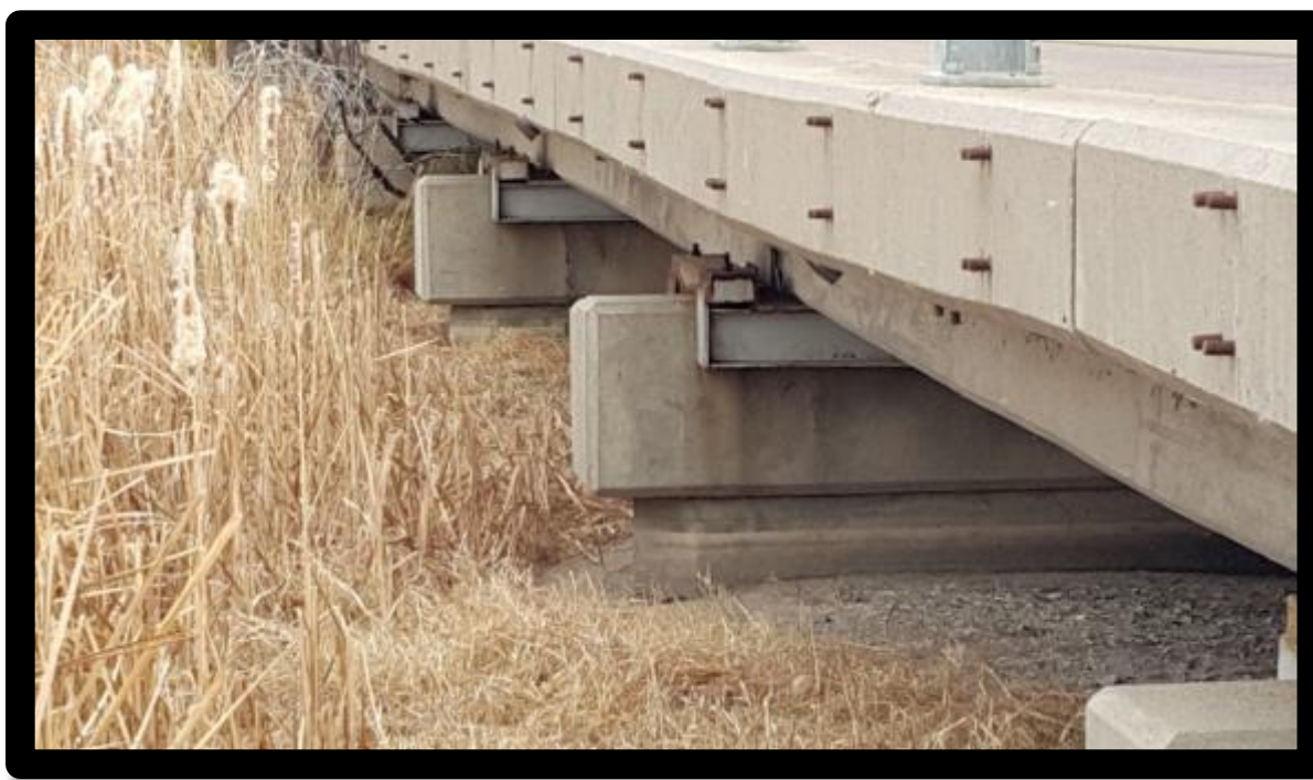
Photo 5: Highway 385 Bridge – silt and cattails have reduced clearance from 8+ feet to 3-4 feet
