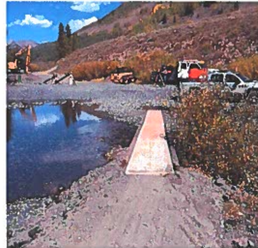
Photo 4: Temporary bridge built for trail users for duration of project.
