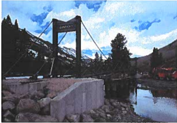
Photo 7: Main cable installation across bridge.
