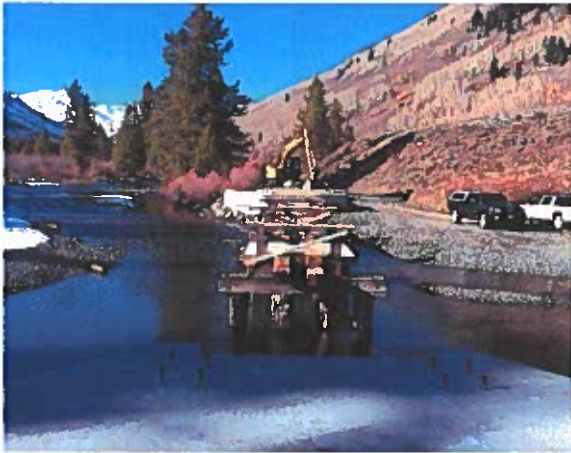
Photo 1: Scaffolding built on top of old bridge with deck and railings removed.
