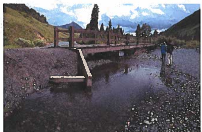
Photo 12: Former Gunsight Bridge with eroded wingwall and deteriorating support piers.
