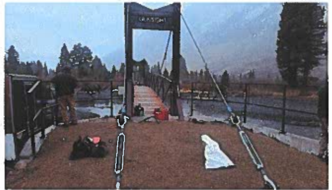
Photo 10: Hand railing installation on wingwalls.
