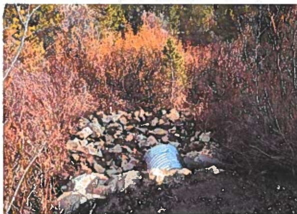
Photo 11: Rock spill pad beneath the culvert's eastern end.
