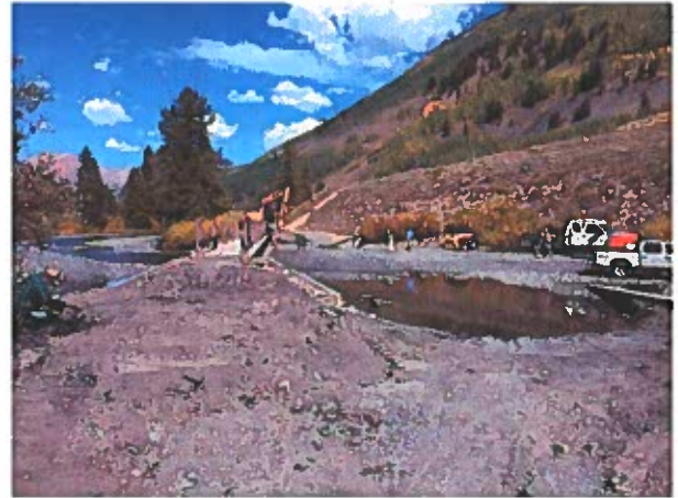
Photo 2: Project team siting location for micro piles after grading the new abutment area.
