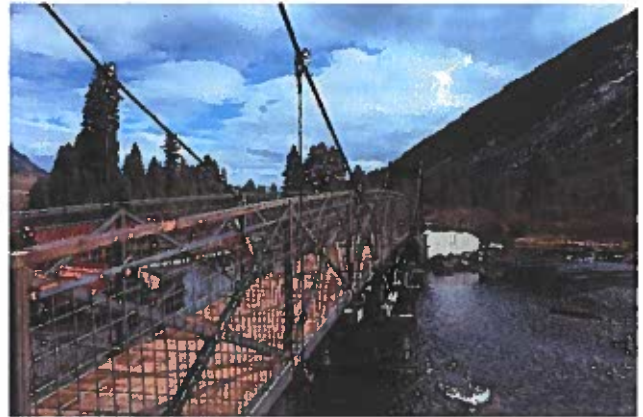
Photo 8: Suspension cable installation from main cable to bridge deck.
