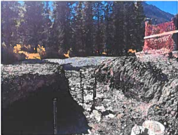
Photo 3: Micro pile installation at southern (downstream) abutment.
