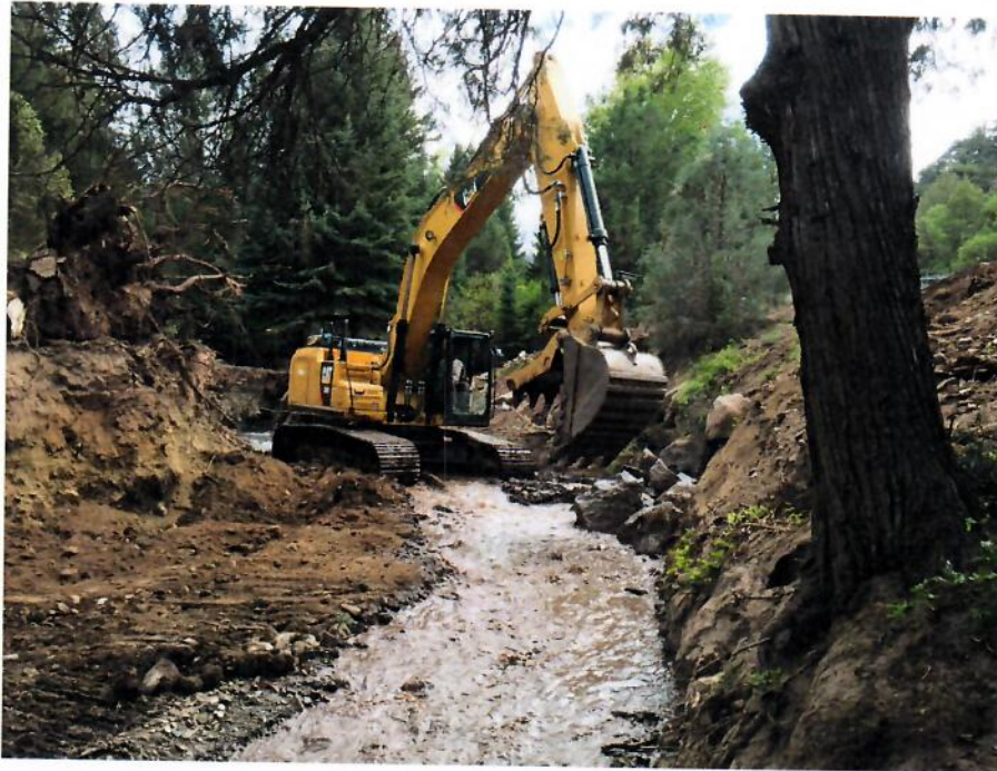
This photo shows the excavator at work. The protrusion has been removed in the left center of the photo.
