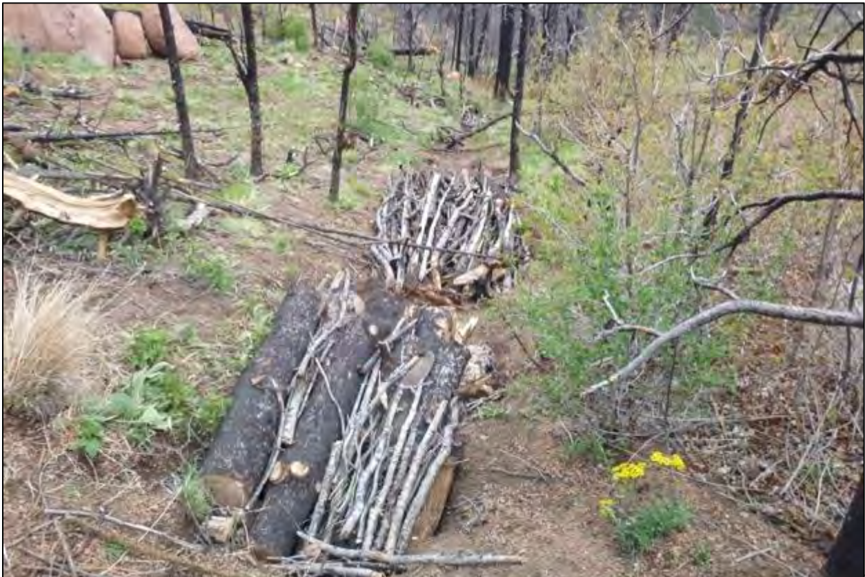
Figures 15 & 16. Before and after photo (top and bottom) showing construction of a debris filter within an eroded drainage of Waldo Canyon.
