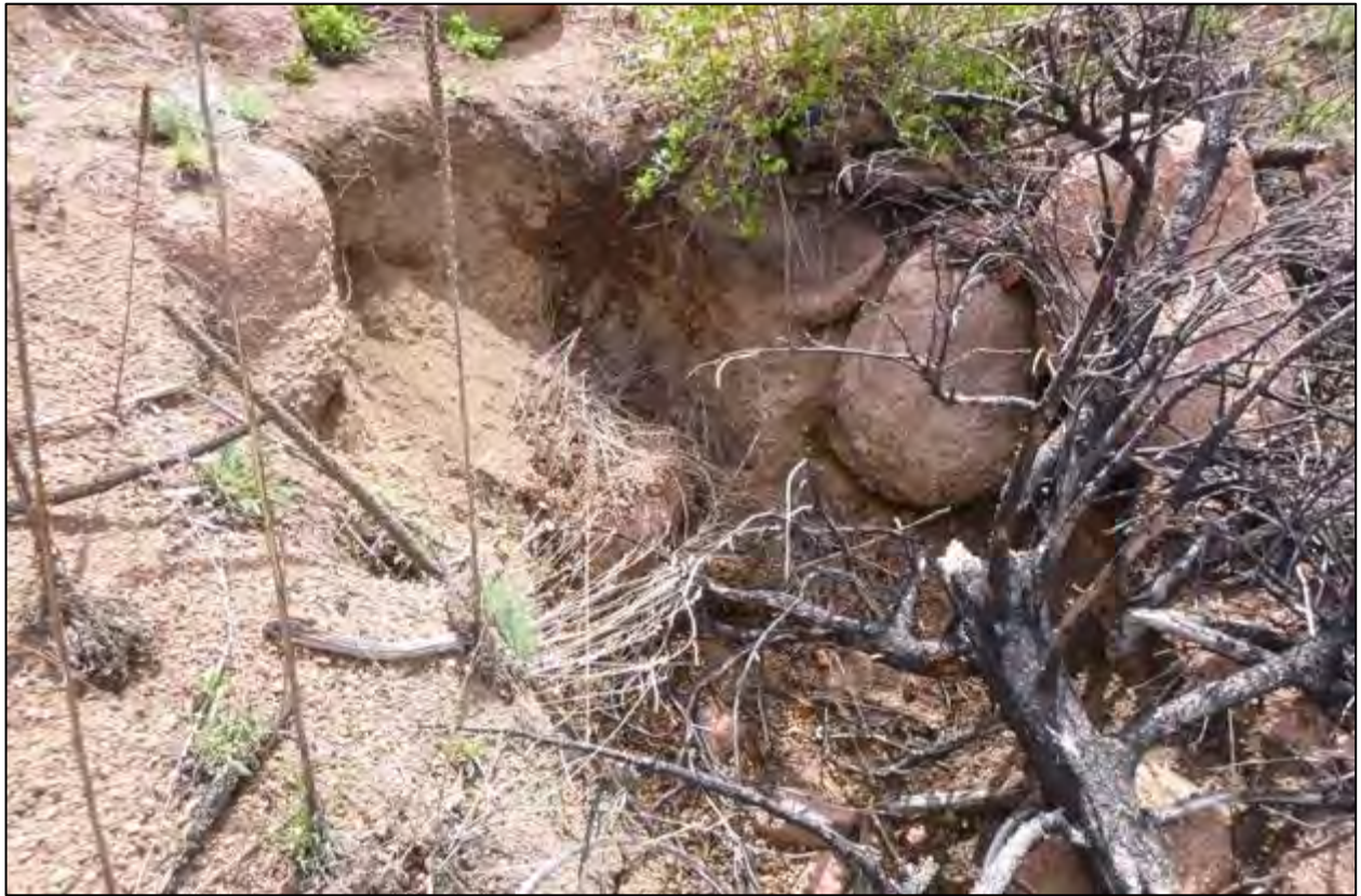
Figures 17 & 18. Before (above) and after (below) photos showing log step-fall construction to stabilize an eroding head-cut in the Waldo Canyon drainage.
