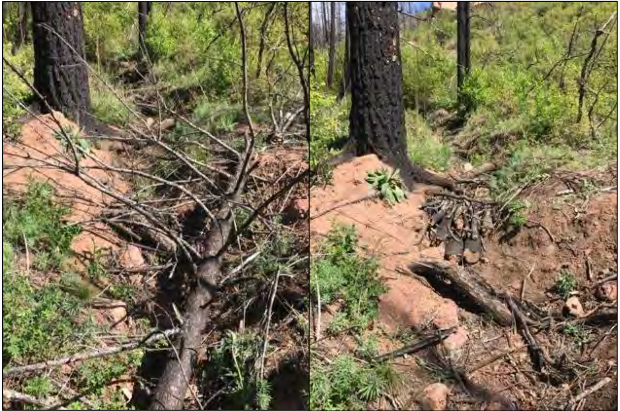
Photos 19 & 20. Before and after photo (top and bottom) showing construction of a debris filter within an eroded drainage of Waldo Canyon.
