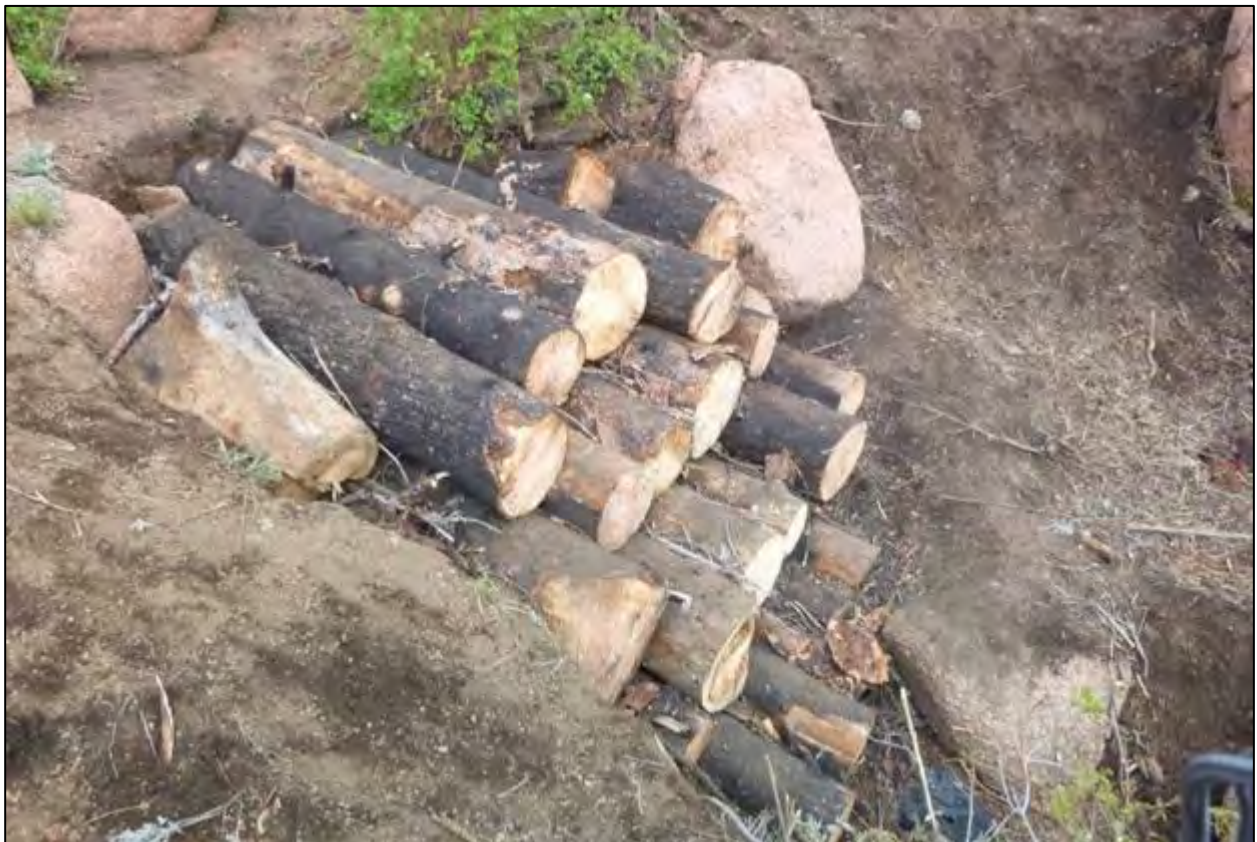
Figures 17 & 18. Before (above) and after (below) photos showing log step-fall construction to stabilize an eroding head-cut in the Waldo Canyon drainage.
