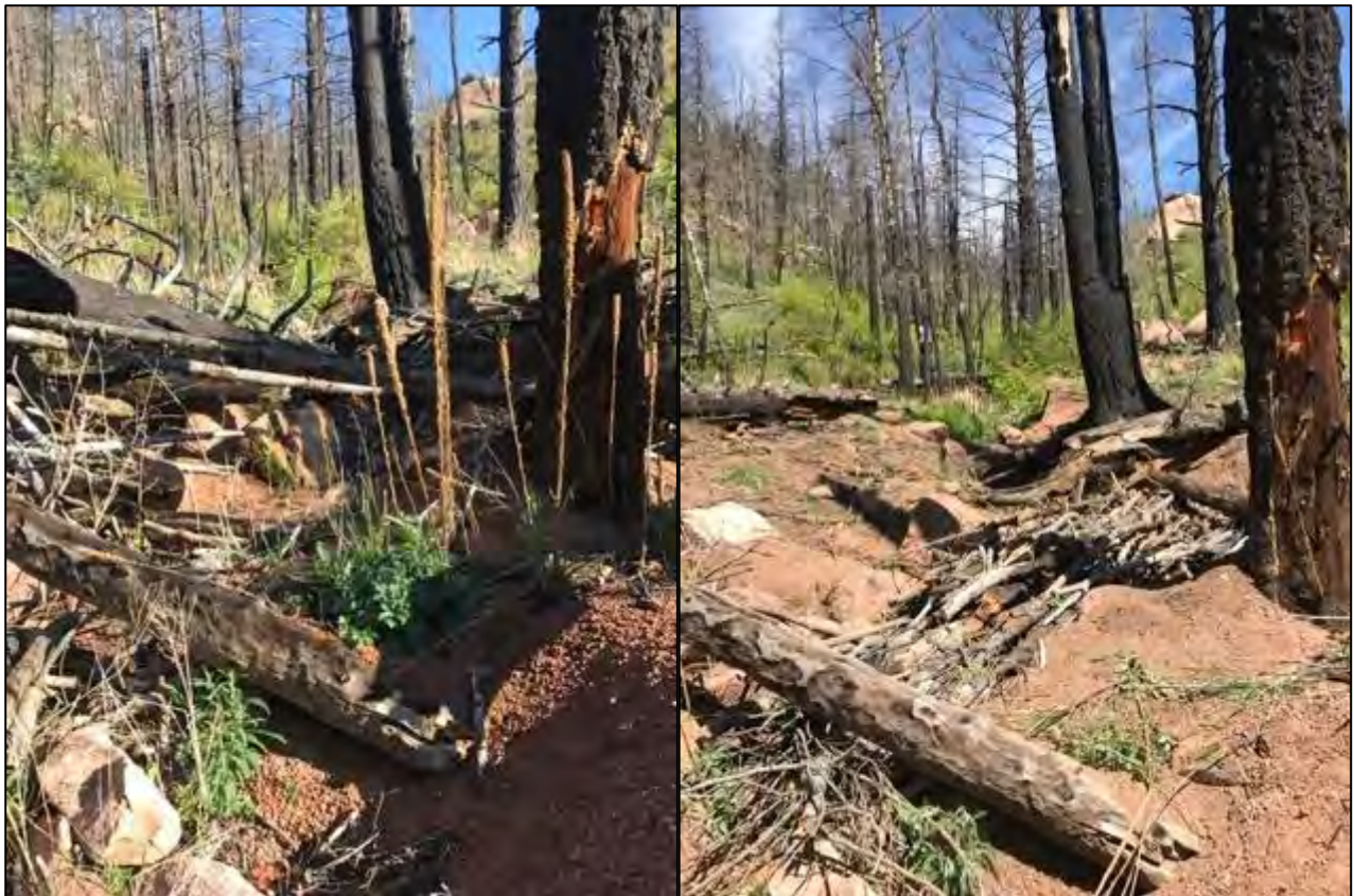
Photos 19 & 20. Before and after photo (top and bottom) showing construction of a debris filter within an eroded drainage of Waldo Canyon.
