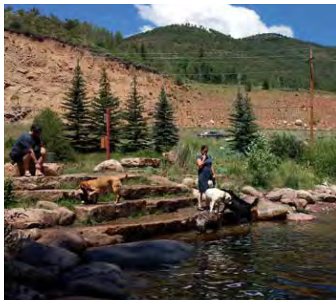
Image 4-6 An example of a bank repaired with boulders and steps
