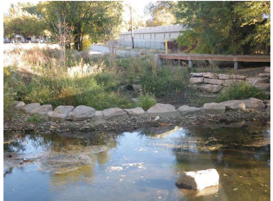
Stormwater retention wetland and boardwalk from the Ogden River Restoration provides an opportunity for public education on green infrastructure principles
