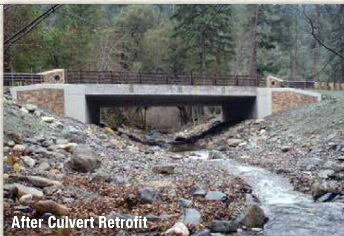
Retrofitted bridge to allow fish passage in Fort Goff Creek, Klamath National Forest, California. Photo courtesy of USFS.
