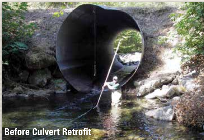
Bridge culvert impeding fish passage in Fort Goff Creek, Klamath National Forest, California. Photo courtesy of USFS.
