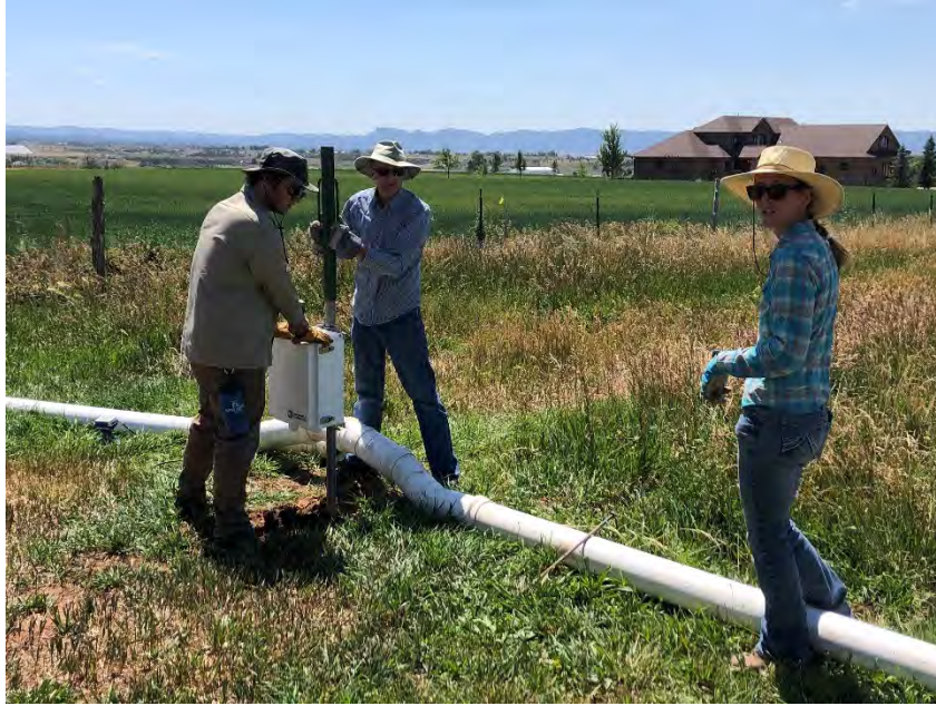
Installation of the equipment
