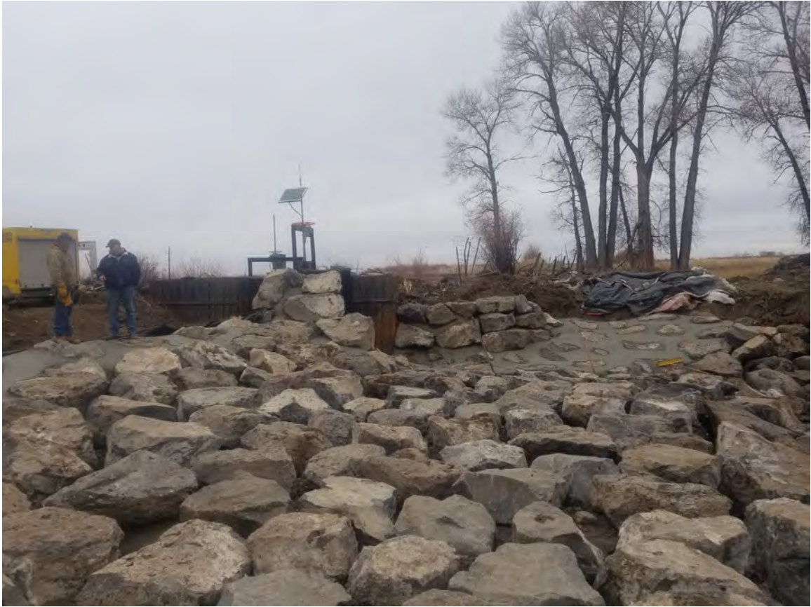
New sluice and automation hardware for the Richfield ditch in background. Rock placement ready for grout in foreground.
