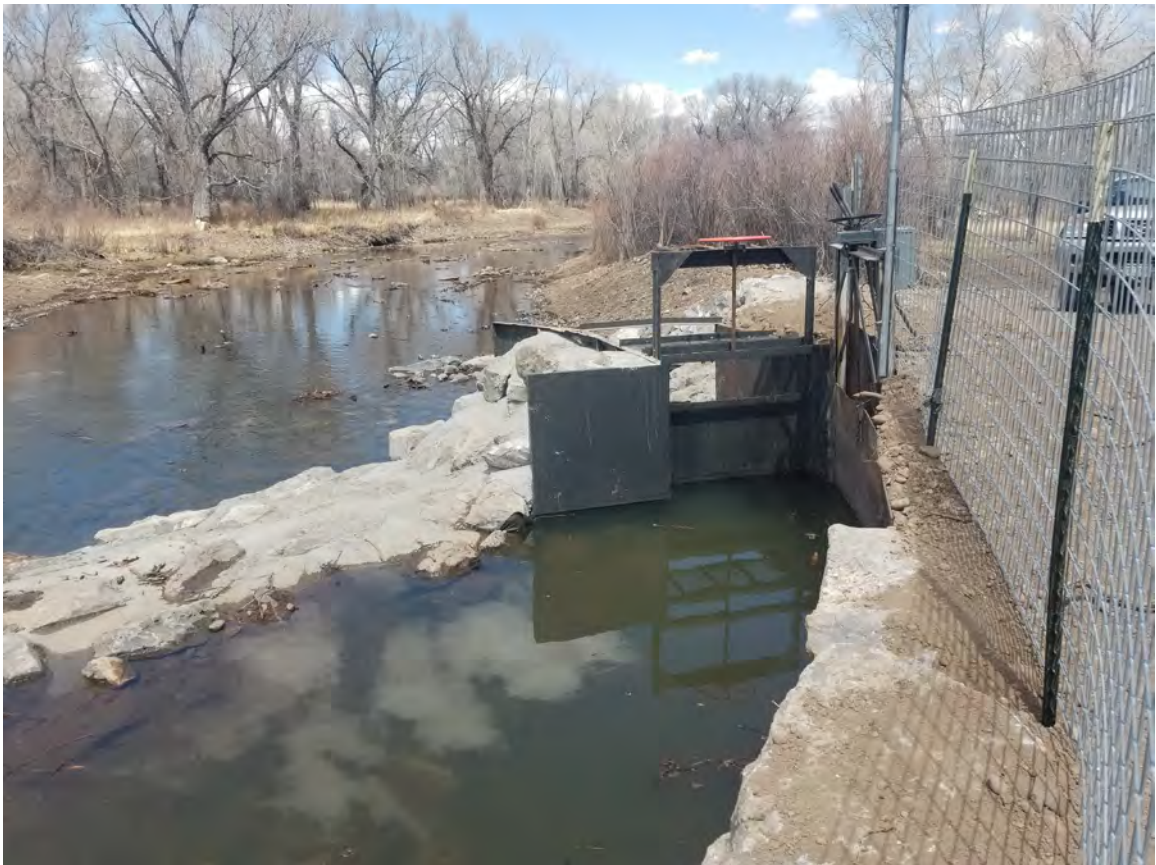
Looking downstream at the new 6&10 sluice and grouted rock core. Just to the right of the Sluice you can see the new automation hardware.
