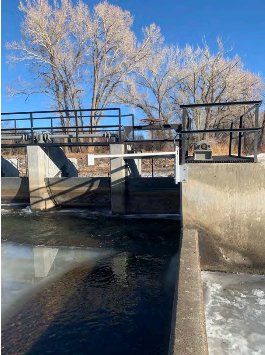
New downward facing radar unit for measurement at Conconco. During low water flows this unit will be swung back over the concrete core and will control the existing automatic gates to ensure compact flows pass this area of the River.
