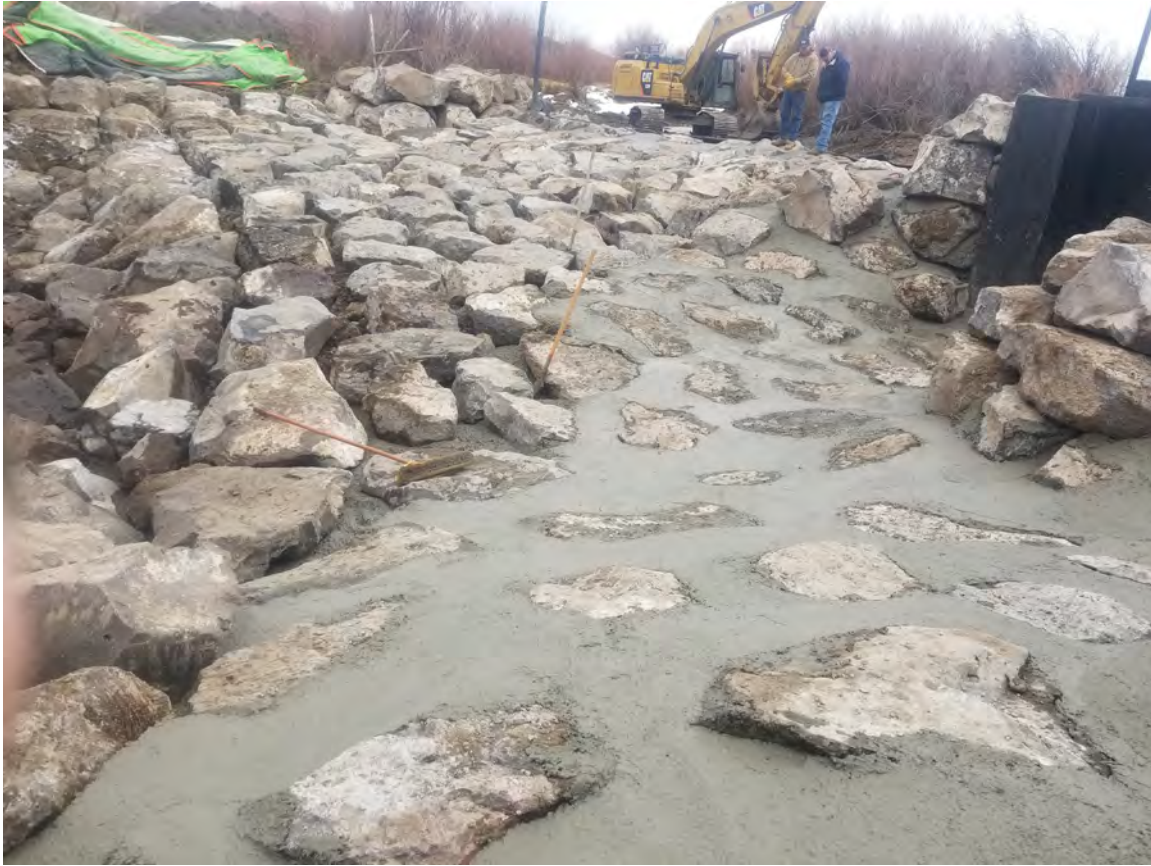
Beginning of the grouting process for the sluice and crossing structure at the Richfield diversion
