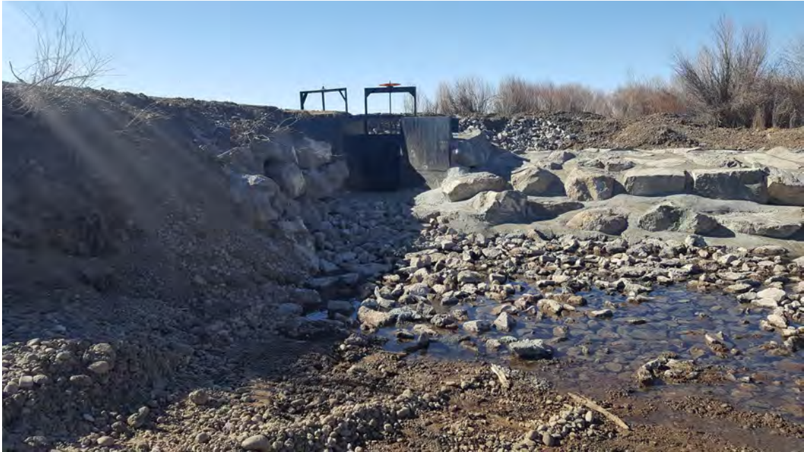
New sluice structure and grouted core at the Salazar (8&12)
