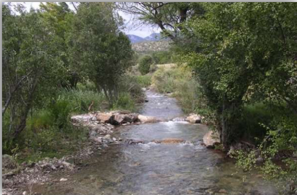
Photo 12. Rock Cross vanes with scour pool below structure.
