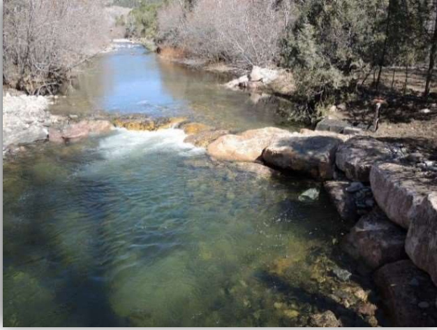
Photo 30. Example of Rock Cross Vane Structure connected to rock toe protection.
