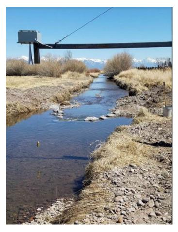
Saguache Creek at Cemetery Road- Cantilever and Radar Installation (Division 3). Note these installations are more cost efficient as they require significantly less infrastructure than a typical stilling well and shelter.
