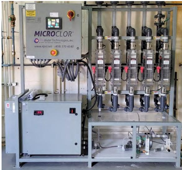
**Figure 8 – Chlorine Dosing Equipment**
