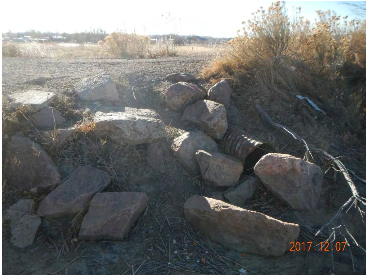
21_Pipe Spillway on left end of dam
