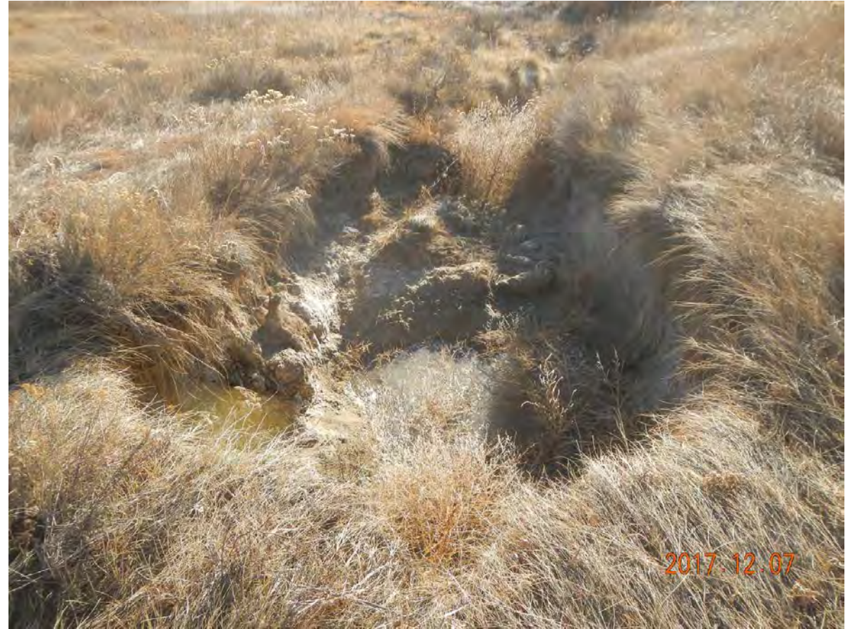
24_Em Spwy headcutting
