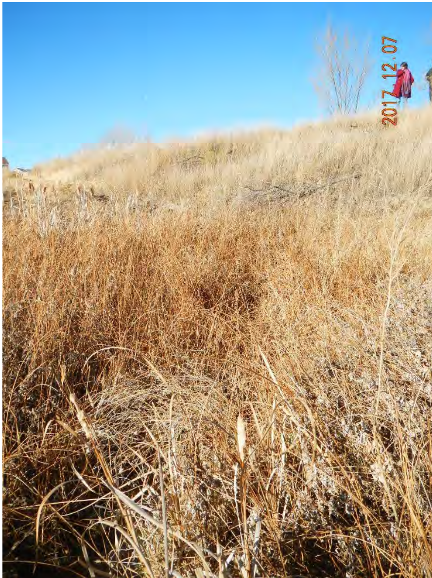
11_Downstream Slope, above old outlet
