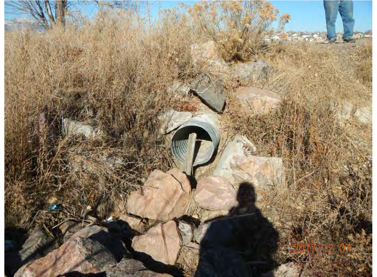
22_Pipe spillway on left end of dam
