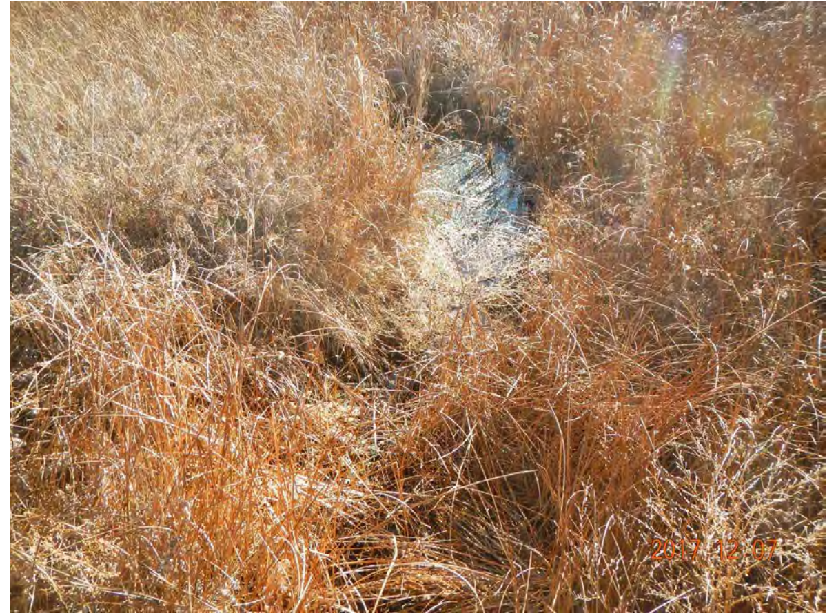
20_Seepage area left of old outlet
