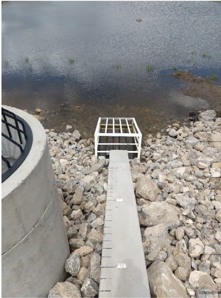
Figure 2. Von Springs #1 – Low-Level Outlet with Grade Beam, Service Spillway Standpipe at Left
