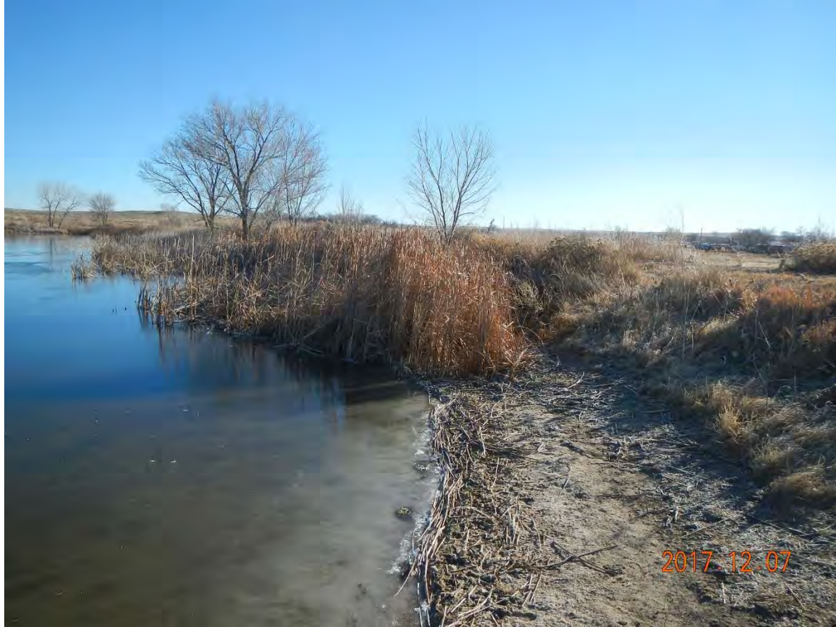
01_Upstream Slope, from right abutment
