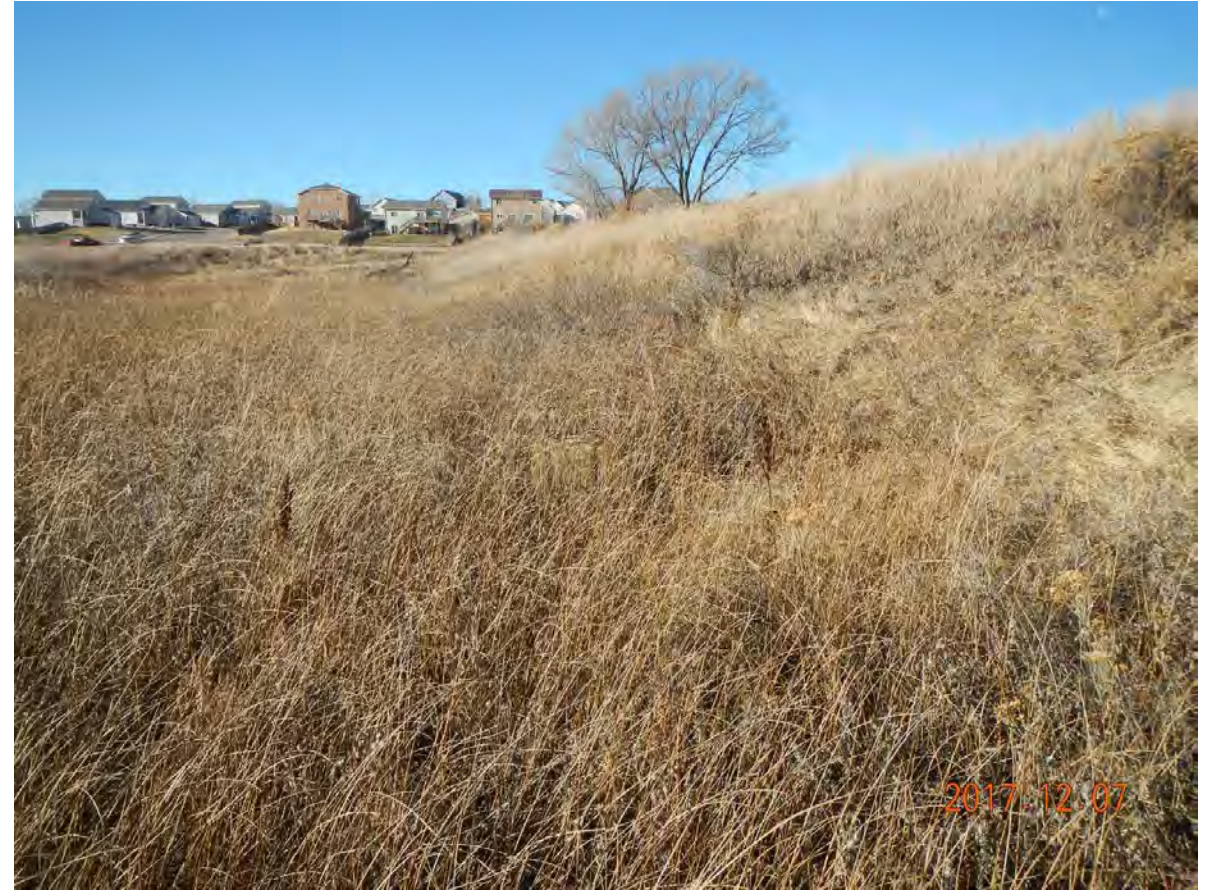
10_Downstream Slope, looking right at central portion
