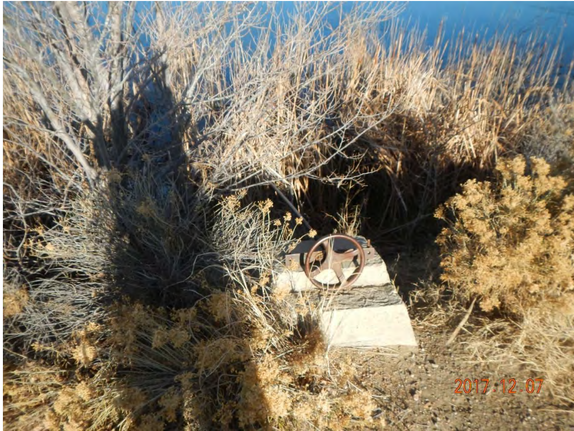
15_Outlet, old operator
