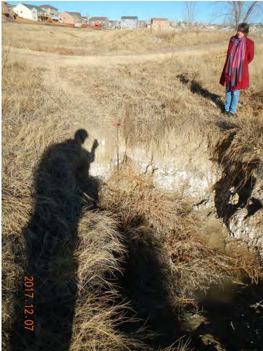
25_Em Spwy Headcutting
