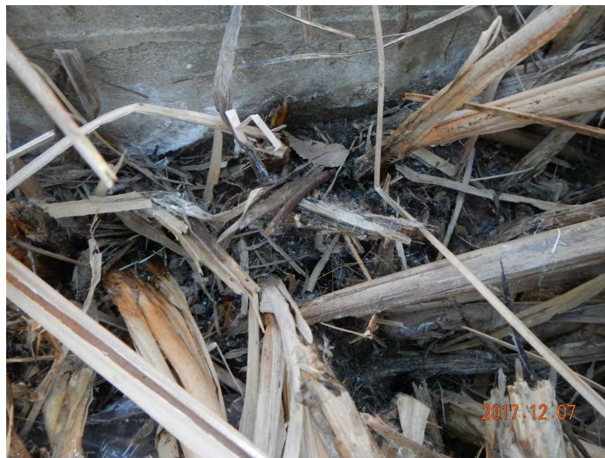
18_Outlet, old discharge point concrete
