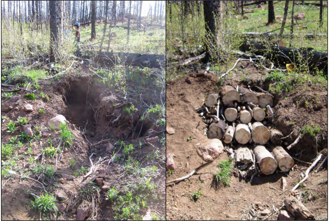
Figure 11. Before (left) and after (right) showing headcut stabilization treatment.
