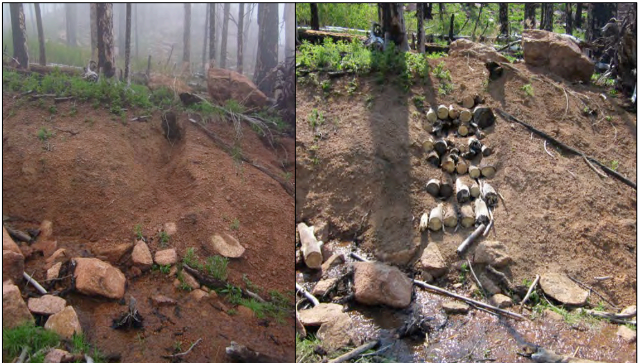
Figure 12. Before (left) and after (right) of a stepfall construction technique to stabilize the stream channel.
