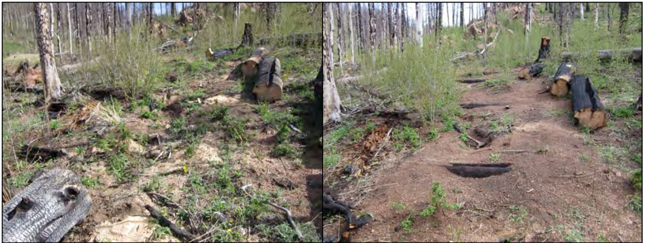
Figure 10. Before (left) and after (right) photos showing sills emplaced in a side drainage to stabilize the slope.
