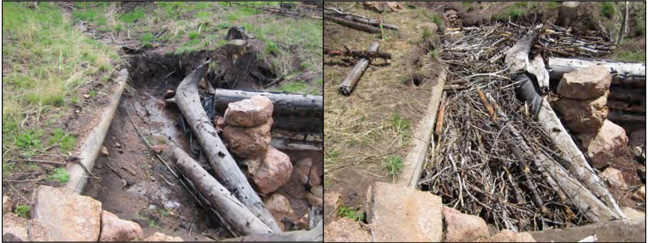
Figure 9. Before (left) and after (right) photos of headcut stabilization treatments completed by RMFI and MHYC.
