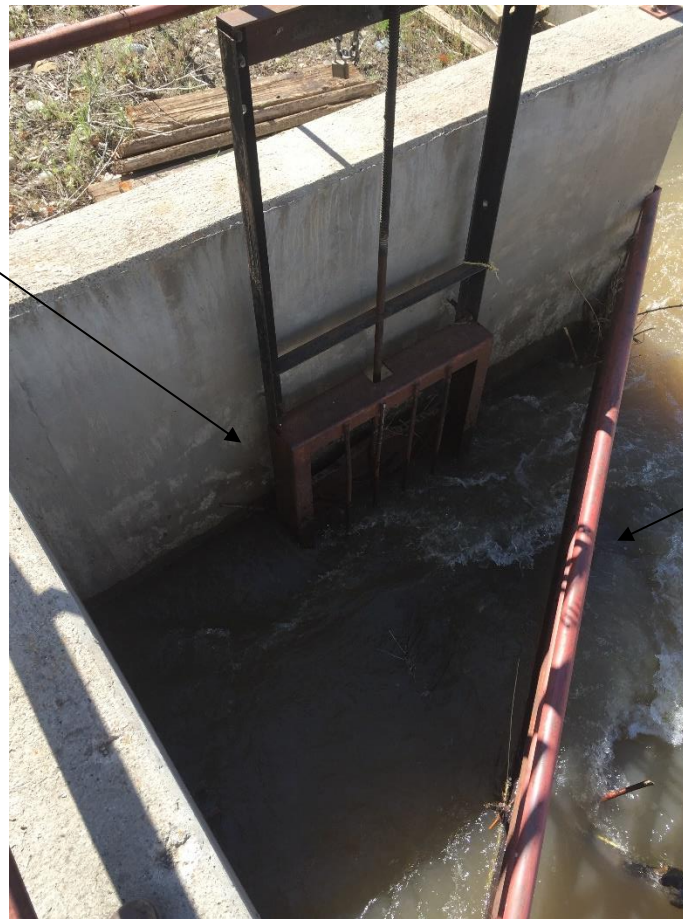
Figure 2.8.1.4. Canal Headgate with Safety Fence
