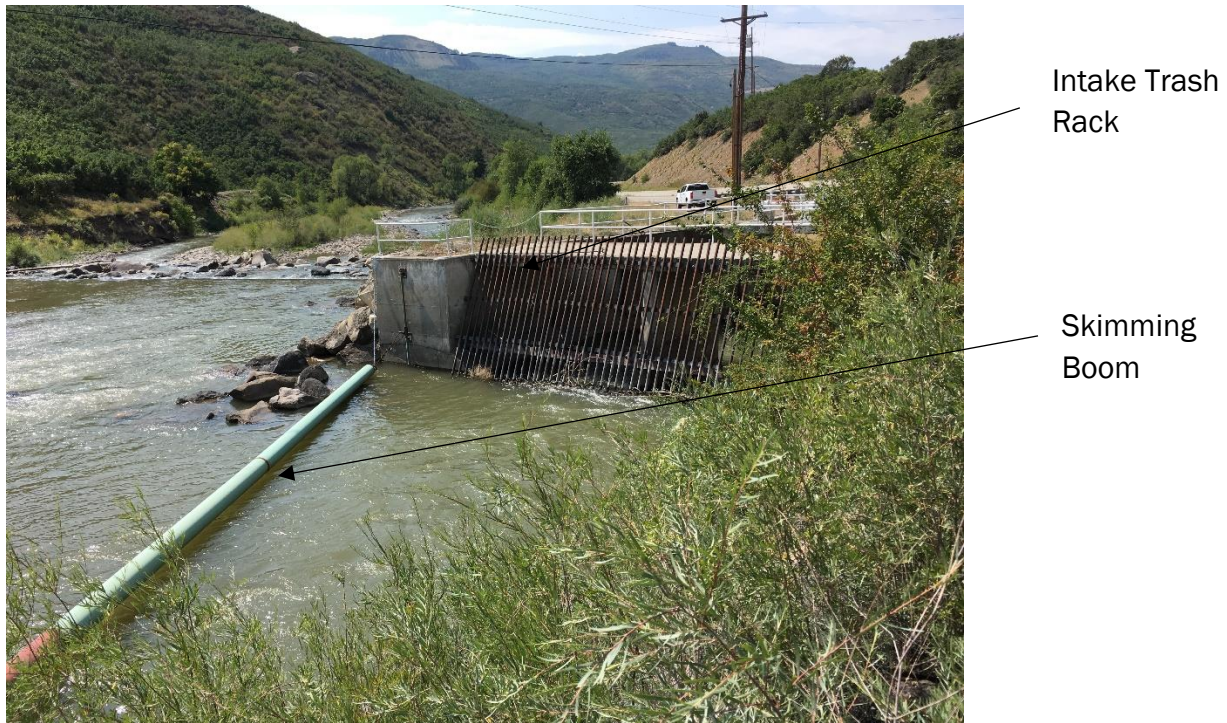
Figure 2.2.1.4. Fire Mountain Canal Intake Structure
