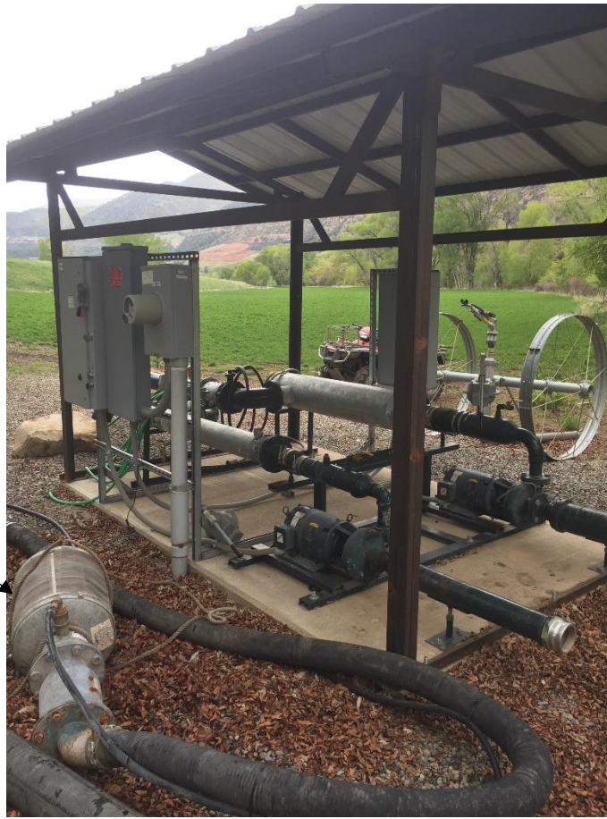
Figure 2.2.3.4 Lennox Ditch Pump System to Convey Irrigation Water
