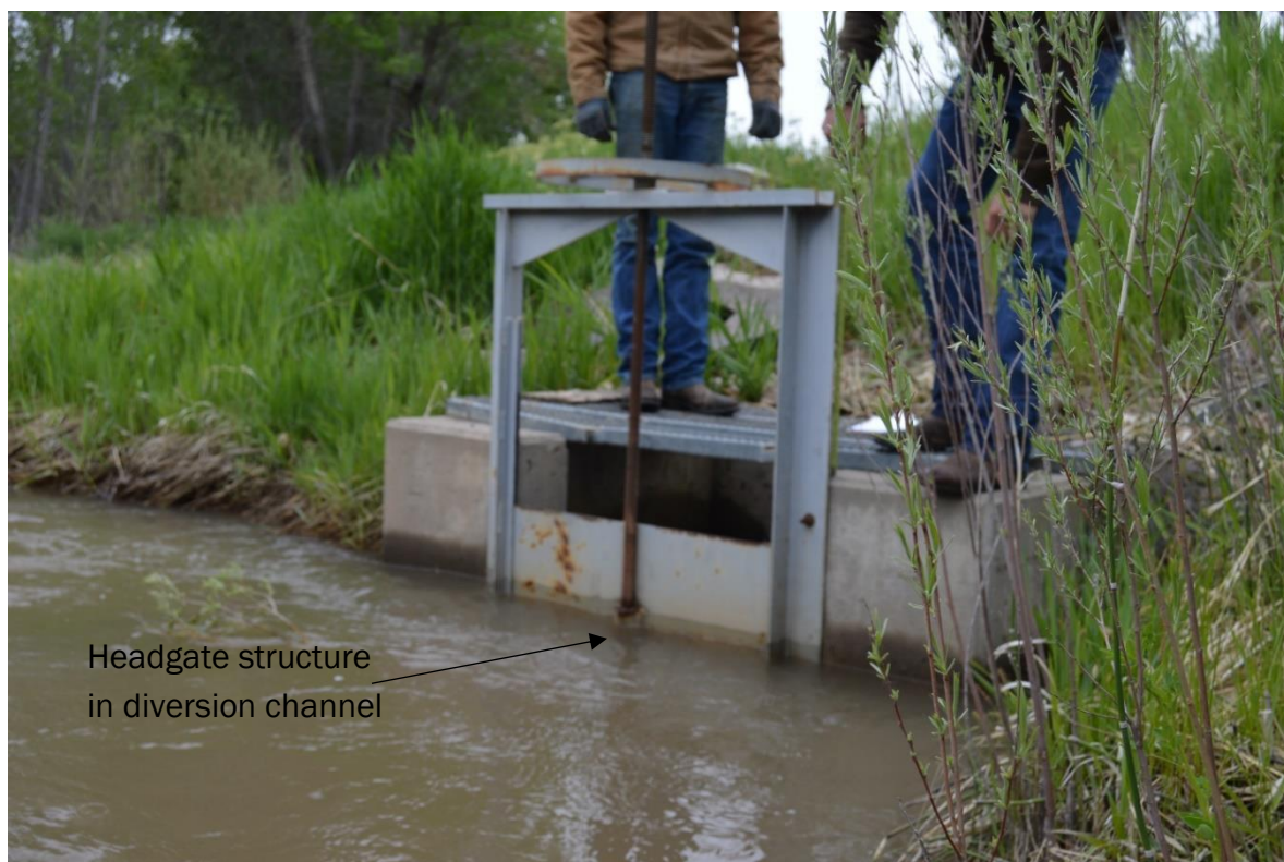
Figure 2.5.2.6. Monitor Ditch Headgate
