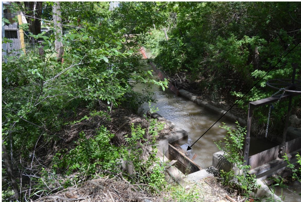
Figure 2.5.1.6. Paonia Ditch Secondary Spill and Headgate
