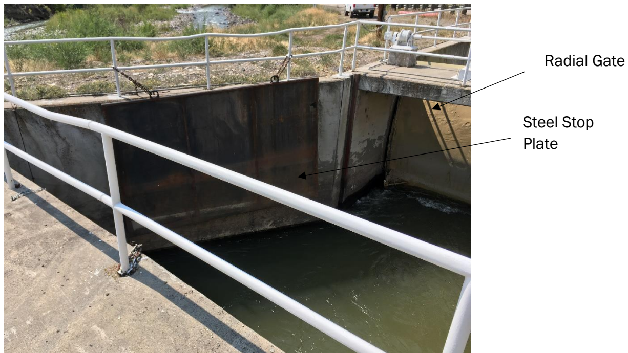
Figure 2.2.1.5. Radial Gate and Steel Stop Plate within Fire Mountain Canal Intake Structure
