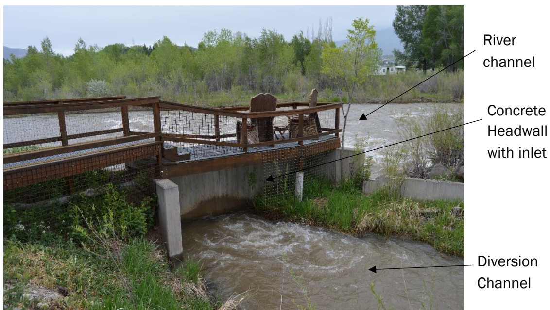
Figure 2.5.2.4. Concrete Headwall for Monitor Ditch at River Diversion
