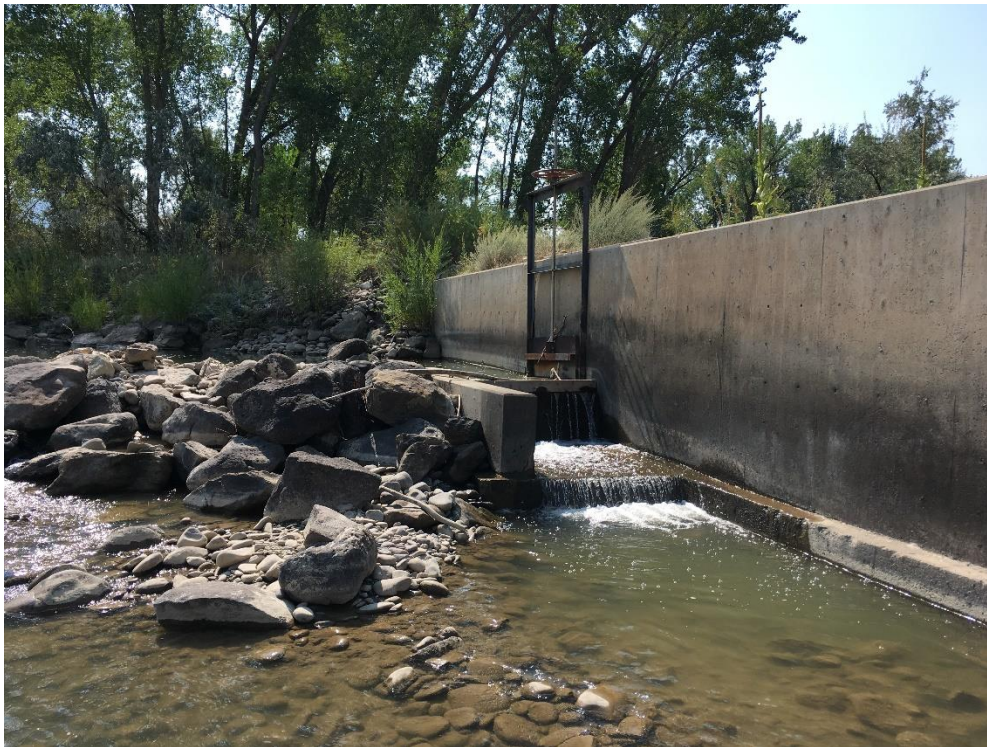
Figure 2.6.1.4. Short Ditch Diversion Headwall and Intake
