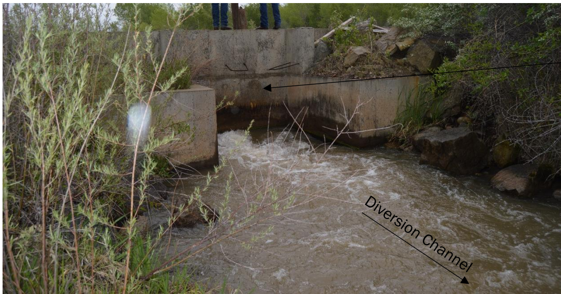
Figure 2.5.3.4. Concrete Headwall and Intake Structure from Diversion Channel
