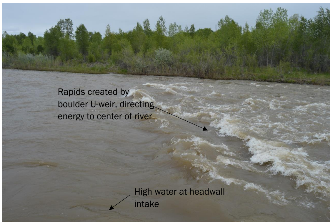
Figure 2.5.2.3. Resultant Water Profile from Monitor Ditch Diversion
