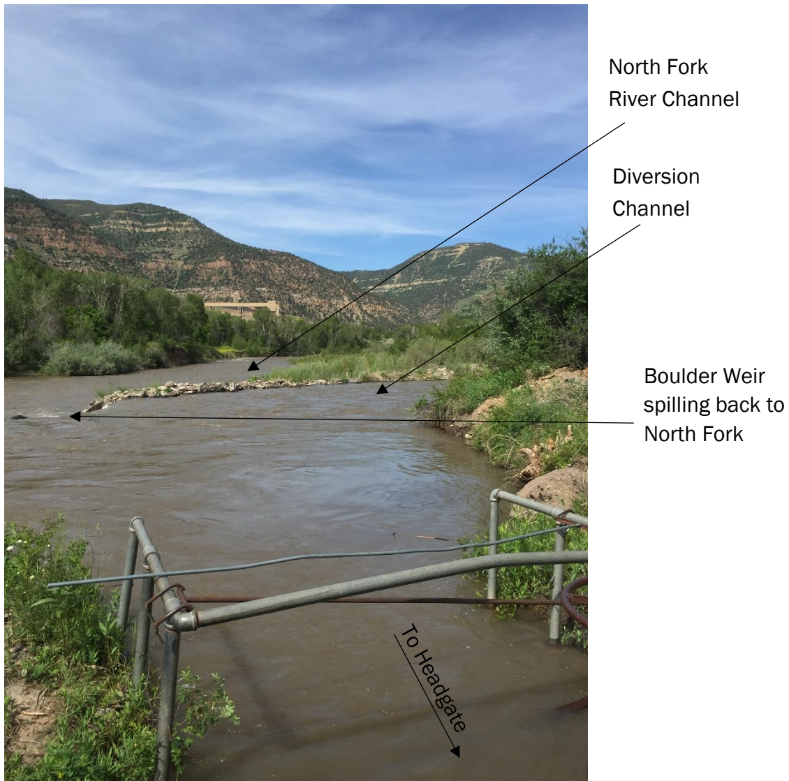
Figure 2.3.1.3. View of Stewart Ditch Diversion Channel from Headgate
