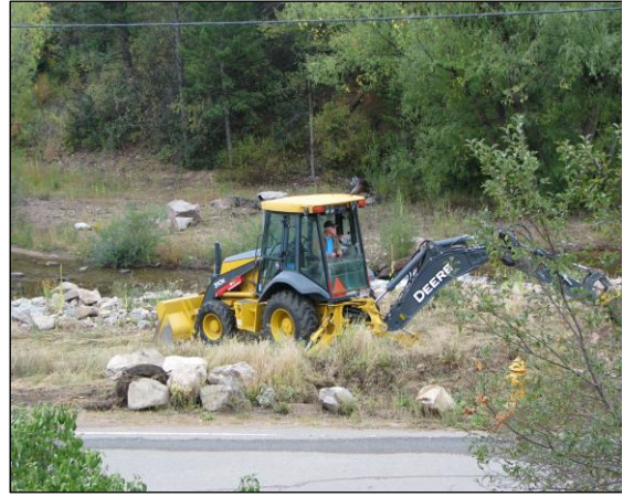
Figure 2. Project Site 1 backhoe operation to dig under invasive weeds, spread topsoil, and dig holes for planting trees and shrubs
