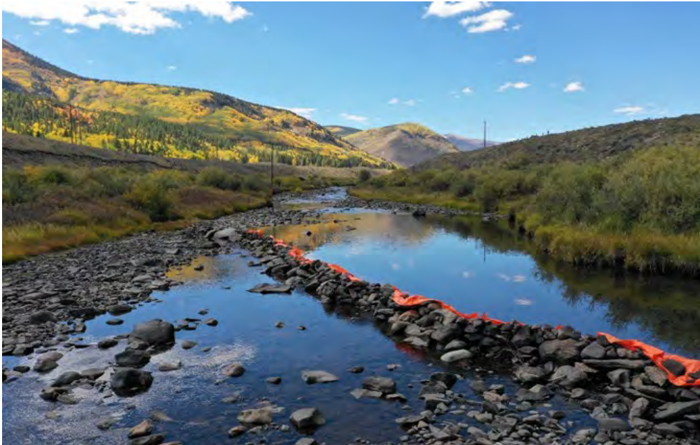
Photo 16-2: A large diversion in the Slate River caused substantial dry down during early fall 2018. The diversion structure dried a portion of the channel (see left side of photo) and the push-up dam prevented fish passage. The diversion structure also increases labor costs for the irrigator.
