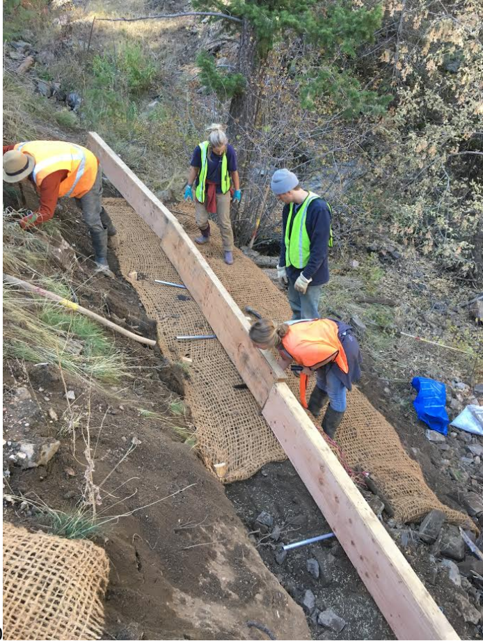
Started soil lifts Right bank +- Station 4+00
