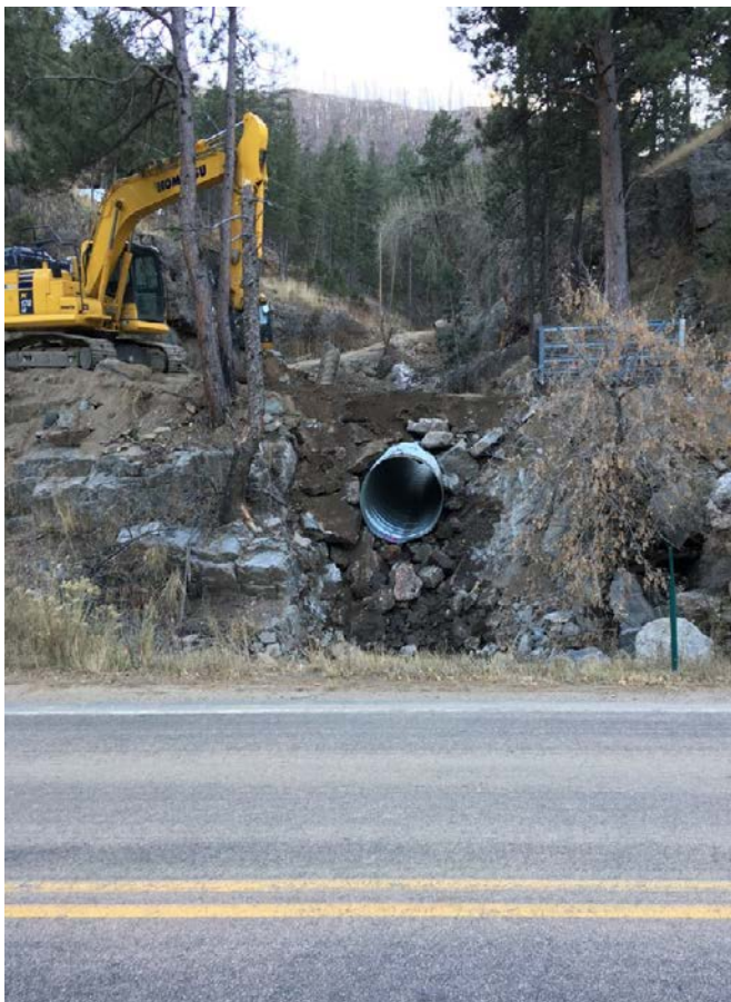
Photo 5. 60" bottom culvert installed (replaced 18" culvert)
