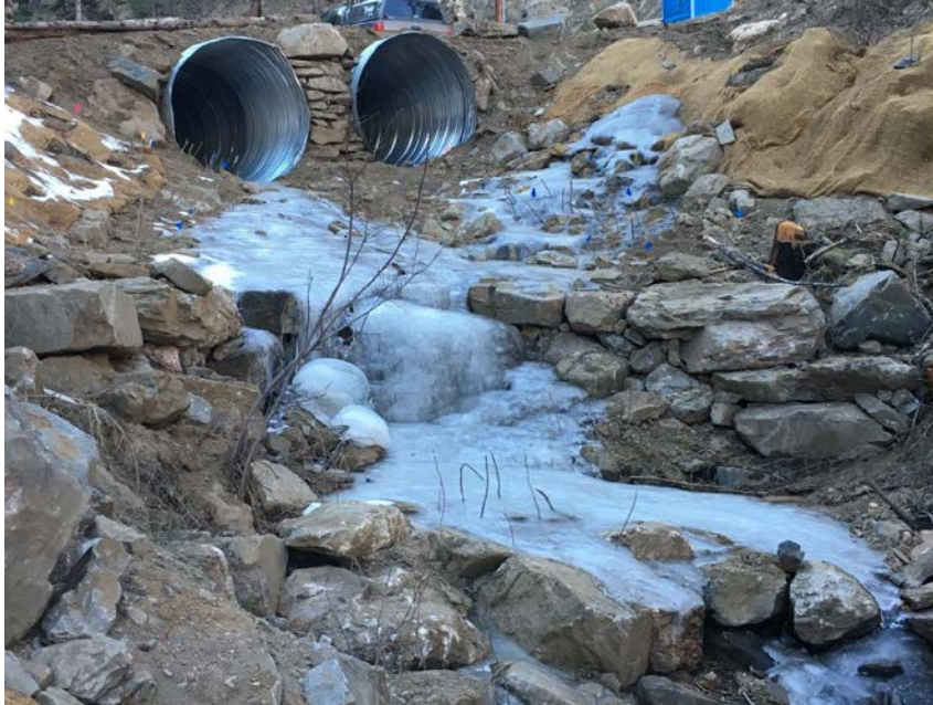
Photo 4. Two 72" culverts installed (replaced two 36" culverts) Stone toe was placed on both banks for approximately 30', along with coir matting, seed, container plantings, and willow stakes
