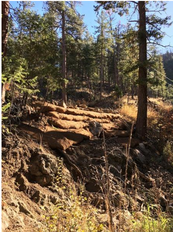
Photo 6. View Upstream Station 4+50 Vegetated Soil Lifts
