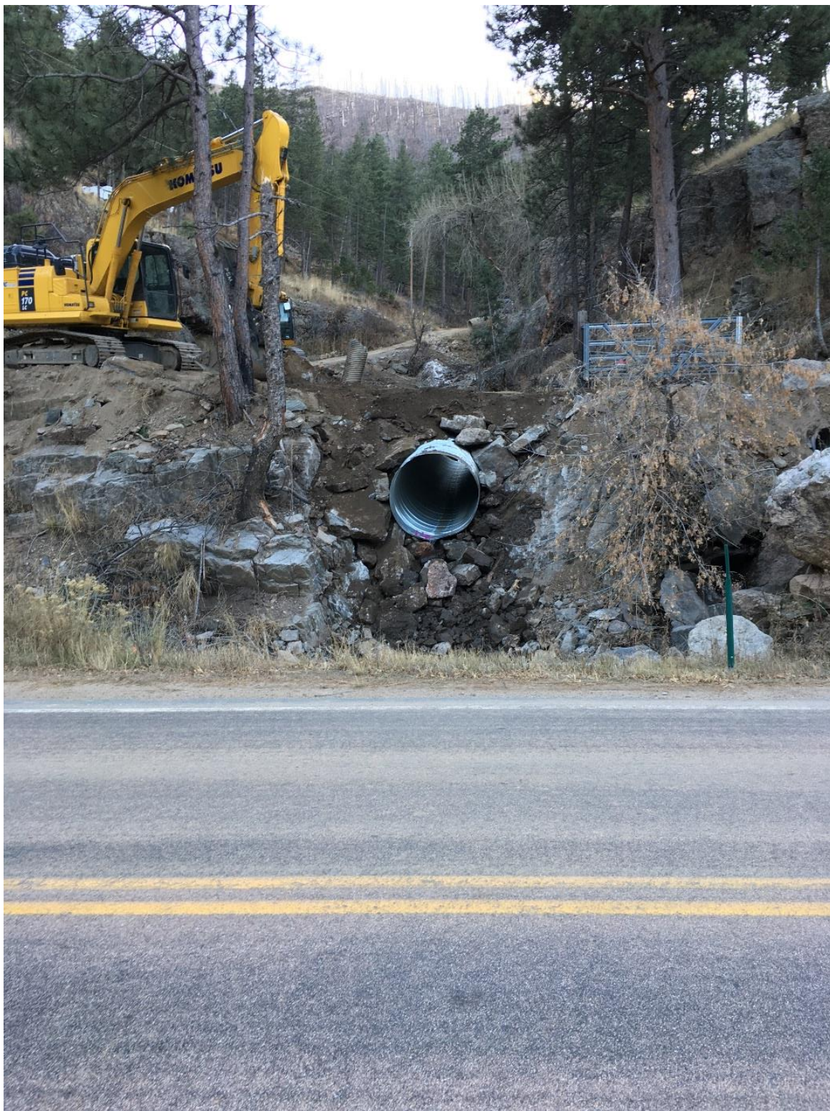
Photo 10. View Upstream Station 8+00 Culvert install
