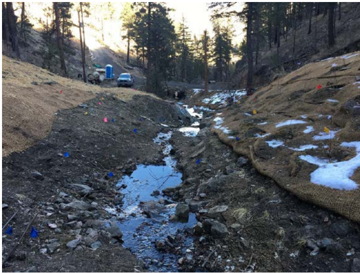
Photo 6. rock crossvane was installed to reduce the risk of head cutting upstream, and to stabilize the stream bankfull channel, floodplain re connected to stream.
