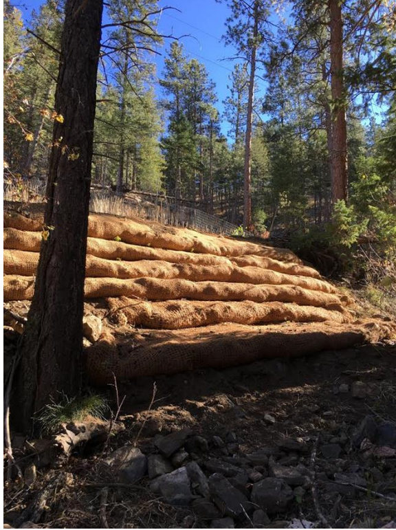
Photo 5. View Upstream Station 4+00 Vegetated Soil lifts
