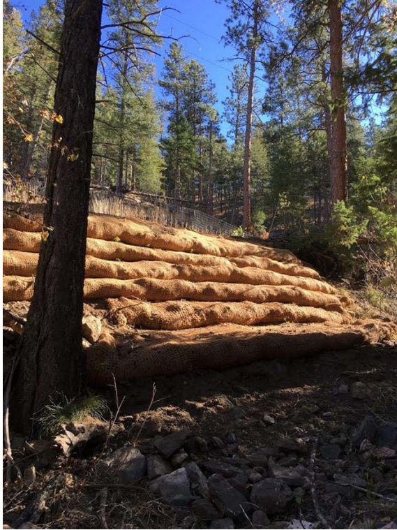
Photo 8. Vegetated Soil lifts installed to address bank hazard in two areas along the road embankment, where sparse vegetation, steep slopes, and poor soil dominated
