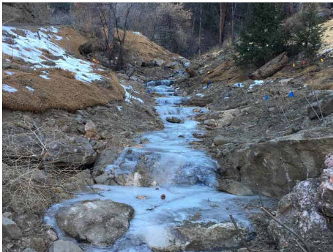
Photo 7. Rock cross vanes and a rock sill were installed to complete the grade drop to the elevation of the downstream culverts
