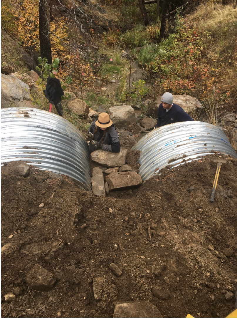
10/12 Constructed cross vane at station 2+20 below culverts. Completed retaining walls on downstream side of culvert at 2+00
