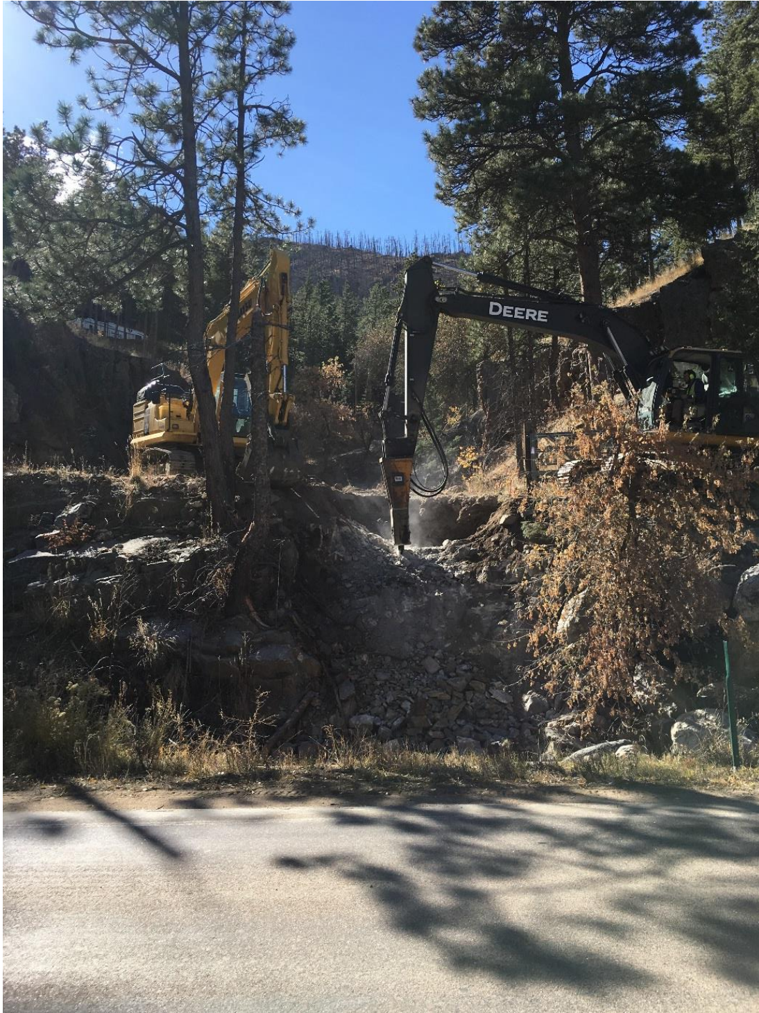
Photo 9. View Upstream Station 8+00 Jack hammering
