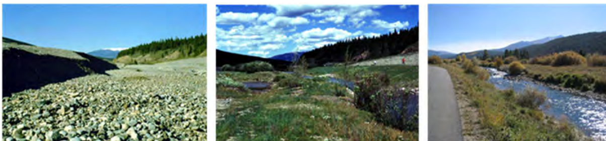
Figure 7. Blue River north of Breckenridge: left photo is before restoration, middle photo of overbank wetlands pond after restoration; right photo is river channel after restoration.
