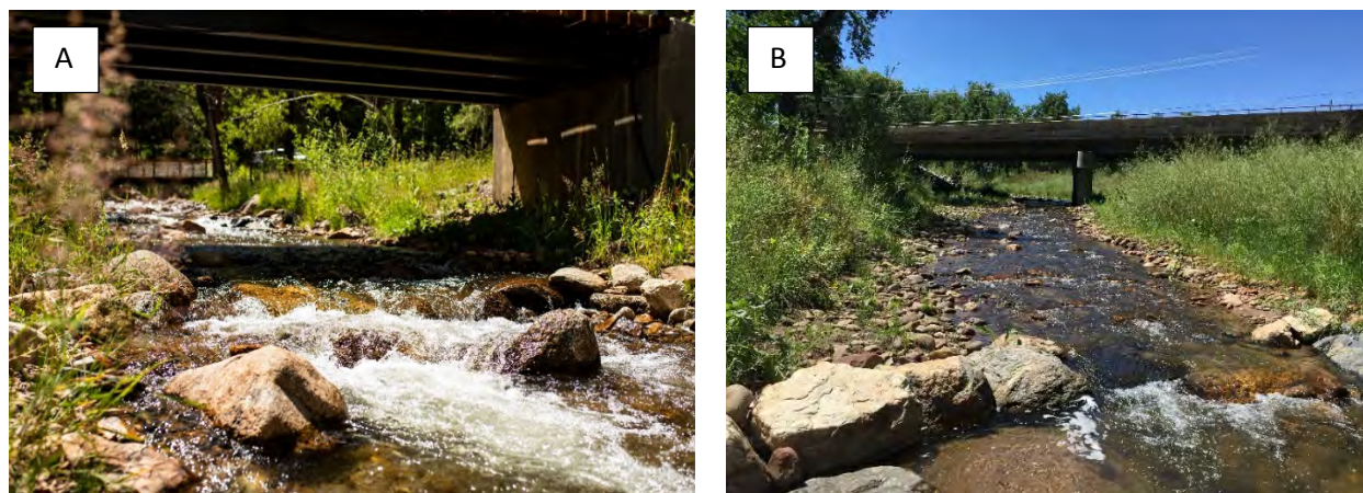
Figure 8. Pool forming cross sections at restored sites on Left Hand Creek. Photo description matches letter. A. boulder cross vane with immediate downstream pool at Upper Left Hand site in Left Hand Creek Watershed. Photo courtesy of OTAK, September 2019. B. constructed riffle at 63 rd Street site in Left Hand Creek Watershed. Fine sedimentation visible immediately downstream of structure. Photo taken 8-28-2019.
