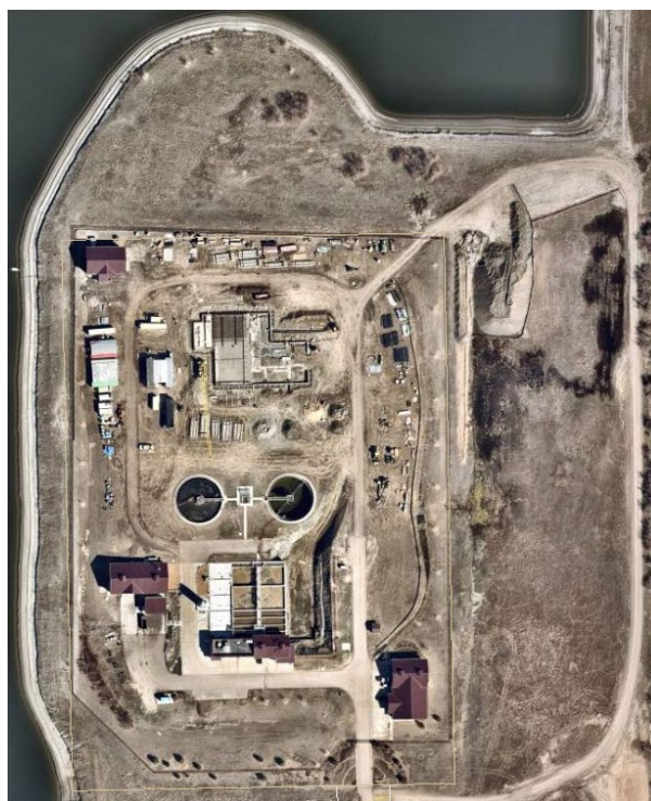
Erie's Wastewater Reclamation Facility
