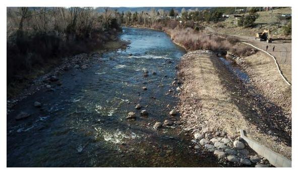
Figure 4 - Engineered riffle, looking downstream. Taken April 6, 2021 (~250 cfs)
