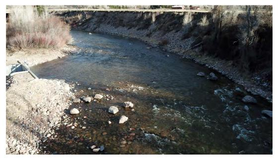
Figure 3 - Upper grade control as constructed, looking upstream. Taken on April 6, 2021 (~250 cfs)
