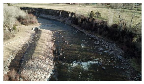
Figure 5 - Engineered riffle, looking upstream. Taken April 6, 2021 (~250 cfs)
