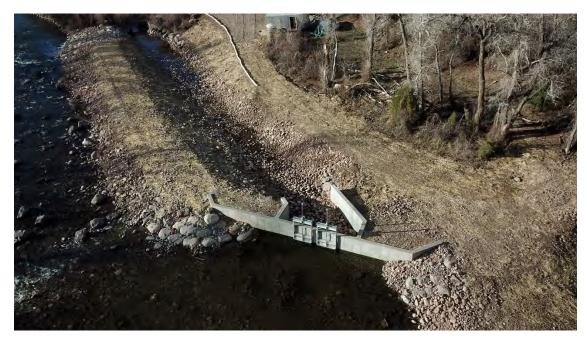
Figure 7 - New Robinson Diversion headgate and improved inlet ditch - Taken on April 6, 2021
