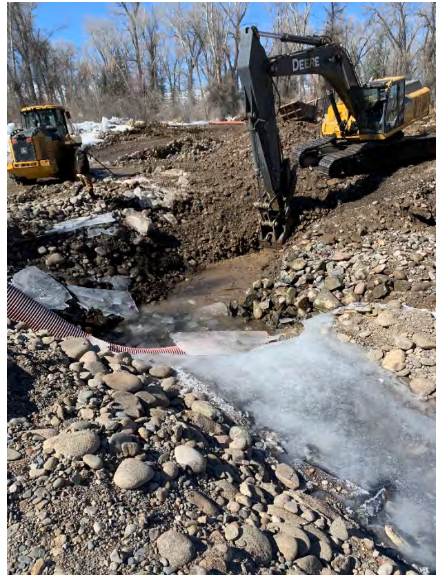
De-watering and excavating foundations for jettie structures.
