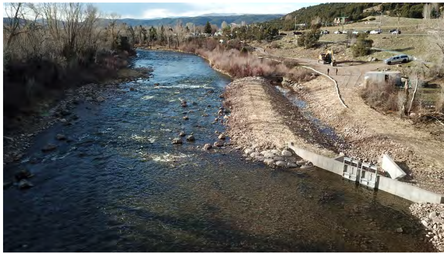
Figure 1 - Completed in-channel work in early April 2021. Grade controls and engineered riffle on river left and the headgate and ditch improvements on river right.
