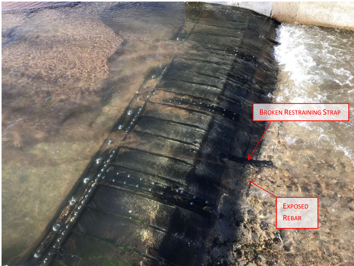
Fig. 3: Diversion bladder gate, note exposed rebar.
