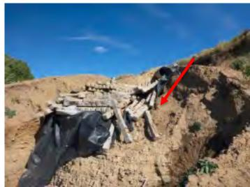
Bank erosion and concrete tie displacement
