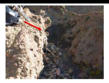
Hillside Seep Installed French Drain & Pipe
