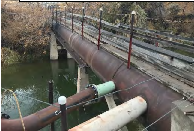
PIPELINE OVERSHOT 48" STEEL PIPE and Walkway from Pump Station #1 Prior to Construction
