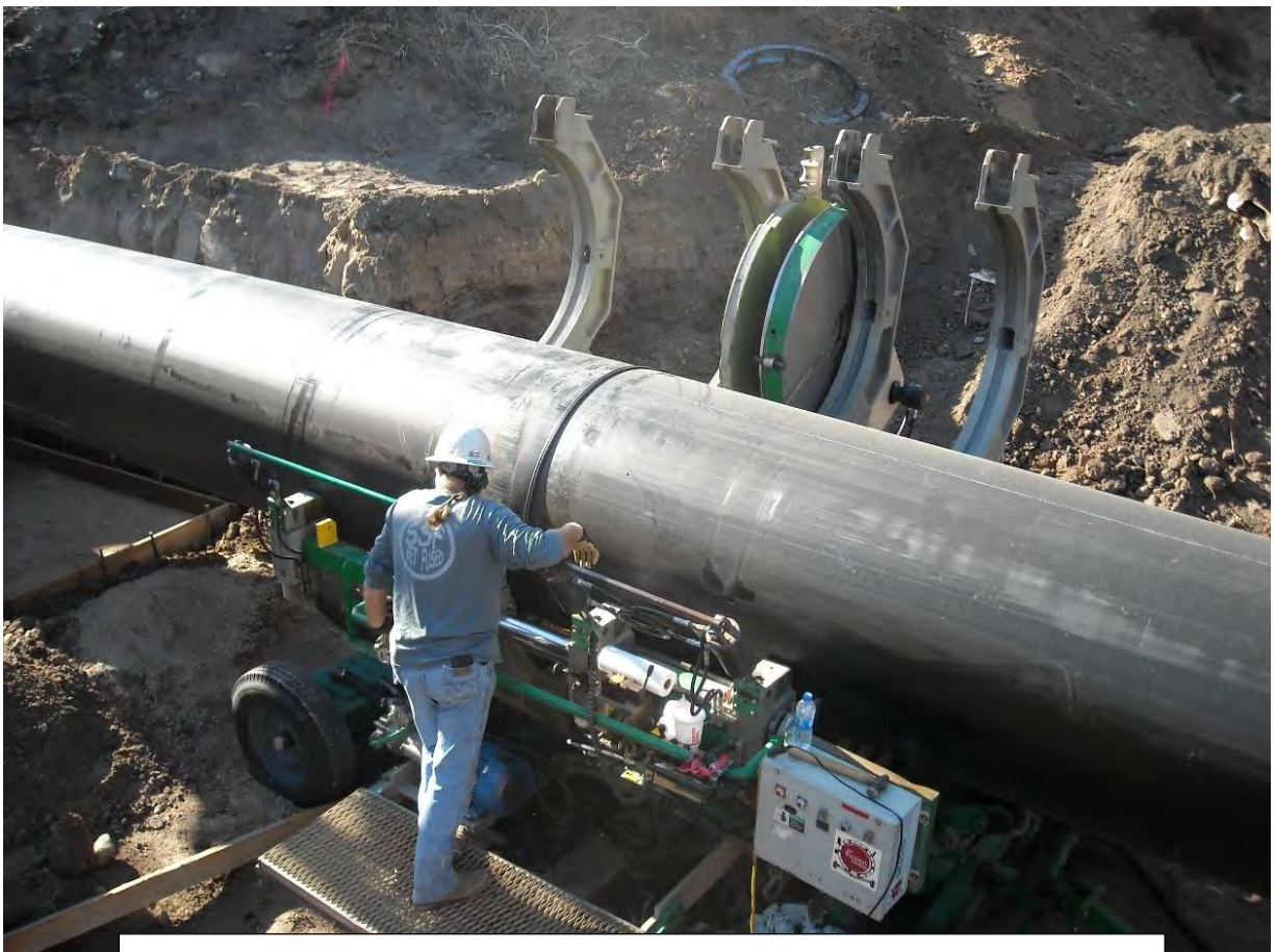
Welding of 48" HDPE pipe and 8" steel pipe for the drainpipe at the lower end of the overshoot. All welding was inspected by engineers or third-party inspectors required by contract, in addition to RW&PC inspections on site.
