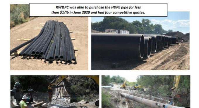
Removal and replacement of the 48" steel pipe overshot and upper section of buried pipe. Concrete plugs were installed to abandon buried pipe with drainpipe at lower end. New pre-cast concrete pier saddles and baring pads were installed under new overshot pipe.
