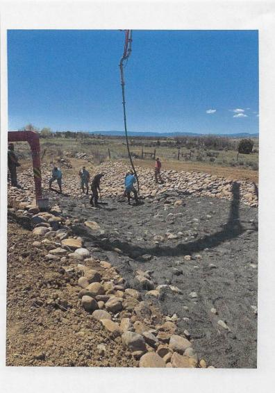
filling rock with pumpable grout
