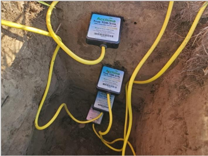
Figure 3: Installing Acclima soil moisture sensors
