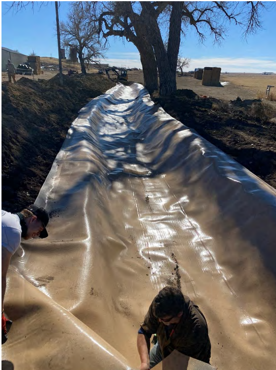
Attaching the Liner to Concrete
