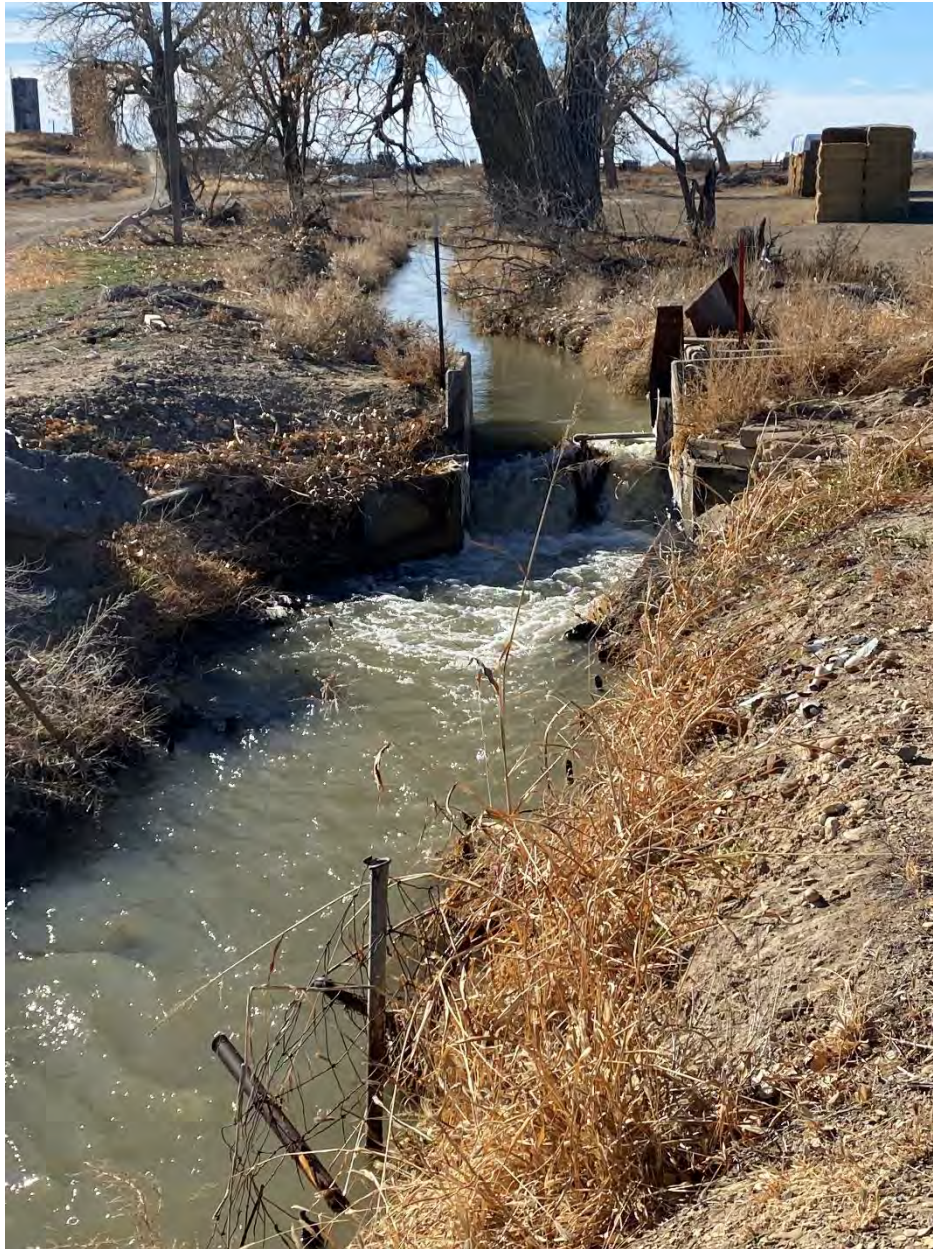
At the Divide Box where NRCS calculated 30% losses
