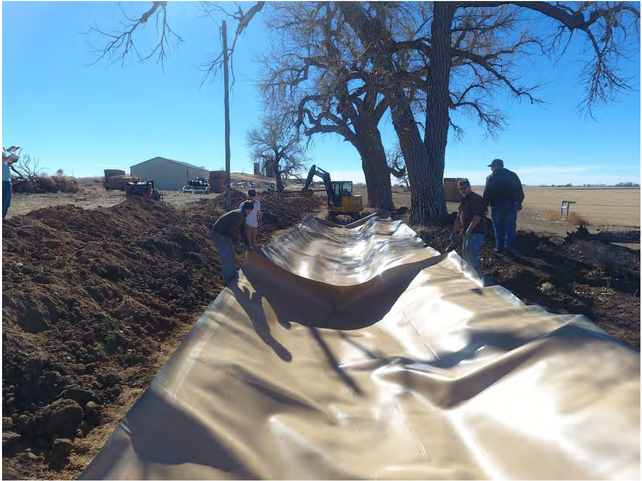
Setting the Liner for Spray and Sealants
