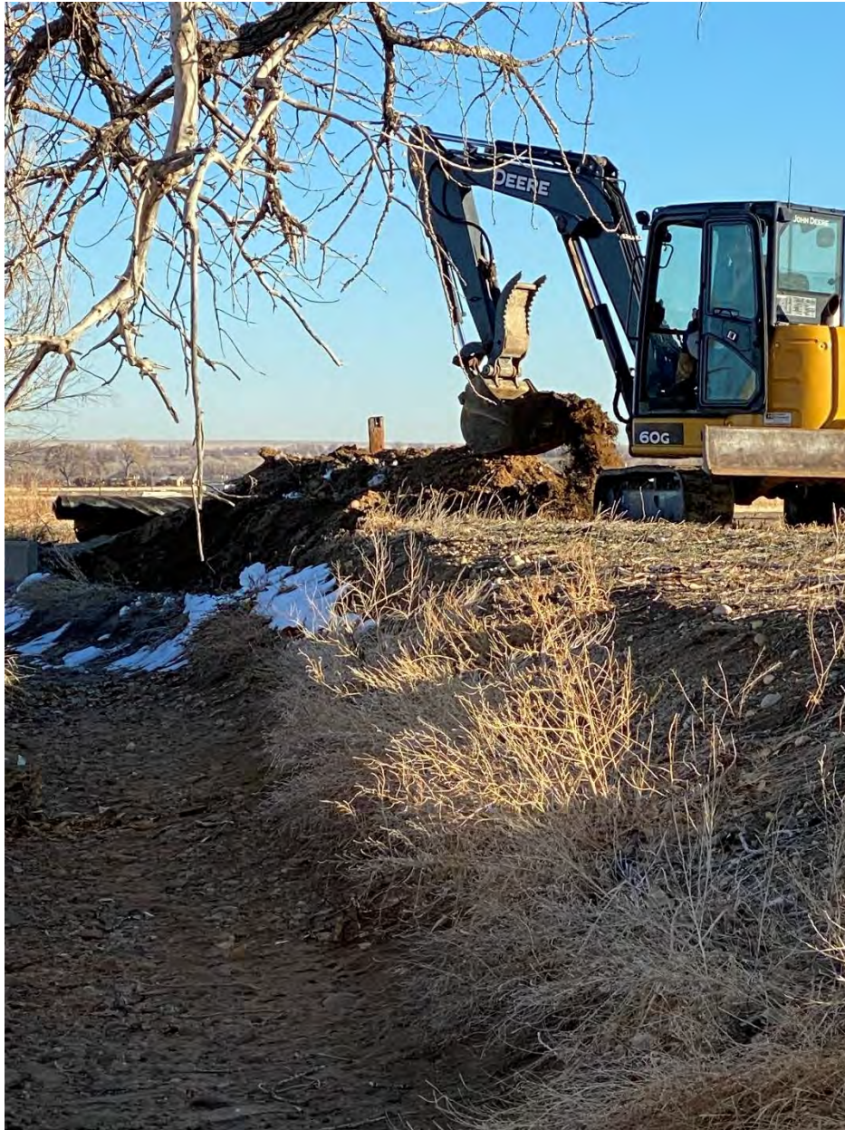
Preinstallation Trenching for the Keyway
