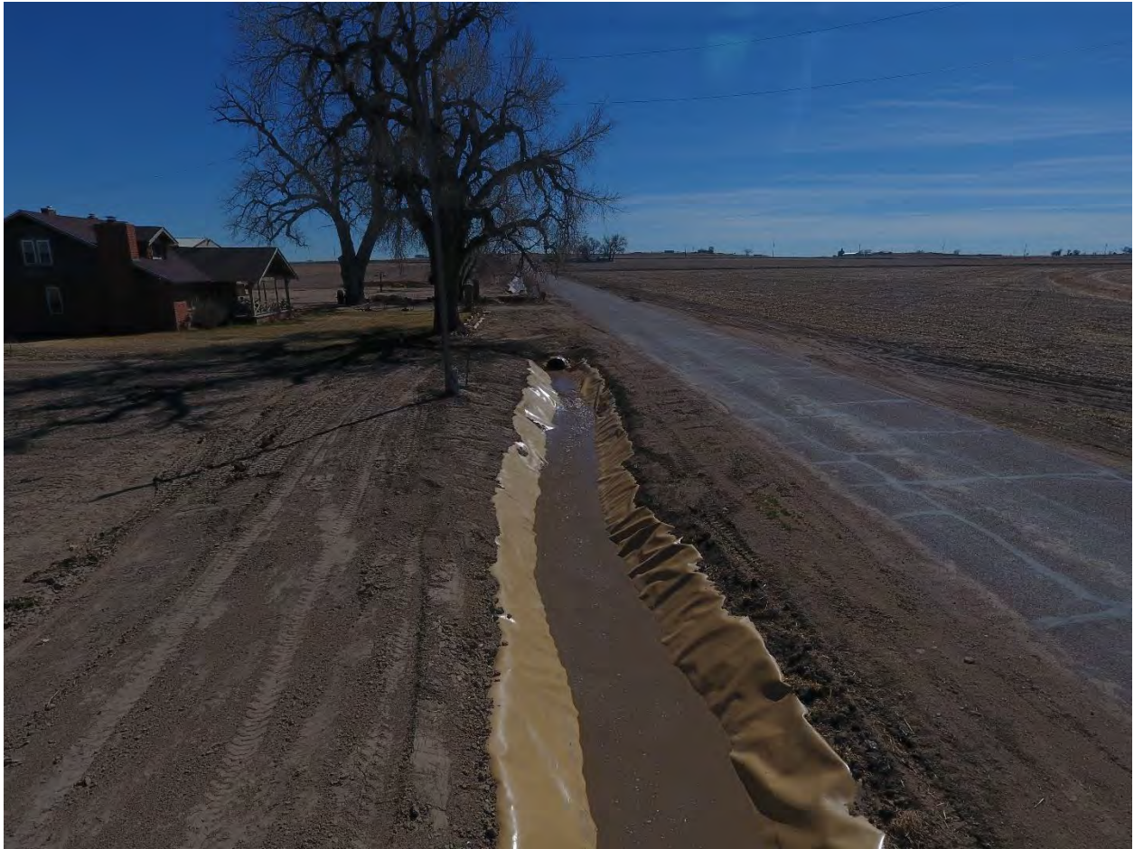
Installed Liner Carrying Water on March 17 th
