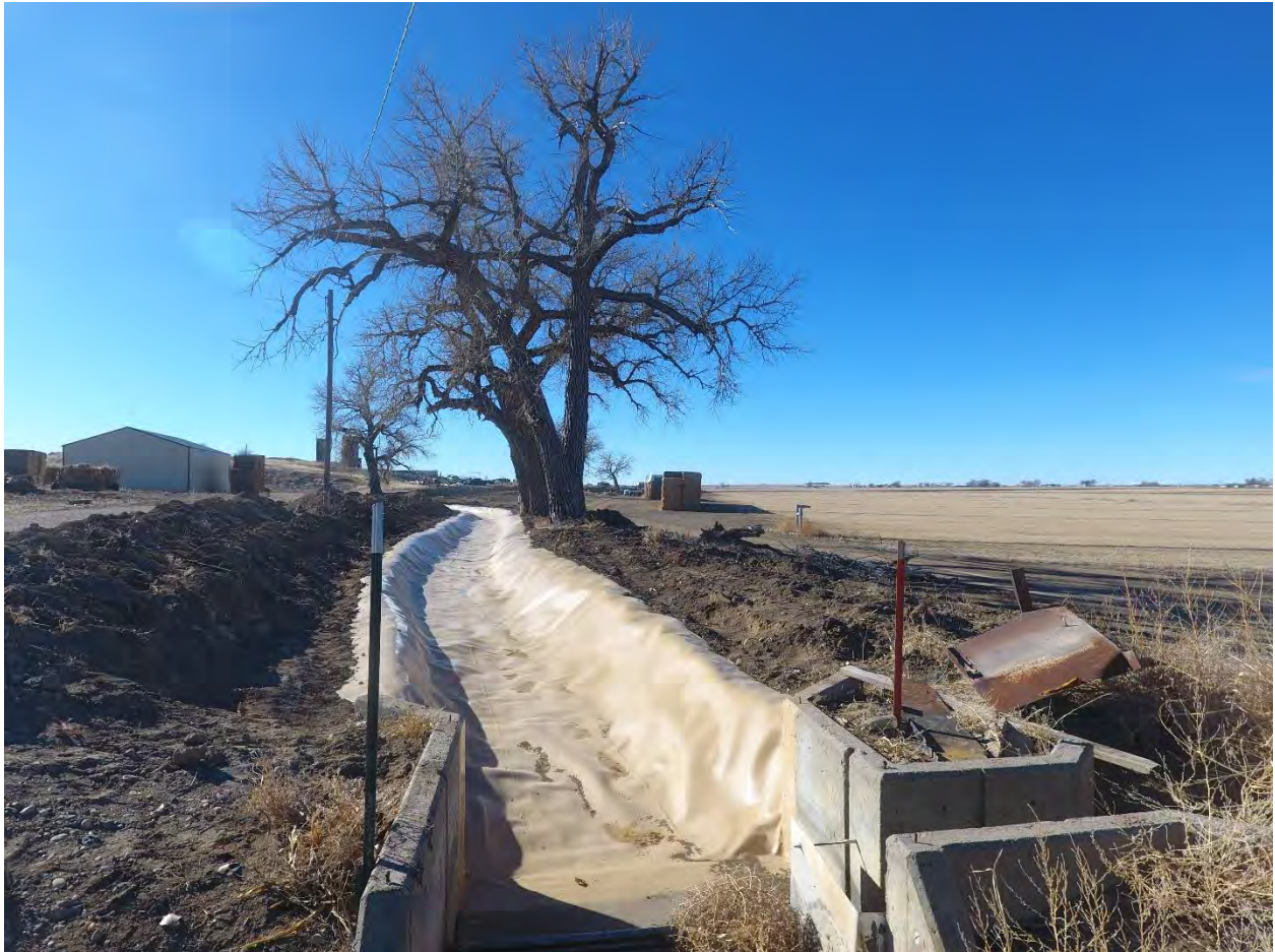
Installed Liner awaiting Backfill
