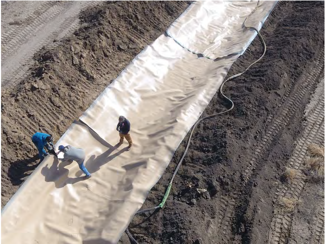
Cutting and Shaping the Liner
