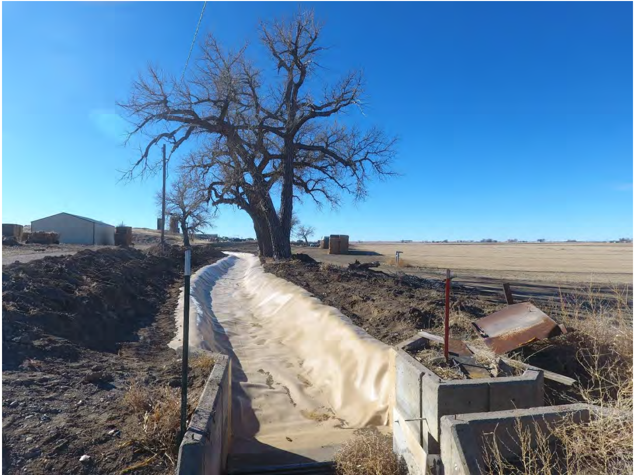
Installed Liner awaiting Backfill
