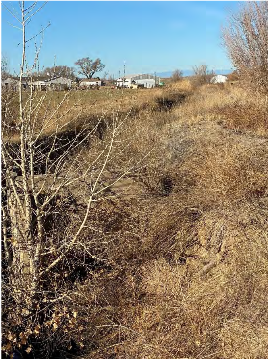
Erosion and Tree Growth at the Headgate
